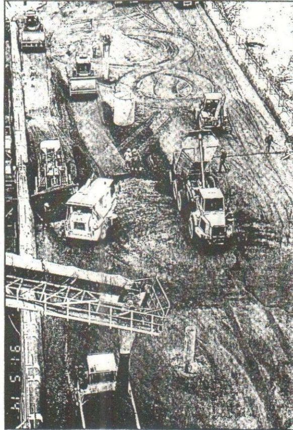
Figure 2: Typical RCC placement and compaction operation
