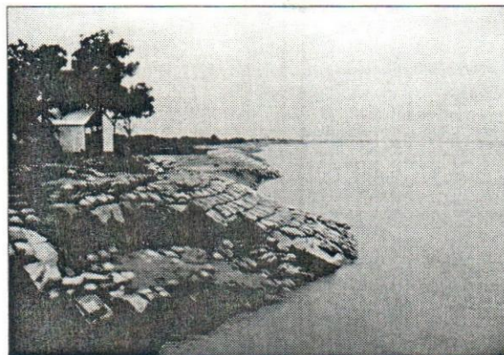
Figure 5: Geobag protected riverbank failure
