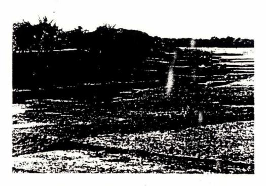
Retired BRE at Baishakhi showing line of borrow pits along riverside foot of embankment
