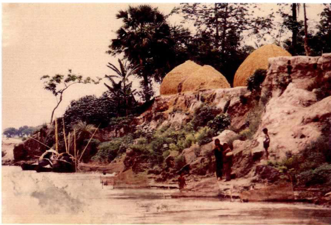
Plate 2 Main bank erosion on the left bank of the lower reach
