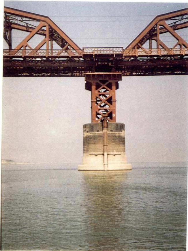
a. Bridge pier showing the BWDB float-well AWLR
