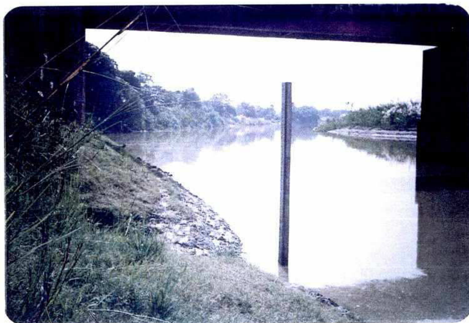
Gauge Station : L Bausi Railway Bridge
