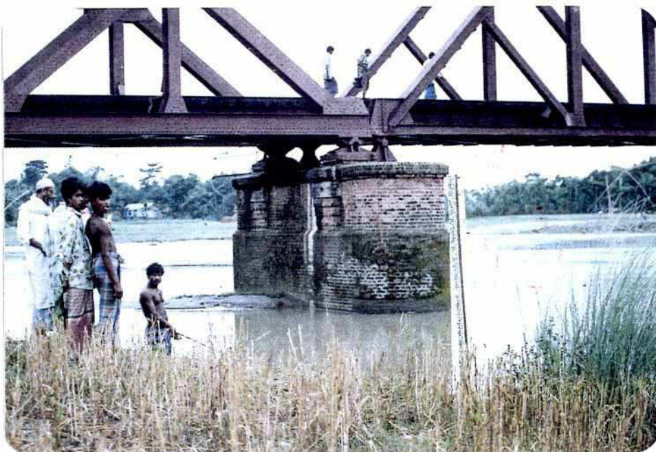
Gauge Station : M Jhenai Railway Bridge
