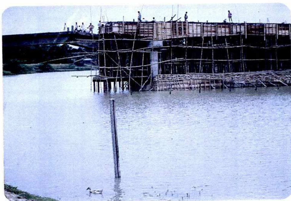
Gauge Station : 06 Poyla Bridge
