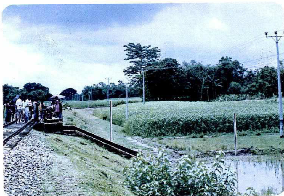
Gauge Station : C Putdanga Railway Bridge
