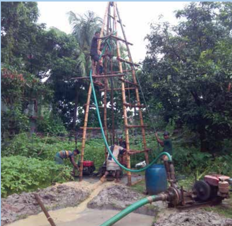
Figure: Exploratory drilling and collection of sediment samples in the project area
