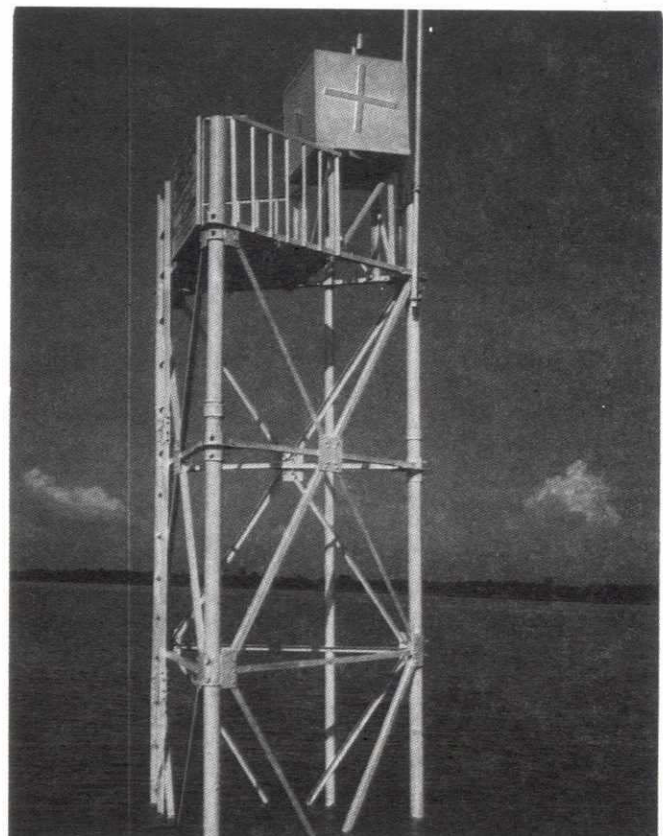
Figure 5.2: An ALWR (Automatic Water Level Recording) platform
