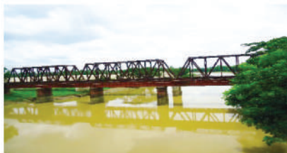
Railway Bridge on Muhuri River
