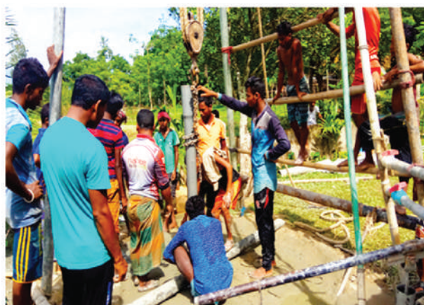
Installation of Tubewell as a Water Supply Option.
