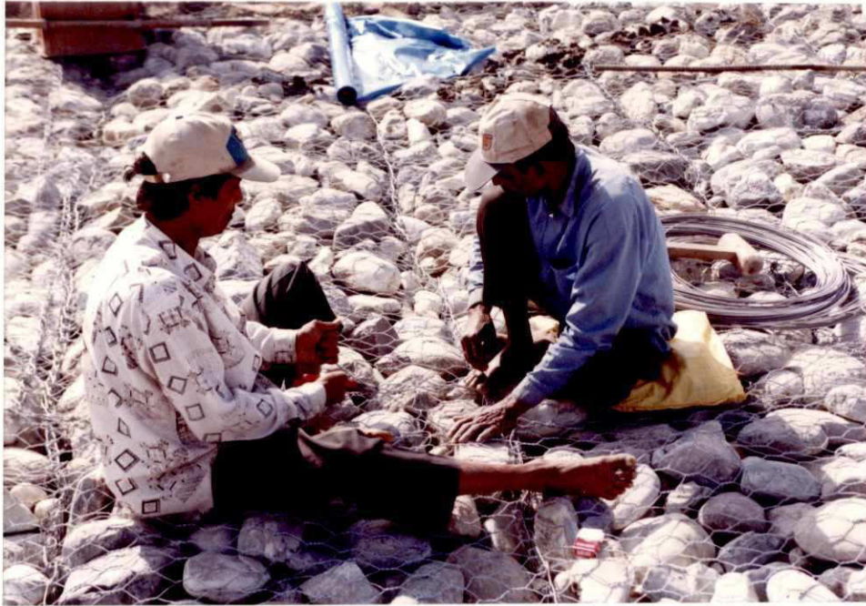
Photo 7: Test Site III – Ghutail; Launching Apron: closing of Reno-mattress
