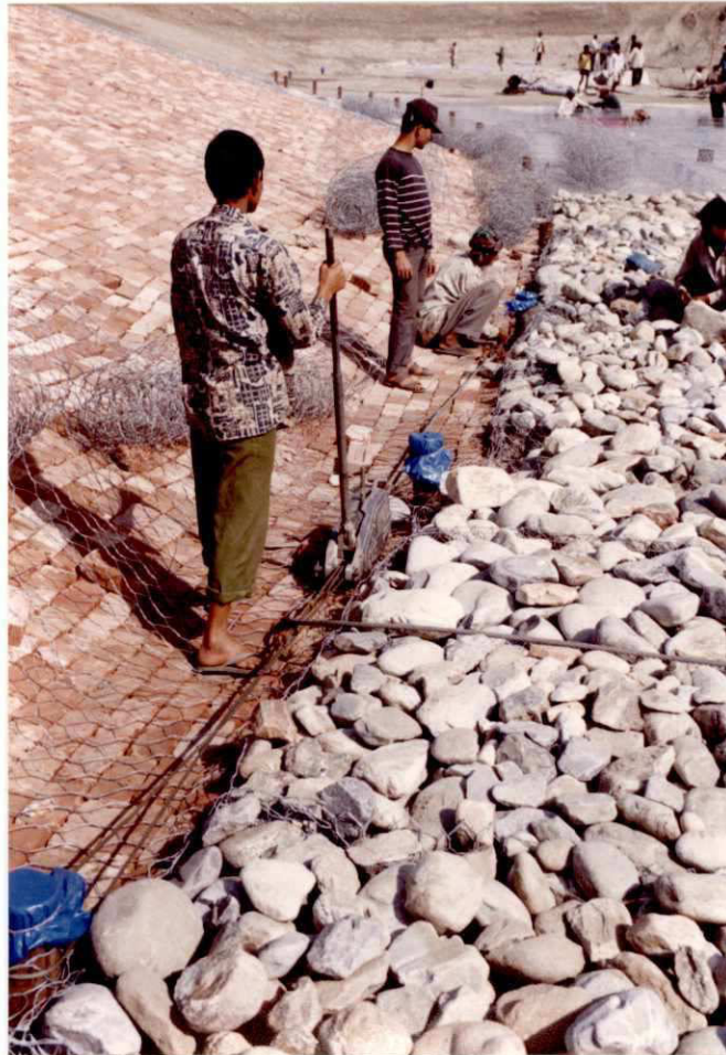
Photo 8: Test Site III – Ghutail; Launching Apron: “pre-stressing” of anchor cables
