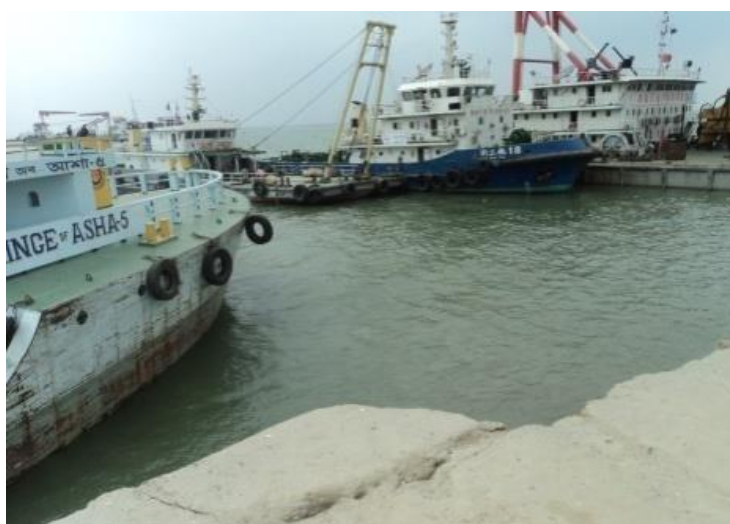
Figure 2.3: Bank erosion of Padma river (at Mawa site, Padma Multipurpose Bridge Project Area)
