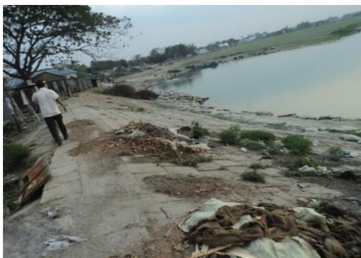
Figure 2.2: Bank caving of Padma river (at Hajiganj bazar, Charbhadrason upazila, Faridpur)
