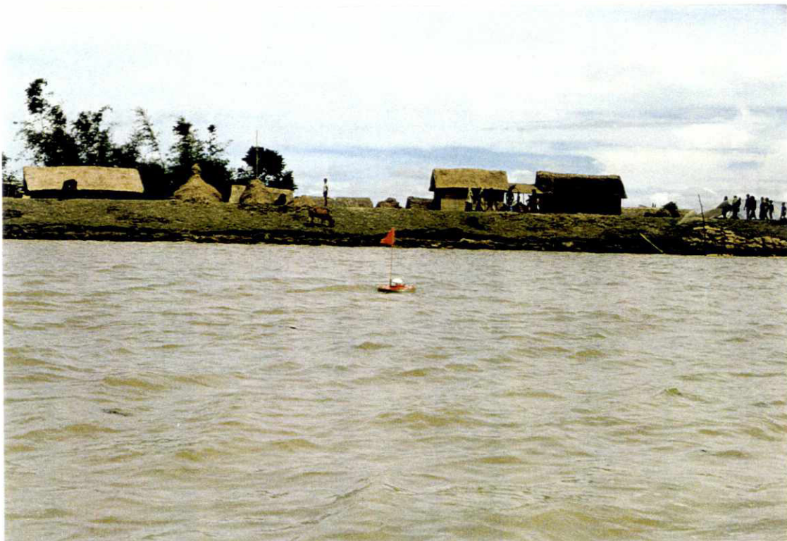
Fig. 15: Photo from the 02/08/96 of Wave Erosion on the Embankment after the Storm on the 26/07/96
