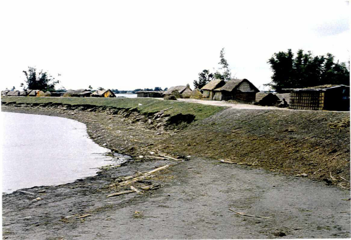
Fig. 16: Photo taken on the 12/08/96 showing the Damage to the unprotected Embankment
