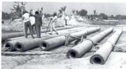
Prestressed spun concrete piles joined at site (2 sections @ 10 m, total length 20 m)
