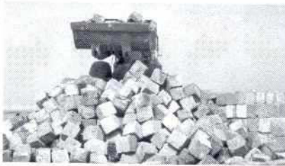
Dumping of CC-blocks within the designated falling apron area of a structure
