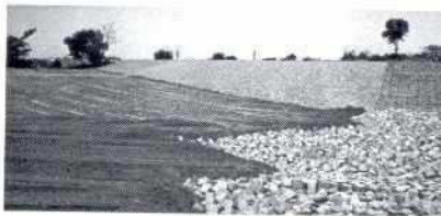
Covering of the completed launching and falling aprons as a protective measure against human intervention
