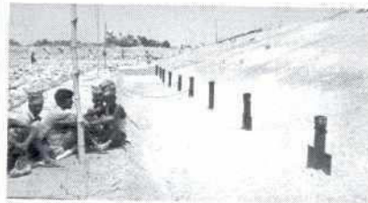
Installation stage of deadmen along toe of upper embankment (berm level)
