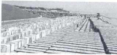
Casting of CC-blocks directly in-situ at the designated falling apron area of a structure.
