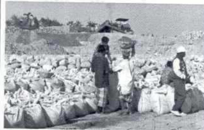
Filling of geo-sand containers at site (directly at the designated location within the structure)
