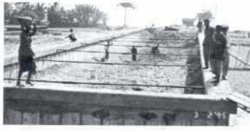
Cofferdam: backfilling and compaction
