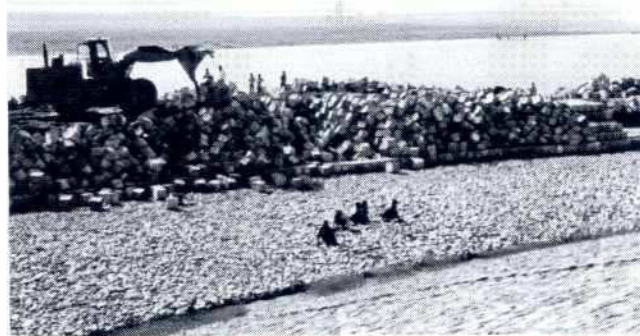
Fig. 5.3-4: Random placed CC-blocks (falling apron)
