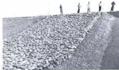
Figure 7.3-3: Placing of multi-layer granular filter and rip-rap cover layer
