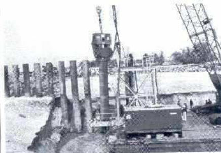
Pile dia. 711 mm during installation stage by vibrator hammer
