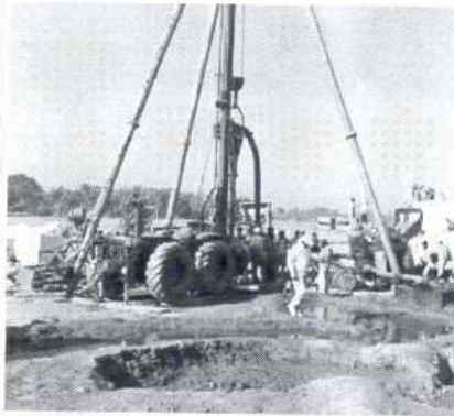
Drilling for in-situ cast reinforced concrete piles by reverse rotary method
