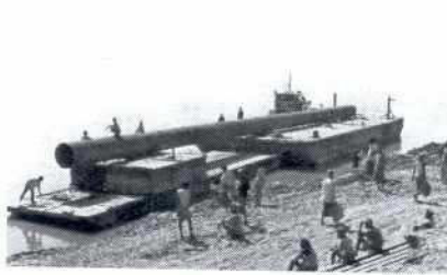
Pile loading shore-to-pontoon
