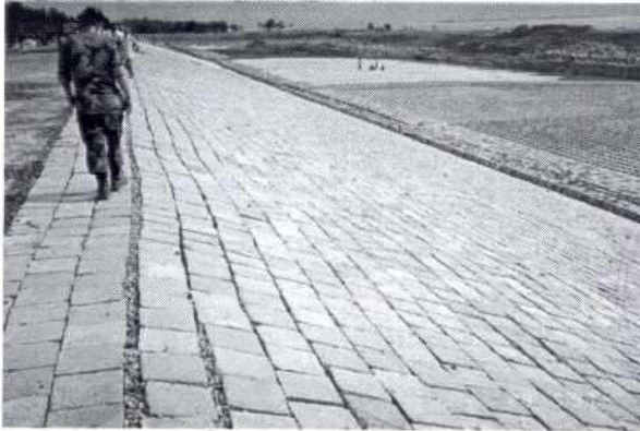
Fig. 5.3-3: CC-blocks used as revetment cover layer
