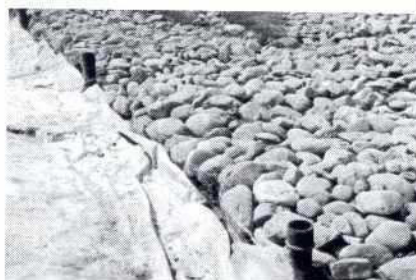
Figure B: Anchor trench partly filled
