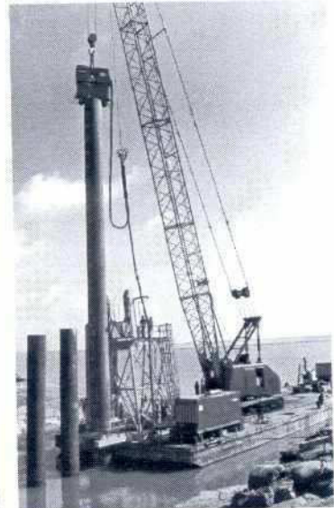
Start of pile installation by vibrator (here: transition zone near bankline)
