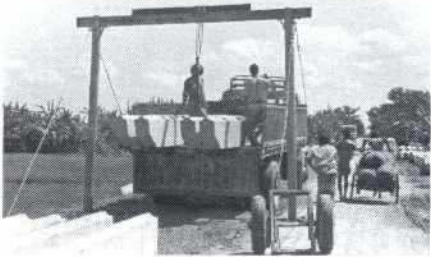
Unloading of RCC-sheet piles for transshipment
