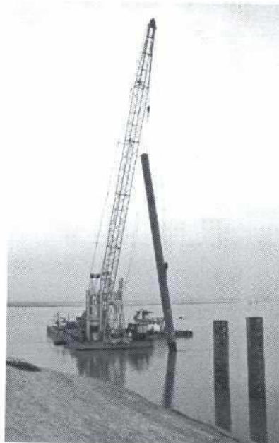
Final stage of pile lifting
