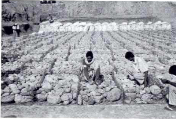
Fig. 5.3-5: Filling of wire mesh mattresses with boulders (launching apron)
