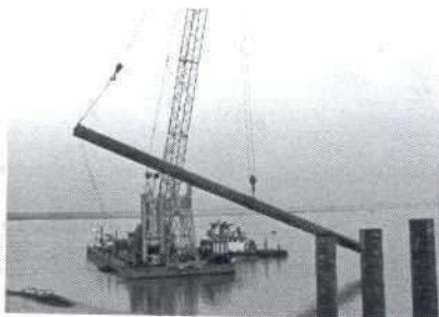
Second stage of pile lifting (transport pontoon towed away)
