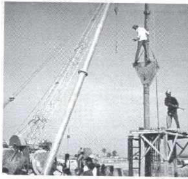
Concreting of pile by tremie pipe method
