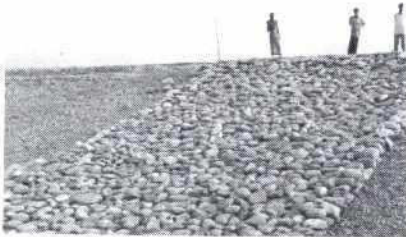
Revetment of rip-rap placed on a granular filter
