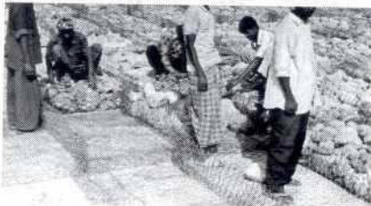
Initial stone filling of RENO®-mattresses (prior to installing steel wire cables)
