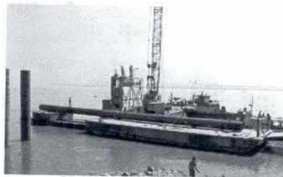
Pile transport to place of installation
