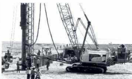
Final driving stage with RB-driving rig and hydraulic BSP-hammer 357-7
