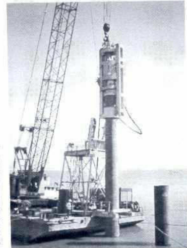
Final pile installation stage by hydraulic hammer MENCK MHF 10-15
