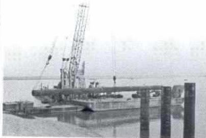
Lifting of pile (initial stage)
