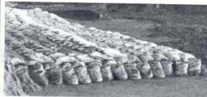
In-situ filling and placing of geo-sand containers within the designated area
