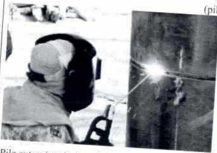
Pile extension during pile installation process
