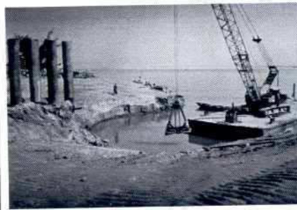
Clamshell dredging for pile installation at the bank-line transition shore-to-riverside
