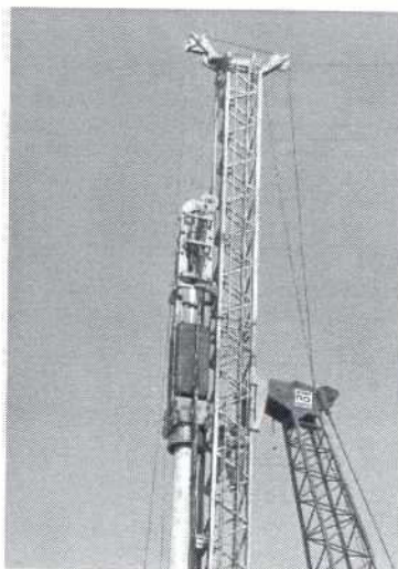
Initial driving stage with RB-driving rig and hydraulic BSP-hammer 357-7
