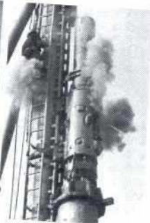
Pile hammer Kobe 22 with pile cap (pile dia. 711 mm)
