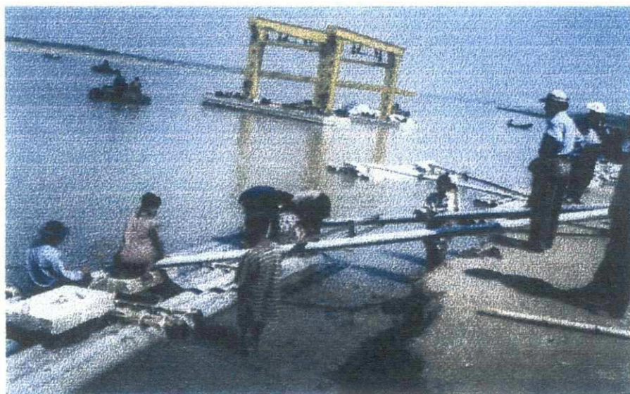
Picture 4 Transport of foundation slabs and A-frames to the THP
