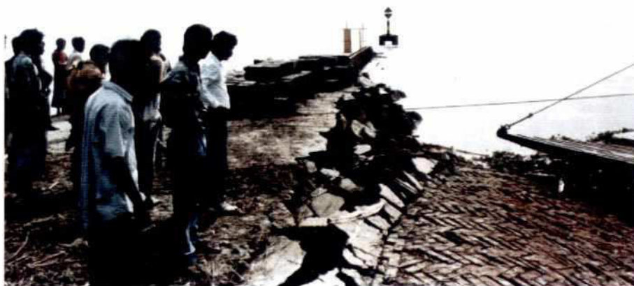
Photo 6.8-2: Development of a crack in groyne G-3, August 1995
