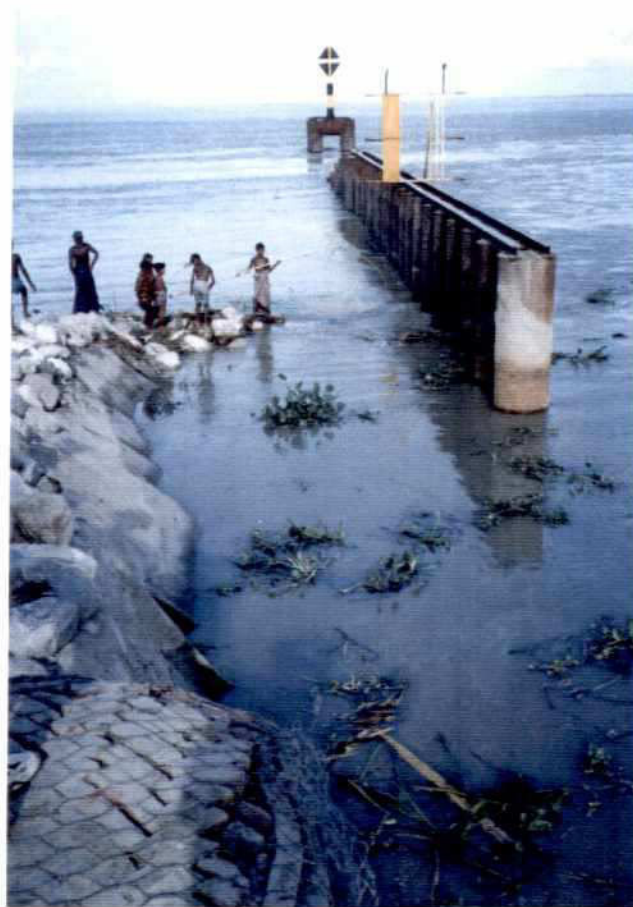
Photo 6.8-7: Transition between permeable pile row and earth dam after slide at groyne G-3, August 1995
