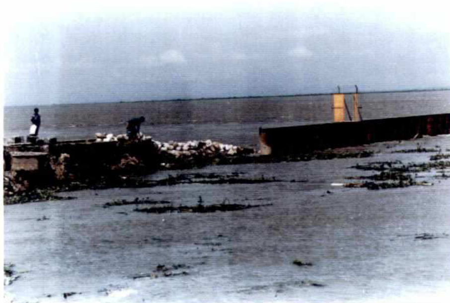
Photo 6.8-6: Transition between permeable pile row and earth dam after slide at groyne G-3, August 1995
