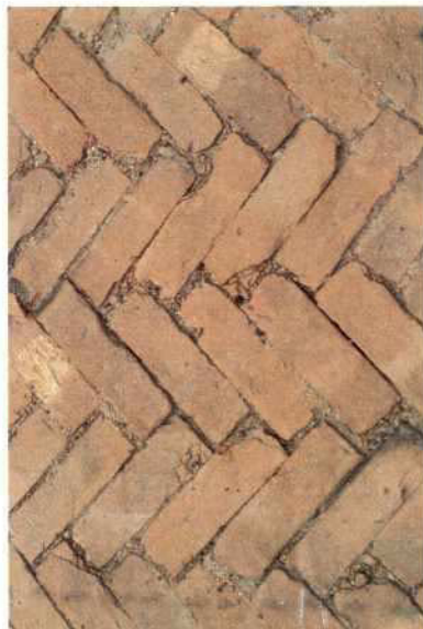
Rural feeder road: herring-bone brickwork
