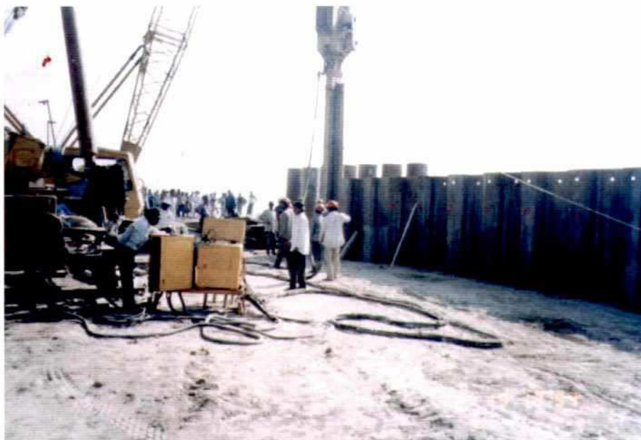
Photo 3.5-7: Steel sheet pile installation at groyne G-1 with electric vibrator
