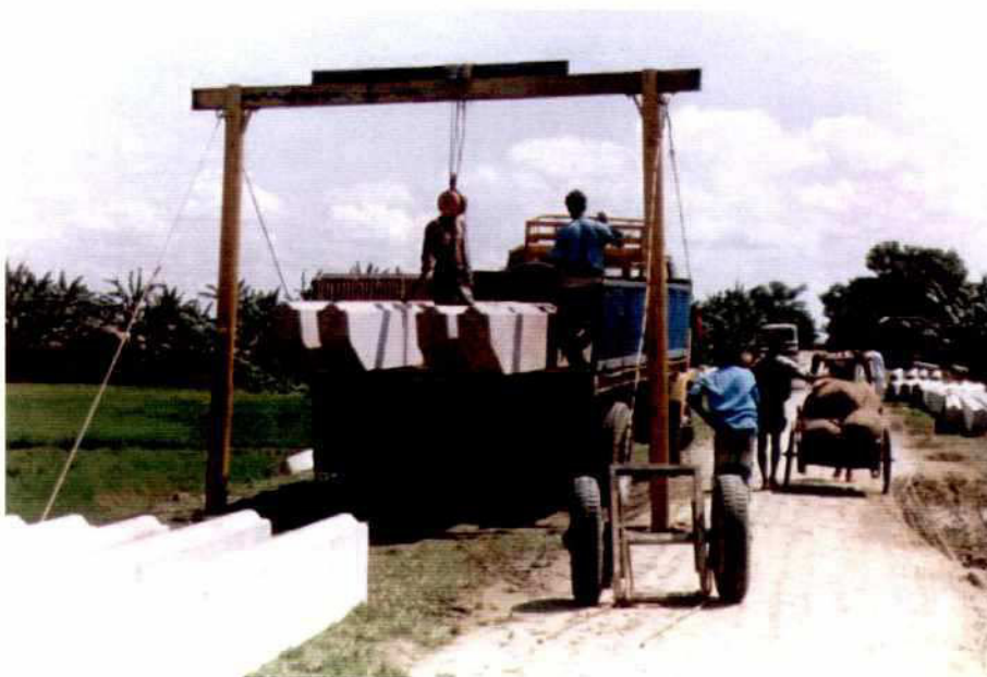
Photo 3.4-3: Pre-cast reinforced sheet piles
