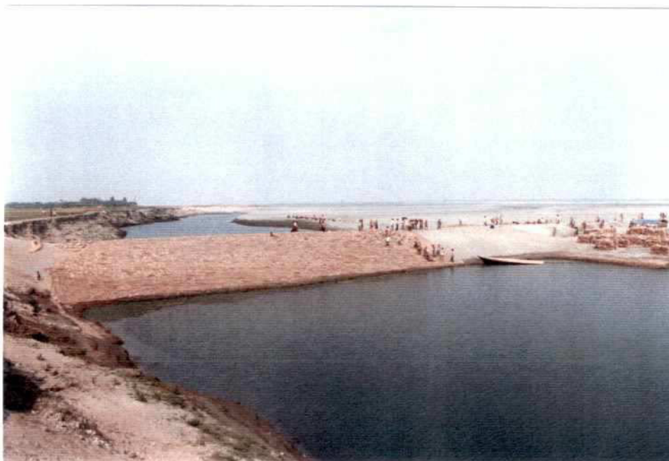
Photo 4.2-2: Earth dam closing Katlamari channel during the final stage of construction in March 1997, in the background the bandal structure
