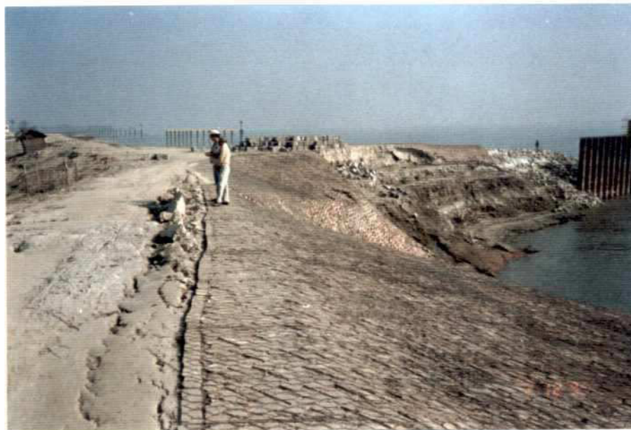
Photo 3.7-3: Downstream face of eroded impermeable section of groyne G-3
