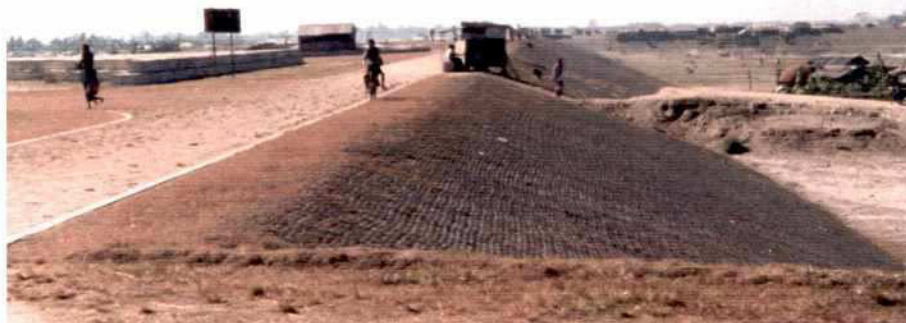
Photo 8.2-2: Earthdam with brick mattresses at "hard point" No. 3. The main embankment can be seen in the background (situation in December 1999)
