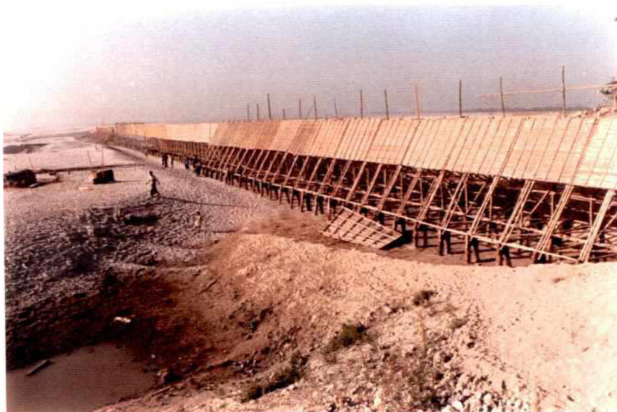
Photo 4.2-1: Improved bandal structure after construction at Katlamari in March 1997
