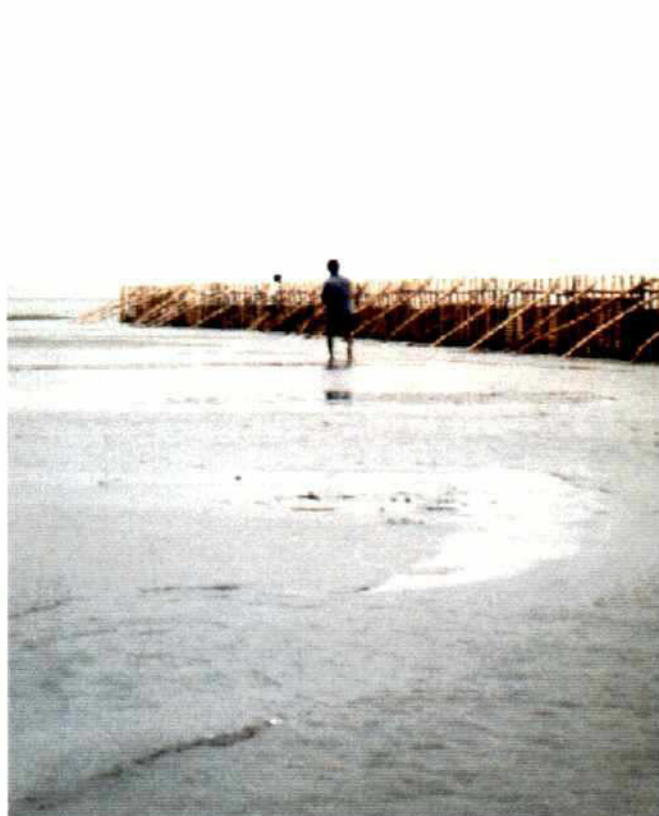
Photo 4.3-4: Sedimentation behind the low water bandals
