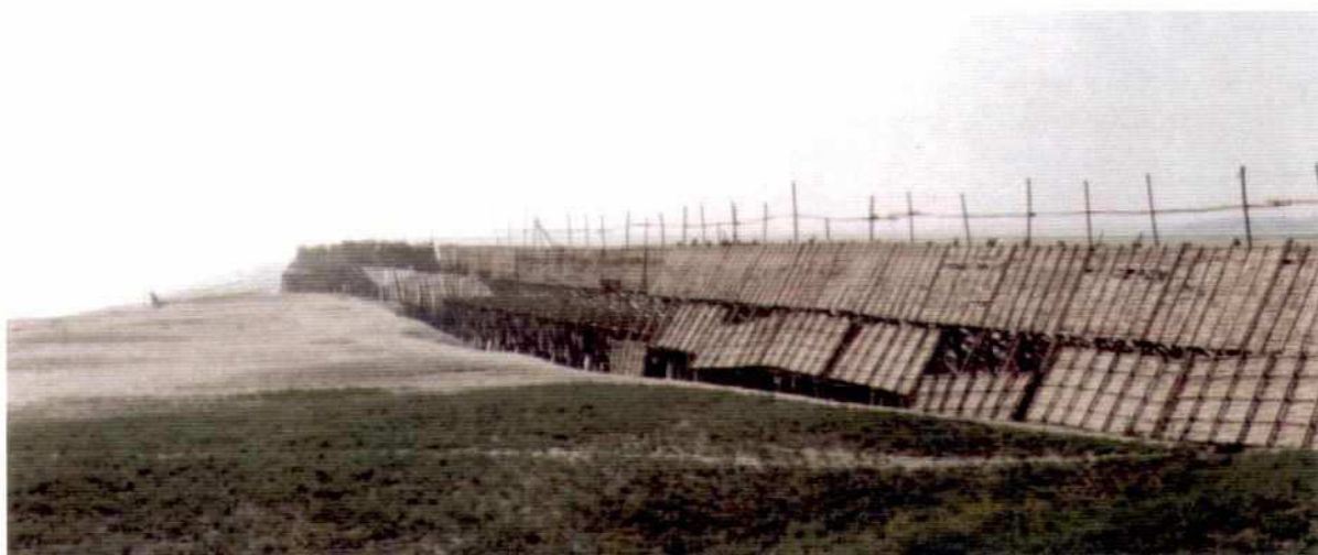
Photo 4.2-7: Bandal structure after the monsoon flood in January 1998
