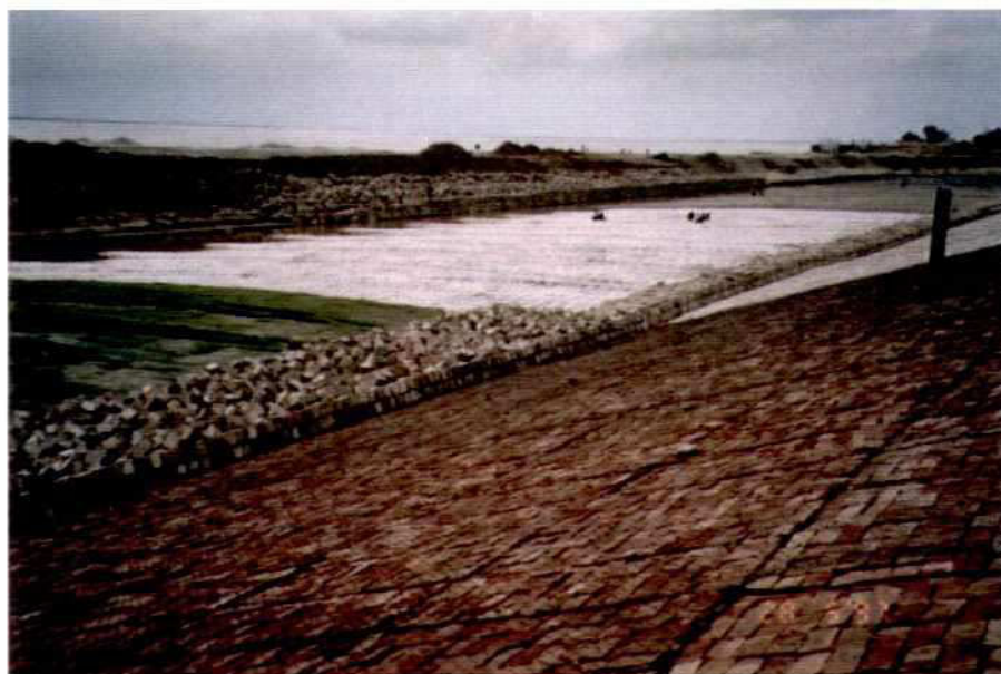
Photo 4.4-2: Slope protection by brick mattresses (test Section F, view to the north)
