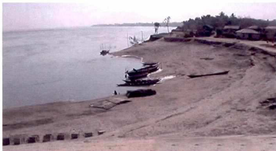
Photo 8.2-3: Erosion downstream from "hard point" No. 3 at Mathurapara (situation in December 1999)
