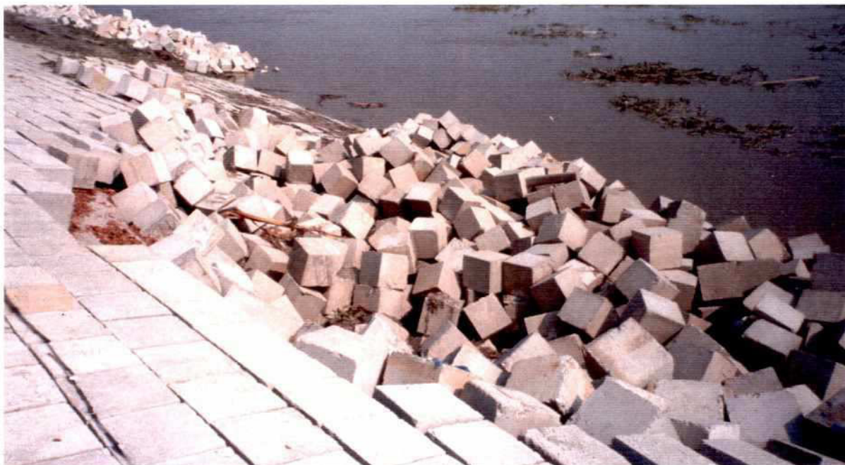
Photo 8.2-1: Damaged revetment at Sirajganj with dumped concrete blocks (situation in October 1998)
