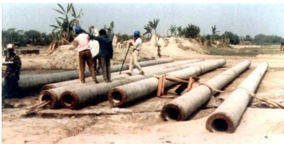
Photo 3.4-2: Pre-stressed spun concrete piles with purpose made joint
