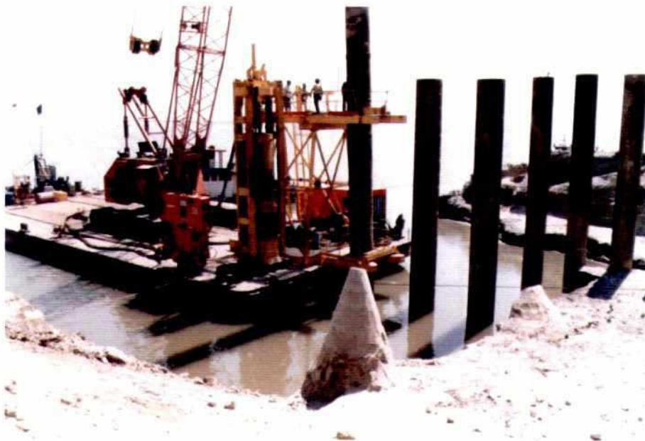
Photo 3.5-5: Off-shore installation of steel pile
