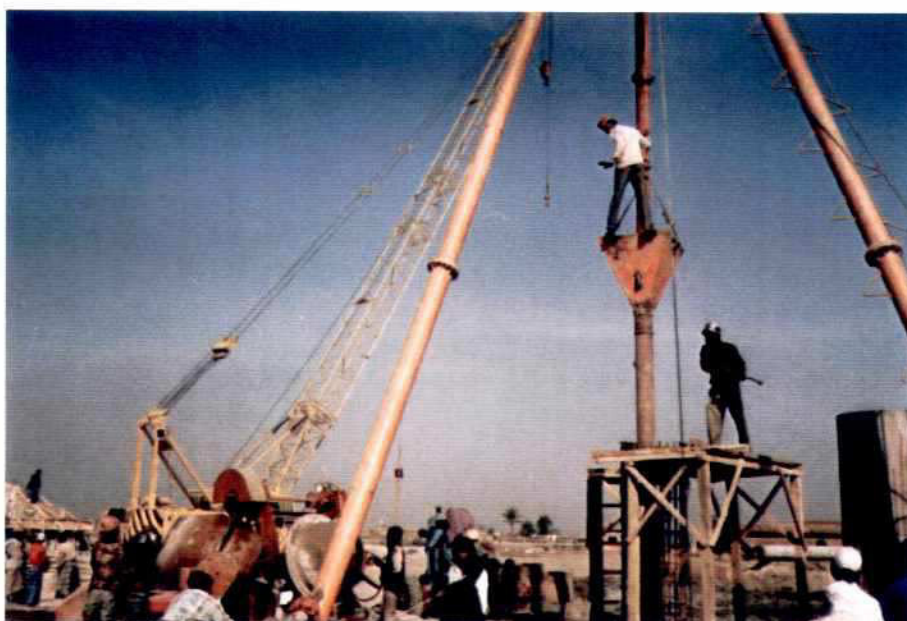
Photo 3.5-6: Concreting of in-situ bored piles
