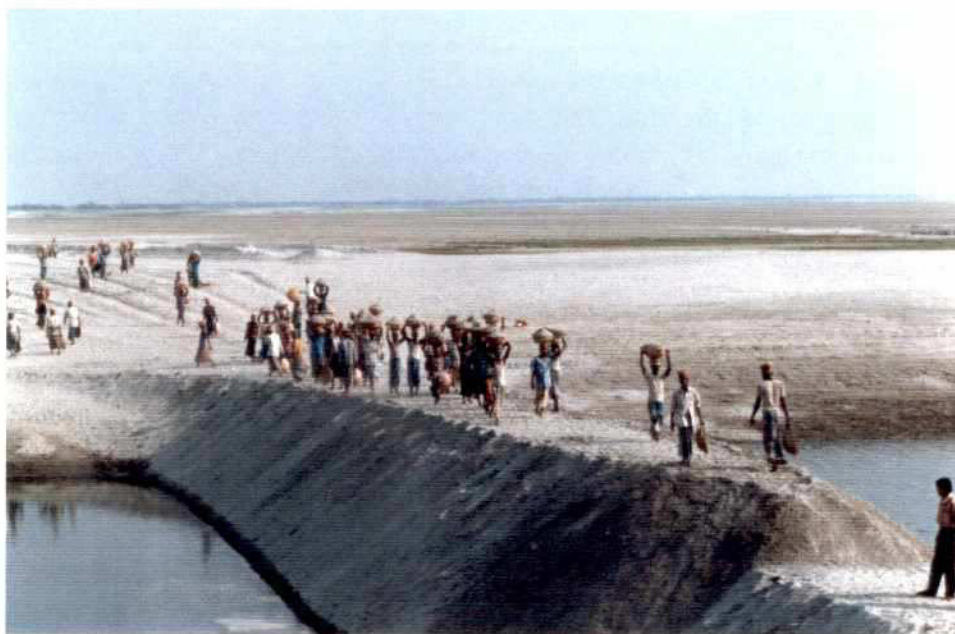
Photo 4.2-4: Construction of earth dam in February 1997
