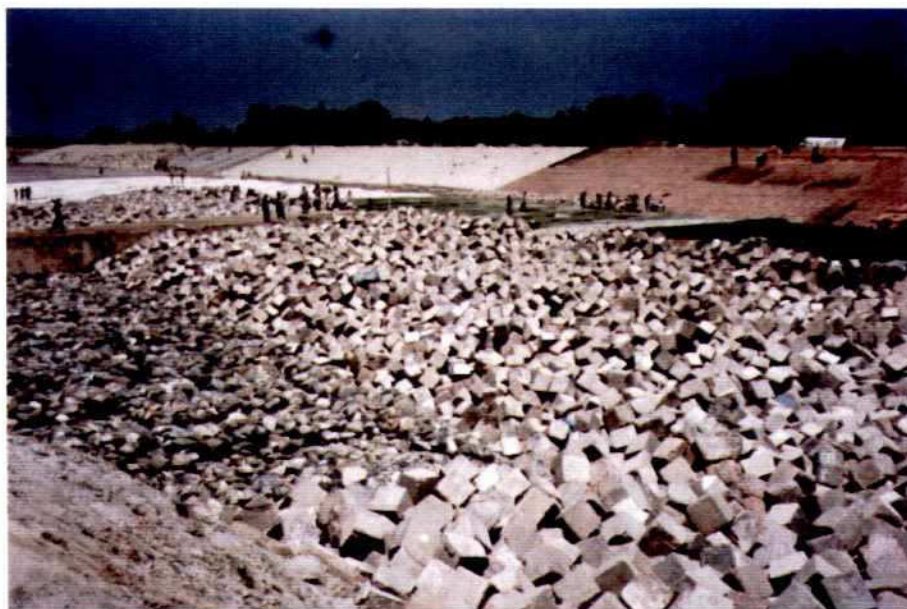
Photo 4.4-6: CC-blocks and gabion sacks (to the left) used as falling aprons
