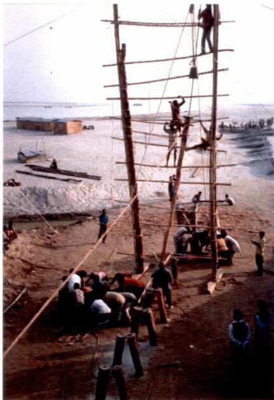
Photo 4.2-3: Pile driving for the foundation of the bandals in January 1997
