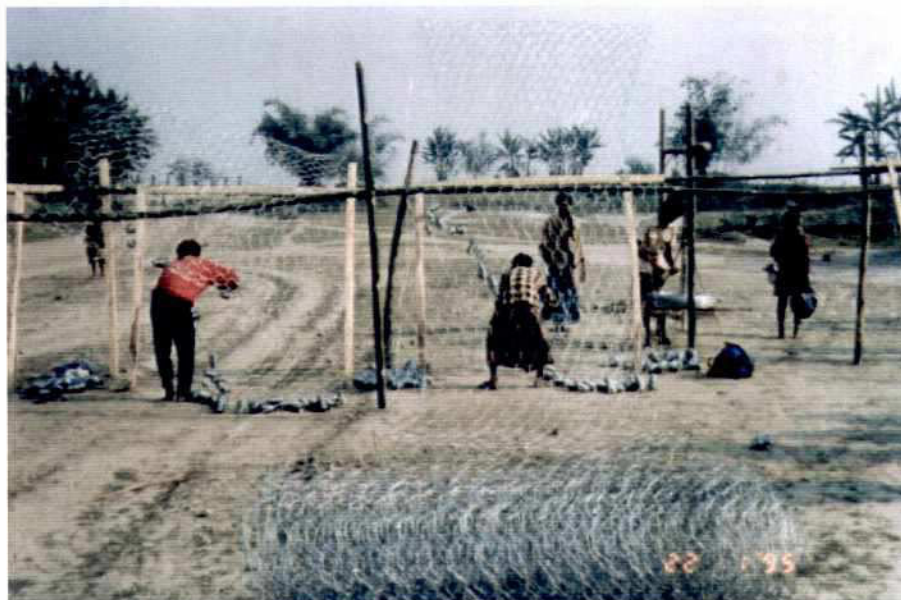
Photo 3.4-1: Production of wiremesh at site
