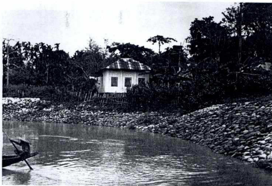
Photo 3: March 28 1994: View of right bank revetment at section 94-1 near Zakiganj
