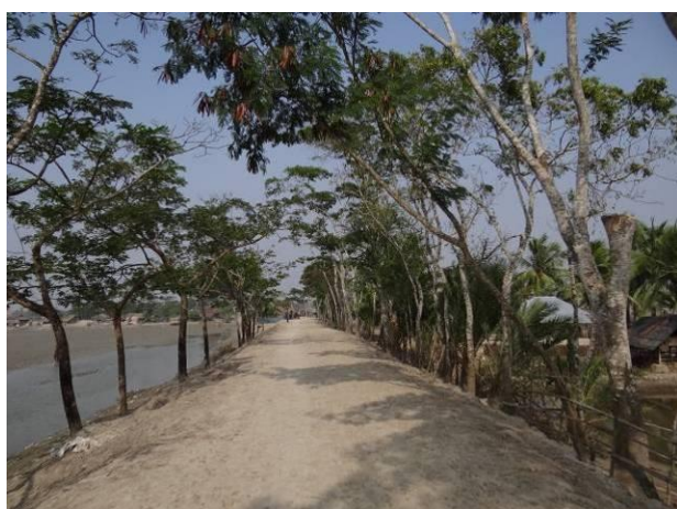
Figure 15: Embankment of the Polder
