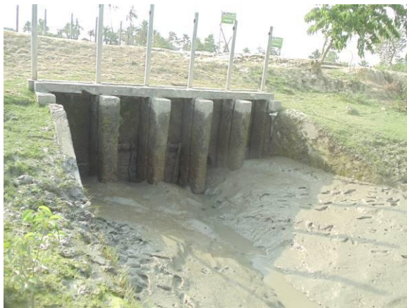
Figure 4.2: 5 vent Drainage Regulator
