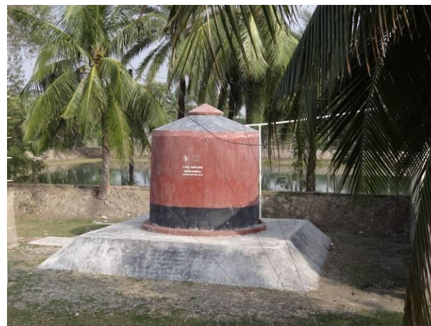
Figure 52: Pond Sand Filter (PSF)
