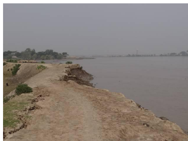
Figure 16: Embankment erosion the Dhaki River
