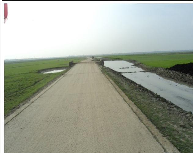
Submersible embankment made inside the haor, but soil to be collected from silt up beel that will be used as fish sanctuary, concern that top soil will not damage, make sure culvert to be installed in a suitable distance
