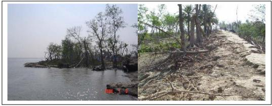
Figure 4-8 Damaged Coastal Polder 35/1 near Rayenda along Baleswar due to Sidr
