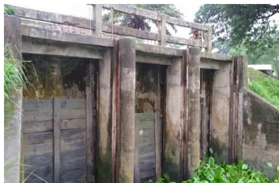
Picture 4.7: DS-4 (3V-1.5m X 1.8m) Sluice at Purbo Golkhali on Musir khal (Ch. 11.77 km)
