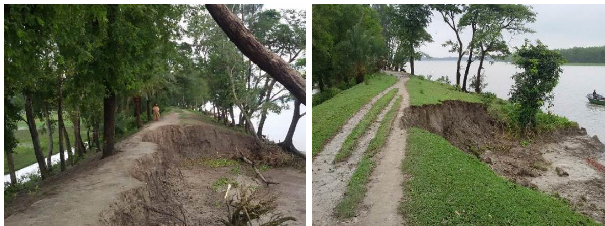
Picture 4.3: Erosion at Ch 13.20 to Ch14.00
