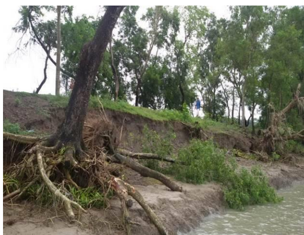
Picture 9: Breached Embankment
