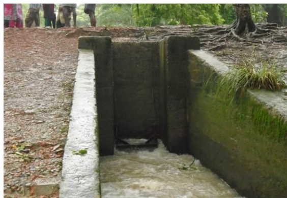
Picture4.9: DS-2 (1V-0.9m X 1.2m) Sluice at Jamal uddin khal (Ch. 22.375 km)
