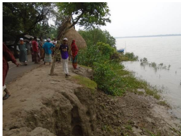
Picture 5.13: Erosion at Horidevpur Char Ch. 18+600 km to Ch. 19+700 km
