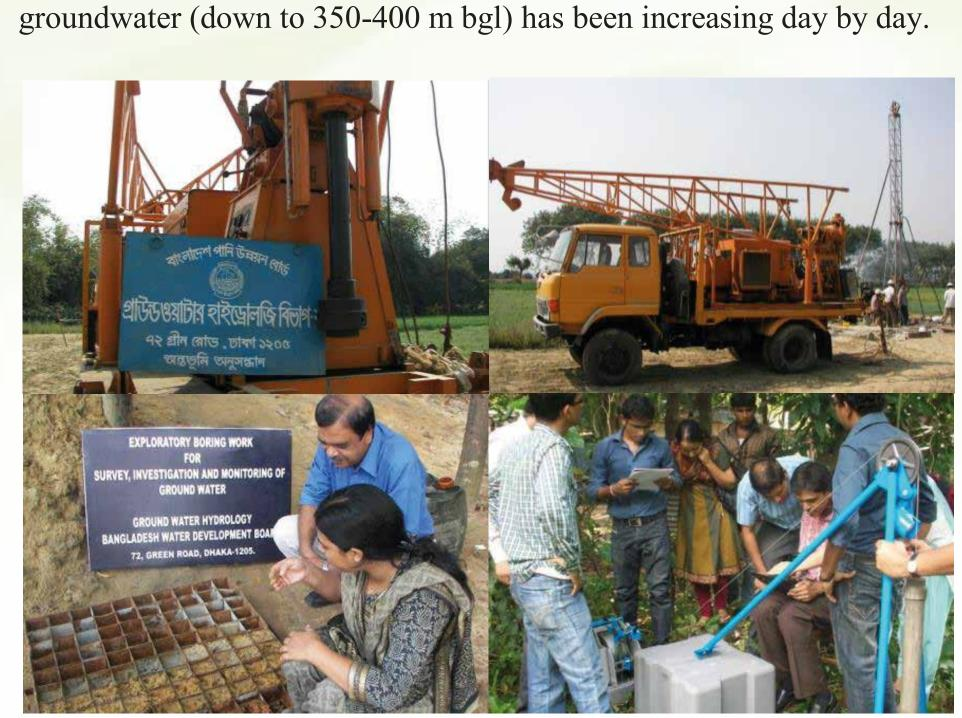
Figure 3: Activities including drilling of boreholes to investigate groundwater aquifer in Bangladesh.
