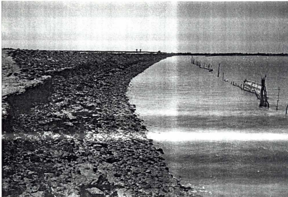
Urir Char cross dam, showing slope erosion
