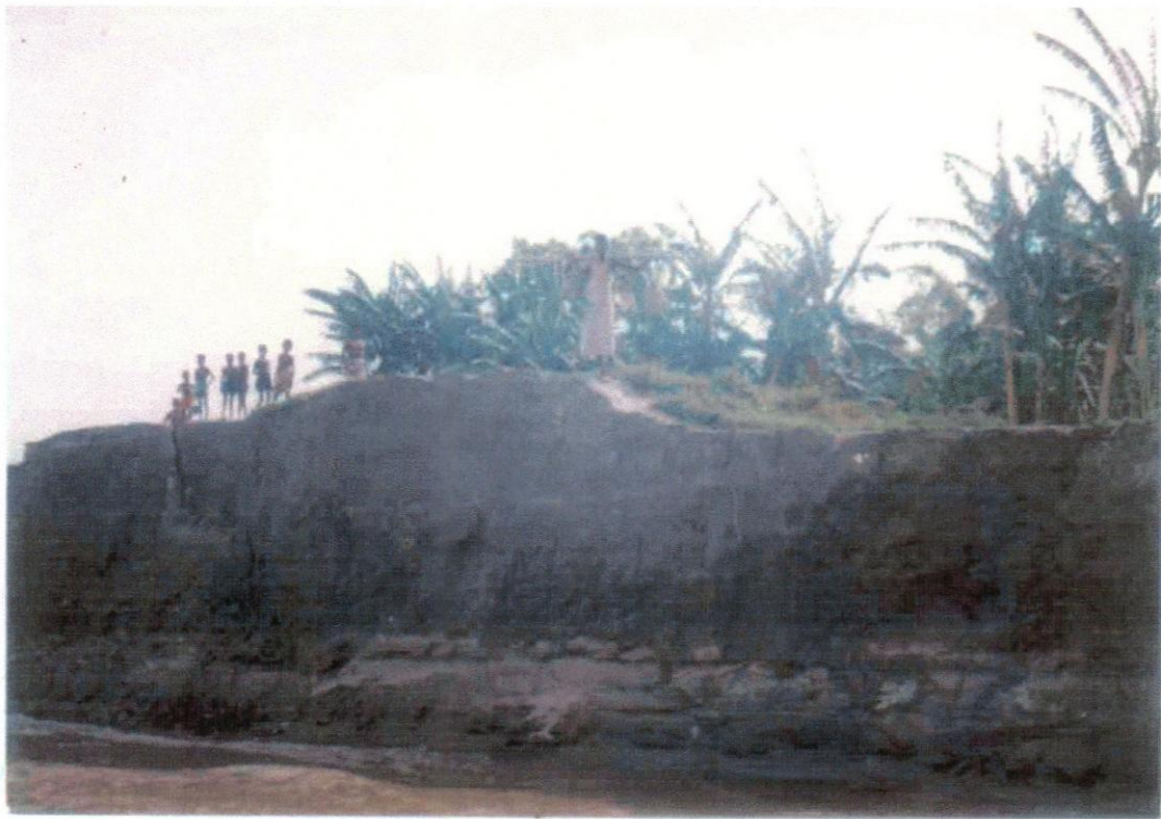
Plate-1: Bank erosion at the d/s of Bangabandhu bridge along the left bank
