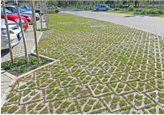
Permeable Pavement for Parking or Footpath
