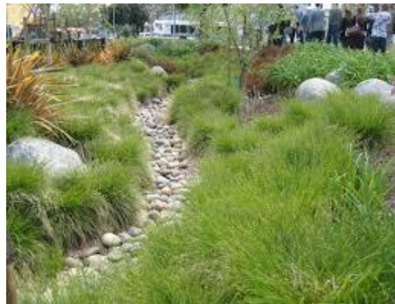
Infiltration Trench or Vegetative Swale
