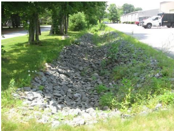
Infiltration Trench or Vegetative Swale
