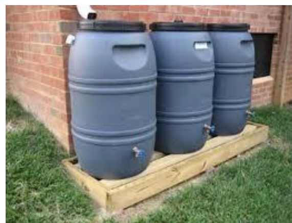
Low Cost Rain Barrel for Disconnection of Storm Water
