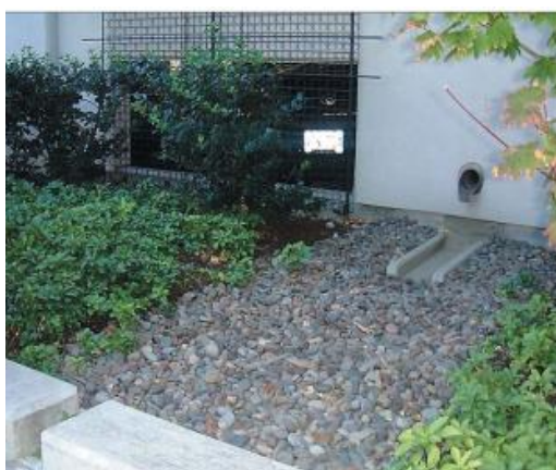
Disconnection of Rooftop Water through Infiltration Trench
