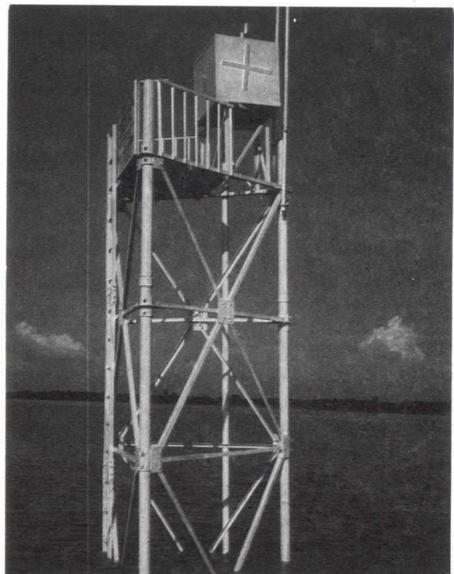
Figure 5.2: An ALWR (Automatic Water Level Recording) platform
