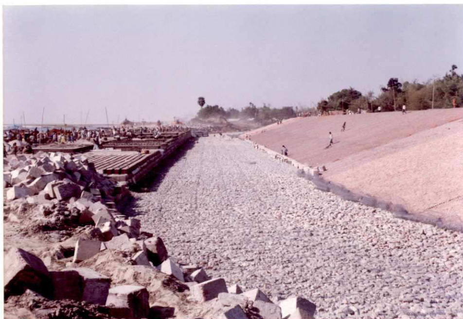
Photo 3: Test Site III – Ghutail; Middle section with (left to right) a. Falling Apron: randomly dumped cc-blocks and “in-situ casted” cc-blocks b. Launching Apron: boulder filled RENO-mattress c. Slope of Embankment: brick mattress
