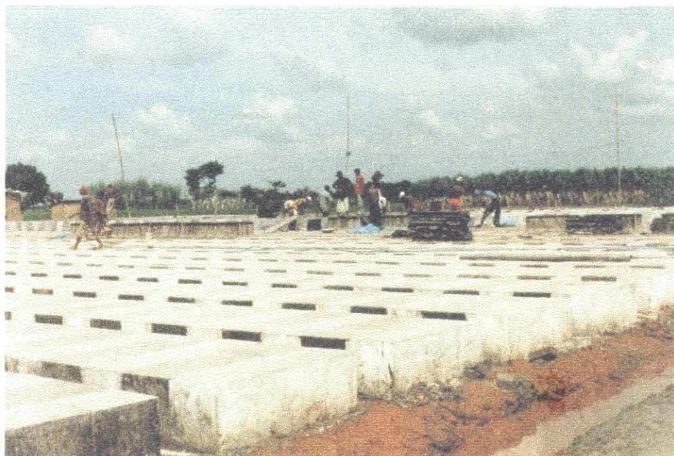
Photo 2: CC-block production in progress on September 20, 1999
