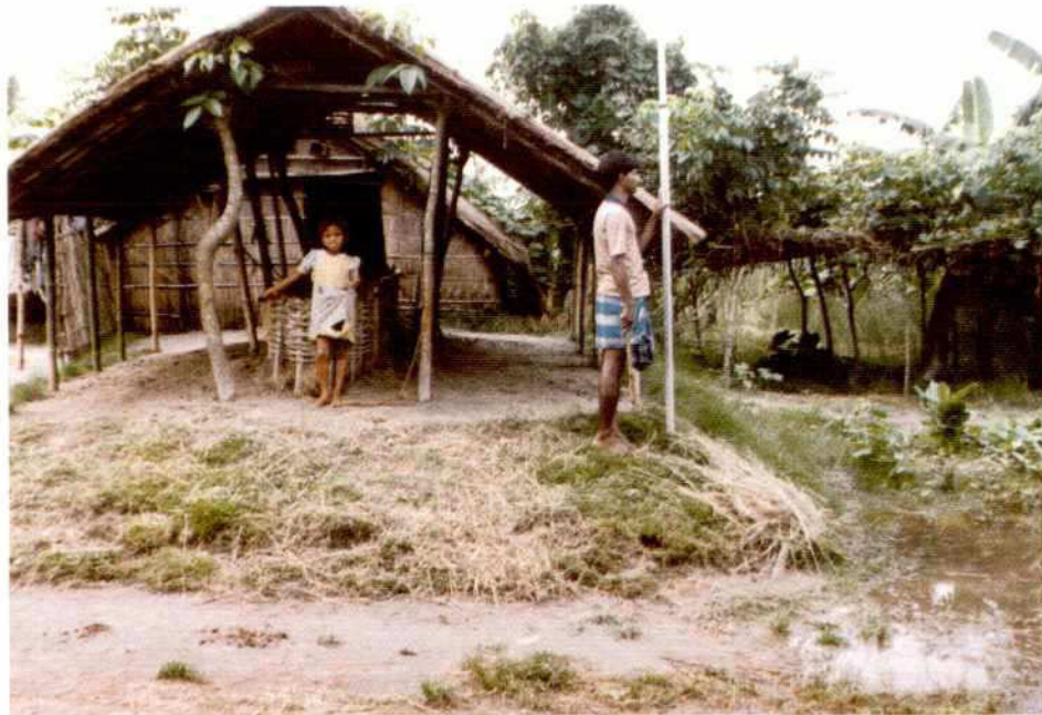
PLATE 3: Homestead cattle shelter. Note that the floor plinth is raised above the level of adjacent houses.
