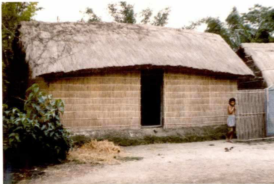
PLATE 2: Homestead living quarters. The raised floor plinth is a typical precaution against flooding, and the grass planted on the plinth protects its side slopes from wave action and rain.
