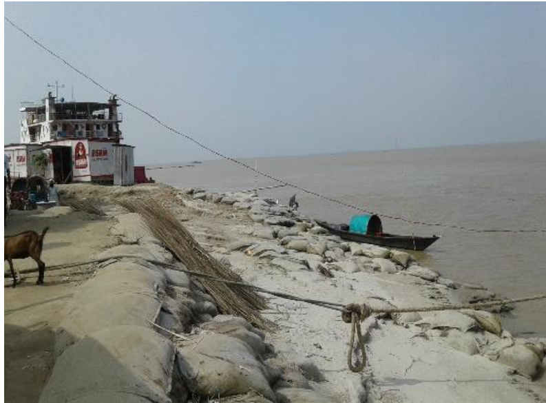
Figure 3.12: Protection work to safe Daulatdia ferry ghat through geo-bag dumping
