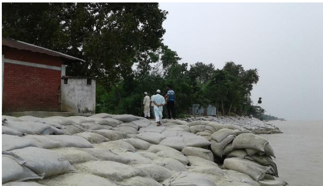
Figure 3.9: Bank protection work of BWDB at Urakandi Primary School, Rajbari, Rajbari
