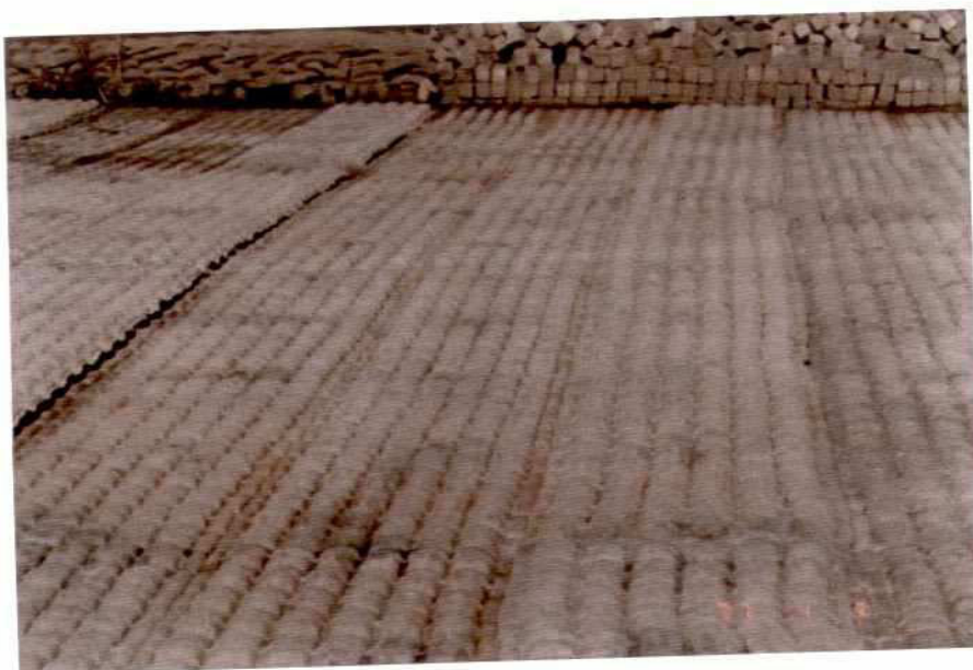
Photo 7.2-24: Section E Launching Apron: Filled Foreshore Cellular Geo-Textile Mattress Overlapping
