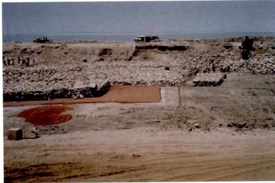
Photo 7.2-36: Section H-1 Falling Apron: Rip-Rap on Granular Filter
