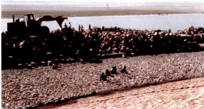
Photo 3.8-5: Downstream Termination A: Slope: Brick Mattressing on Geo-Textile Filter Mat B: Launching Apron: Wire mesh Mattress, Boulder fill C: Falling Apron: CC-Blocks
