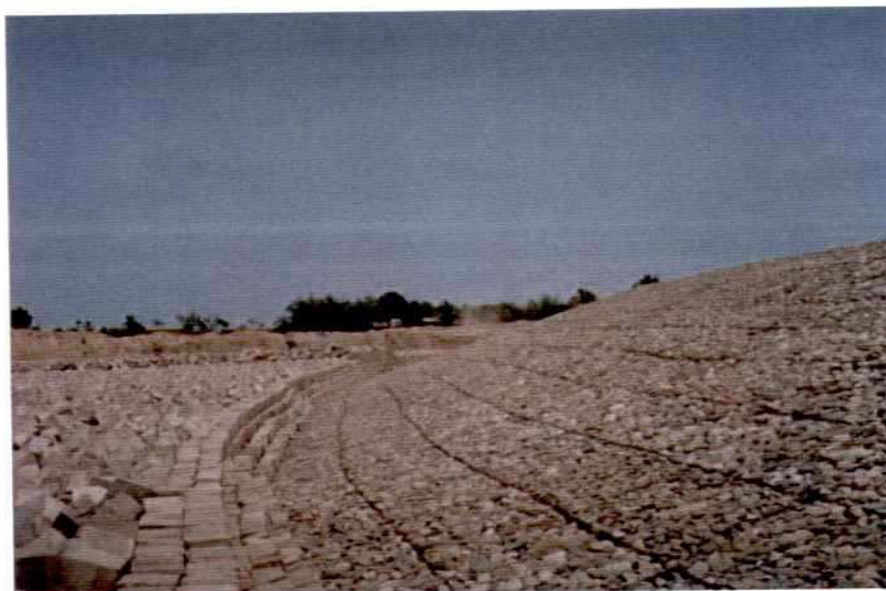
Photo 7.2-7: Section B Slope: Wiremesh Mattress (Reno), Boulder Fill Foot Stabilisation, CC-Blocks Launching Apron: CC-Blocks
