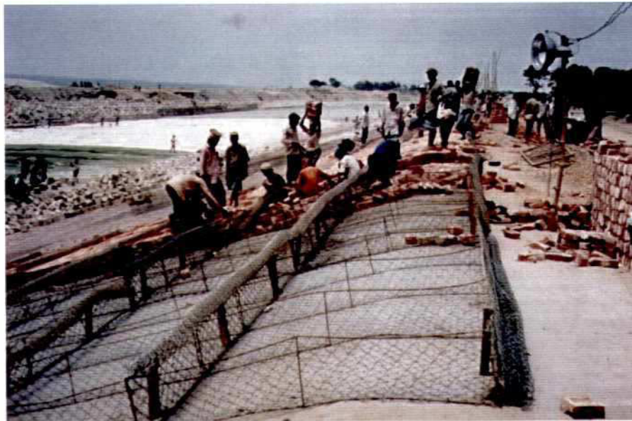
Photo 7.8-8: Wiremesh Mattress, Brick Filling
