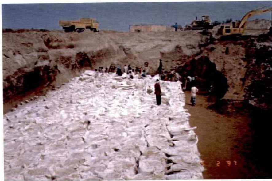
Photo 7.9-24: In Situ Filling of Sand Containers
