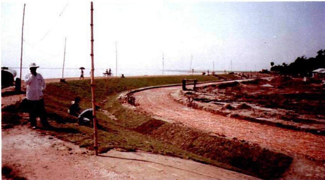
Photo 3.8-11: Embankment: Land sided slope, road construction
