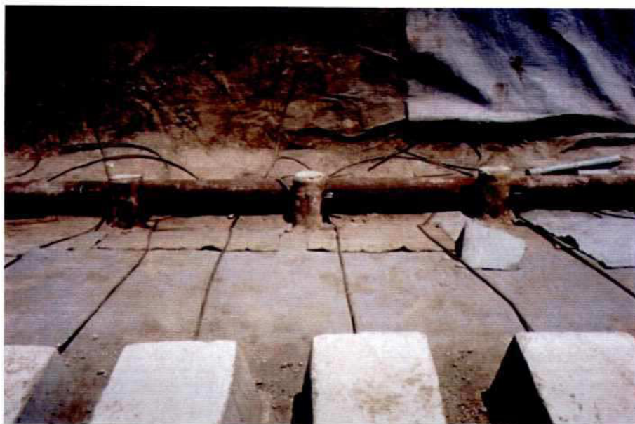
Photo 7.2-20: Section D Launching Apron: Articulated CC-Block Mattress Anchoring System
