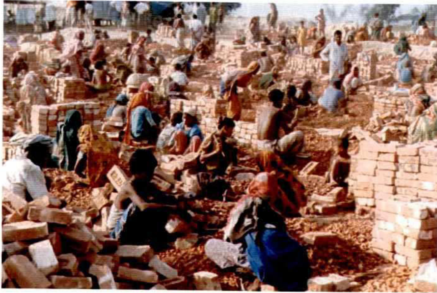
Photo 7.7-1: Brick Cutting for Aggregates and Filter Material
