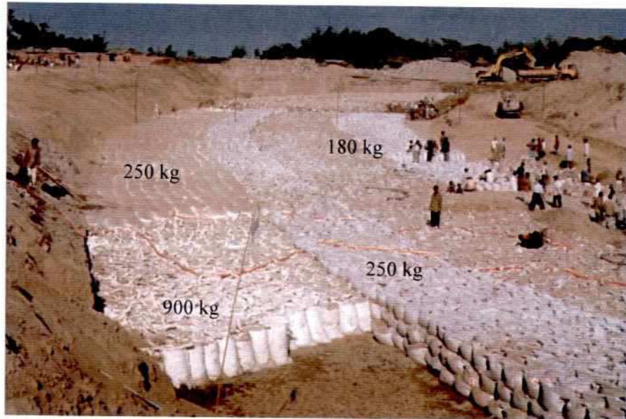
Photo 7.2-9: Section B Falling Apron: Geo-Textile Sand Containers
