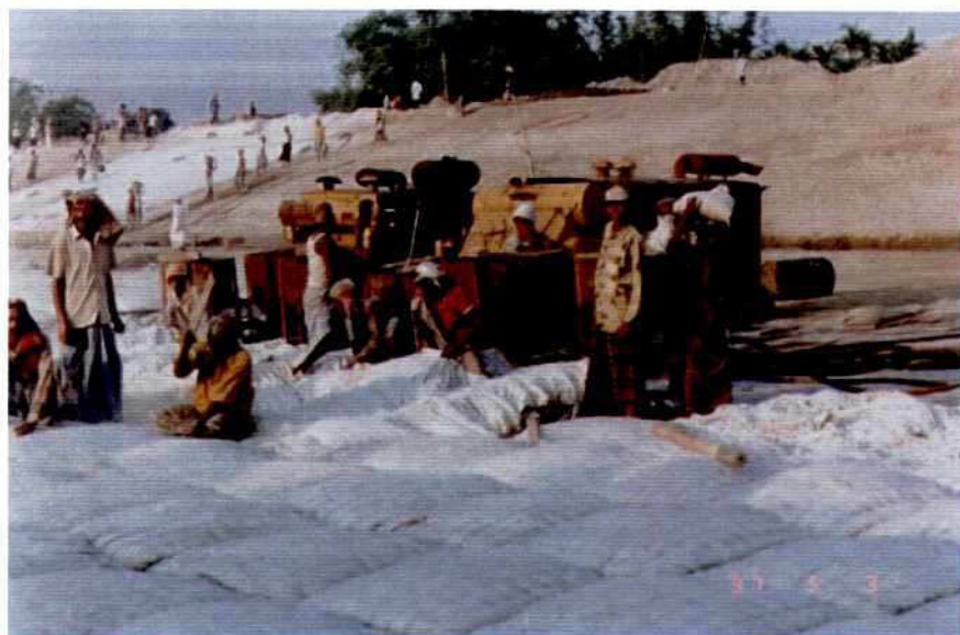
Photo 7.9-19: Sand Filled Cushion of Incomat Mattress
