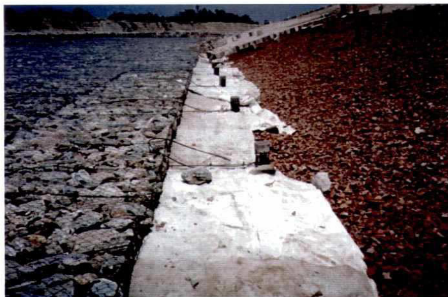
Photo 7.2-14: Section C Slope: Granular Filter, Khoa Launching Apron: Wiremesh Mattress (Reno), Anchor+Anchor Cable
