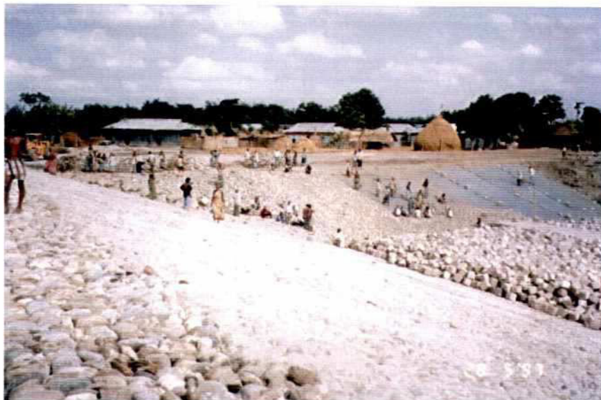
Photo 7.2-35: Section H-2, H-2 end Slope: Rip-Rap with Stone Pitching (Cement Grouting) Launching Apron: CC-blocks
