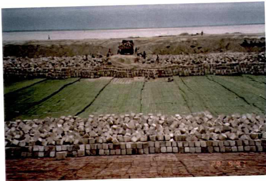
Photo 7.2-27: Section F Slope: Wiremesh Mattress, Brick Filled Foot Stabilisation CC-Blocks Launching Apron: Profix Cellular Geo-Textile Mattress Falling Apron: CC-Blocks
