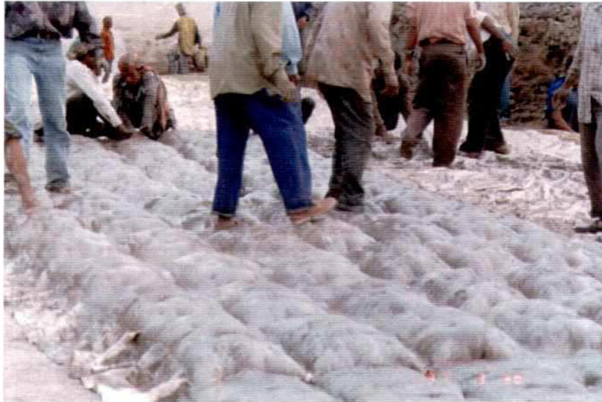
Photo 7.9-11: Foreshore Collapsible Mattress Filling by "Footstamping"
