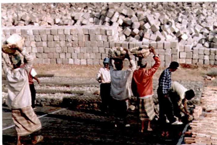
Photo 7.2-5: Section A-2 Slope: Geo-Textile Filter Mat Wiremesh Mattress (Reno), Boulder Fill Foot Stabilisation, CC-Blocks Launching Apron: CC-Blocks
