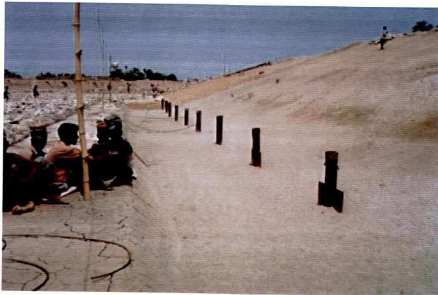
Photo 7.2-13: Section C Slope: Granular Filter, Khoa Launching Apron: Wiremesh Mattress (Reno), Anchor+Anchor Cable
