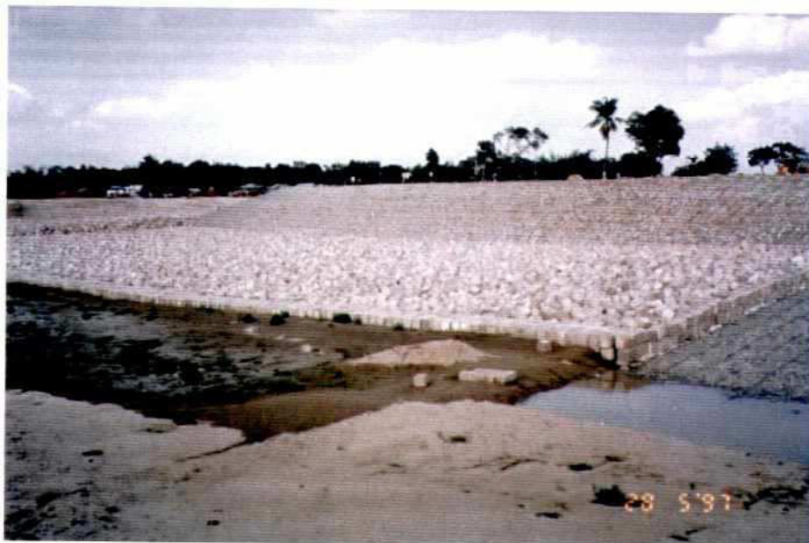
Photo 7.2-10: Section B Slope: Wiremesh Mattress (Reno), Boulder Fill Launching Apron: CC-Blocks Falling Apron: Geo-Textile Sand Containers (covered by earth fill)
