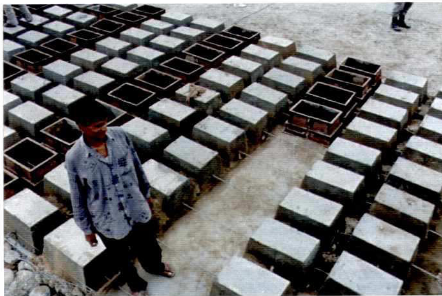
Photo 7.9-6: Articulated CC-Block Mattress Casting Form, Trapezoid CC-Blocks, Anchor Cable
