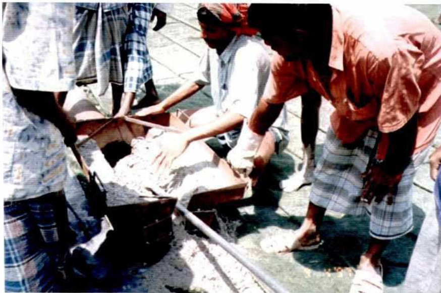
Photo 7.9-16: Filling of Tube of Profix Mat with Coarse Sand
