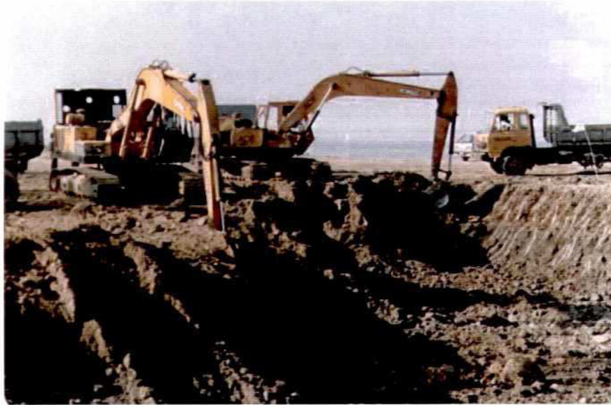
Photo 7.6-3: Mechanical Earth Works during Second Implementation Period 1996/1997 Excavation by Excavator (Backhoe)
