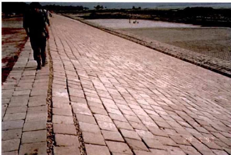
Photo 7.2-15: Section D Slope: CC-Blocks (parallel lines) Foot Stabilisation, CC-Blocks Launching Apron: Articulated CC-Block Mattress
