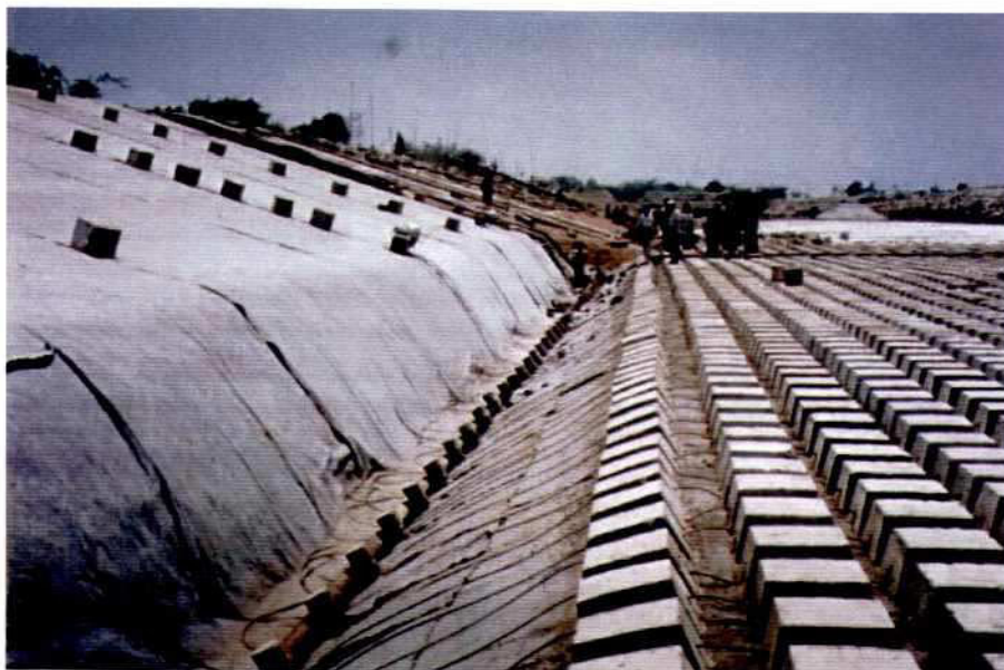
Photo 7.2-19: Section D Slope: Geo-Textile Filter Mat Anchor Trench Launching Apron: Articulated CC-Block Mattress Anchor, Cables
