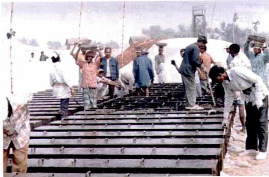
Photo 7.7-3: CC-Block Casting
