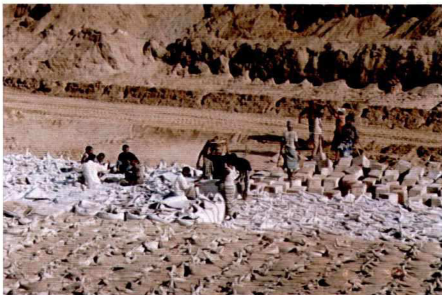
Photo 7.9-22: In Situ Filling of Sand Containers
