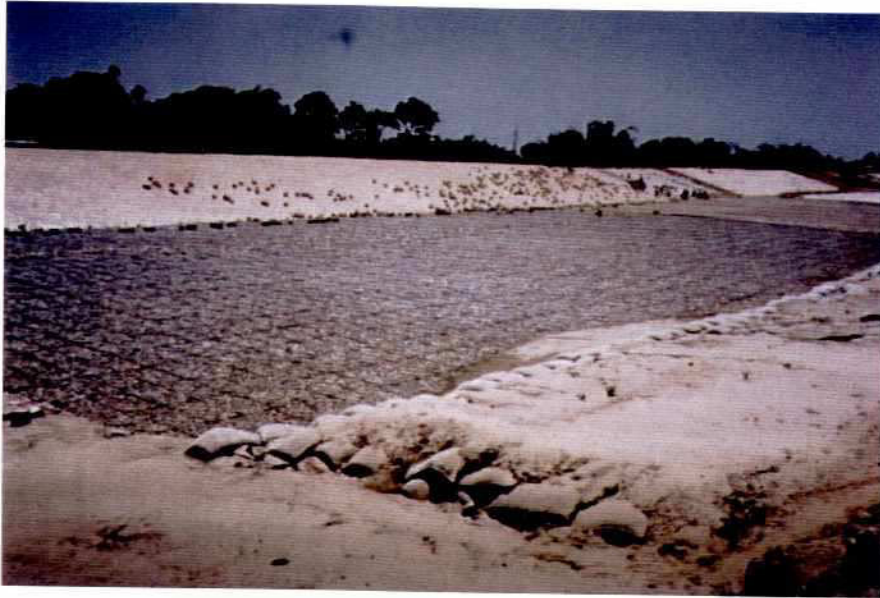
Photo 7.2-12: Section C Slope: CC-Blocks (diagonal lines) Launching Apron: Wiremesh Mattress (Reno), Boulder Filled Falling Apron: Geo-Textile Sand Containers (partly covered by earth fill)
