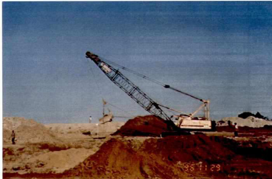
Photo 7.6-4: Mechanical Earth Works during Second Implementation Period 1996/1997 Excavation by Excavator (Dragline)
