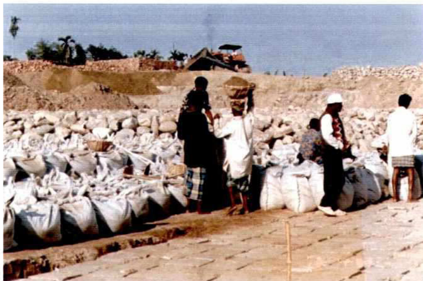
Photo 7.9-23: In Situ Filling of Sand Containers
