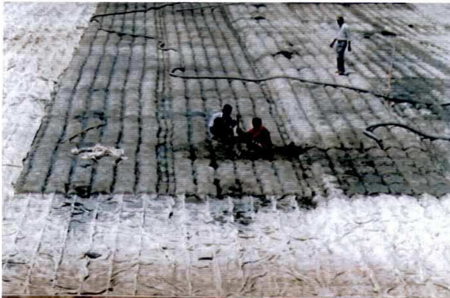
Photo 7.2-23: Section E Launching Apron: Foreshore Cellular Geo-Textile Mattress Filling with Concrete Grout
