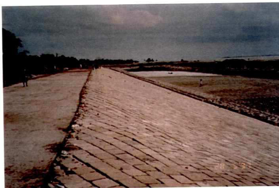
Photo 7.2-11: Section C Slope: CC-Blocks (diagonal lines)
