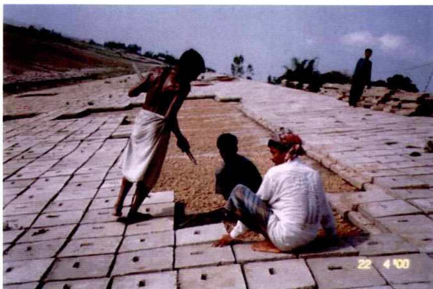
Photo 10.3-1: Section E; Repair of Slope Protection
