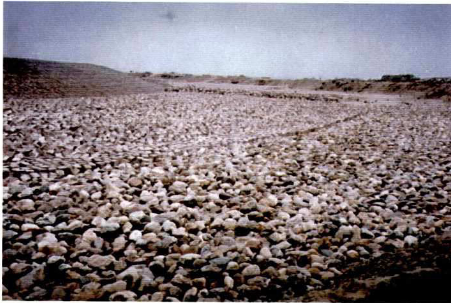
Photo 7.2-6: Section A-2 Slope: Wiremesh Mattress (Reno), Boulder Fill Launching Apron: CC-Blocks Transition, CC-Blocks Falling Apron: Rip-Rap
