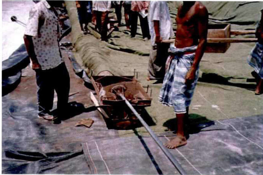
Photo 7.9-15: Filling of Tube of Profix Mat with Sand-Bitumen
