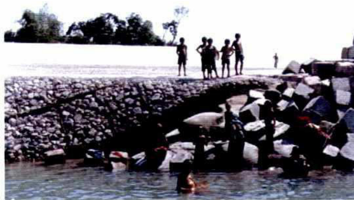
Fig. 4.3-1: Articulated RENO-mattress system after exposure to erosion attack
