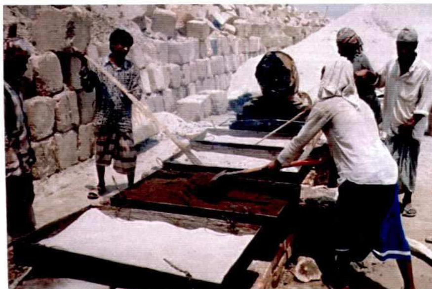
Photo 7.9-14: Drying of Coarse Sand and Mixing of Sand-Bitumen for Filling of Profix Mat
