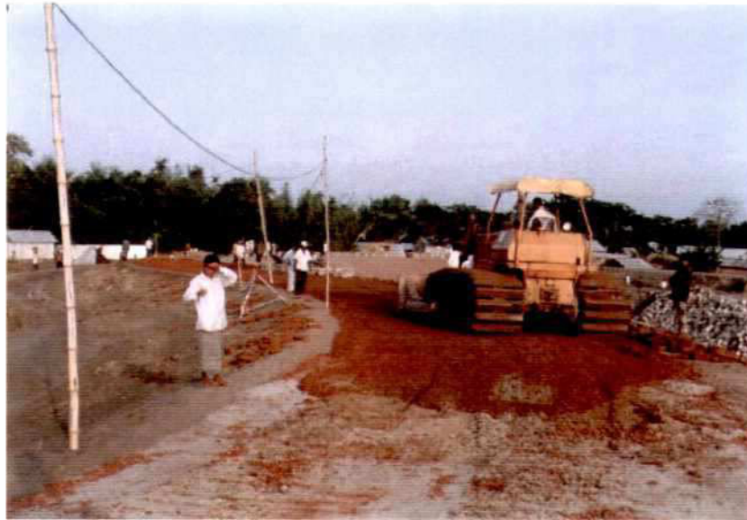
Photo 3.8-10: Embankment Crest Finishing with Khoa sand mix
