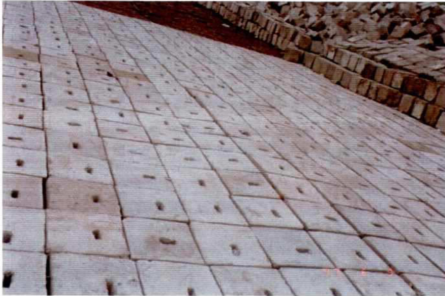
Photo 7.2-22: Section E Slope: Double Interlocking CC-Slabs (Ship-Lap Type) Foot Stabilisation, CC-Blocks
