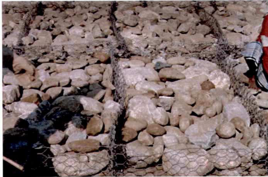
Photo 7.9-2: Wiremesh (Reno) Mattress, Boulder Filling
