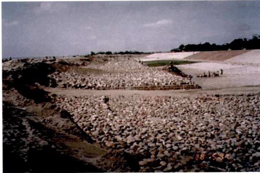
Photo 7.2-33: Section G Launching Apron: Incomat Sandflex Mattress Falling Apron: CC-Blocks (Foreground Section H, F.-A.: Selected Boulders)
