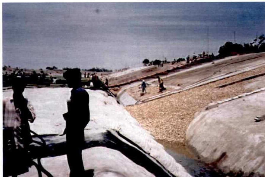
Photo 7.8-4: Trench between Slope and L.-A. filled with Gravel (here Section G)
