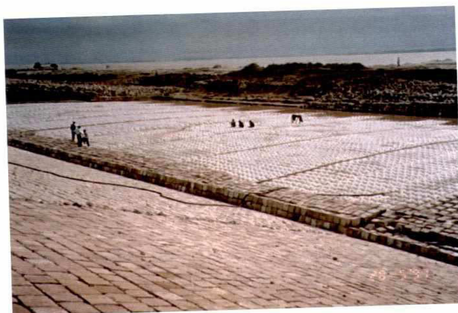
Photo 7.2-25: Section E Launching Apron: Foreshore Cellular Geo-Textile Mattress (Foreground: Slope of Section D)
