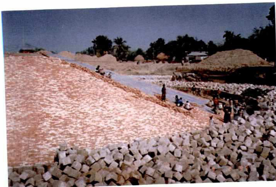
Photo 7.2-2: Section A-1 Slope: Brick Mattress Launching Apron: CC-Blocks
