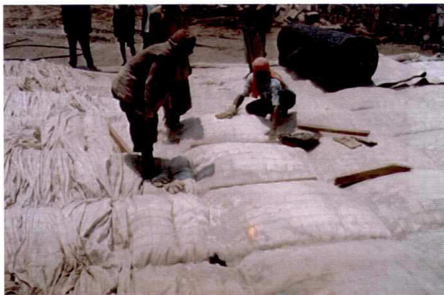
Photo 7.9-20: Sand Filled Cushion Of Incomat Mattress
