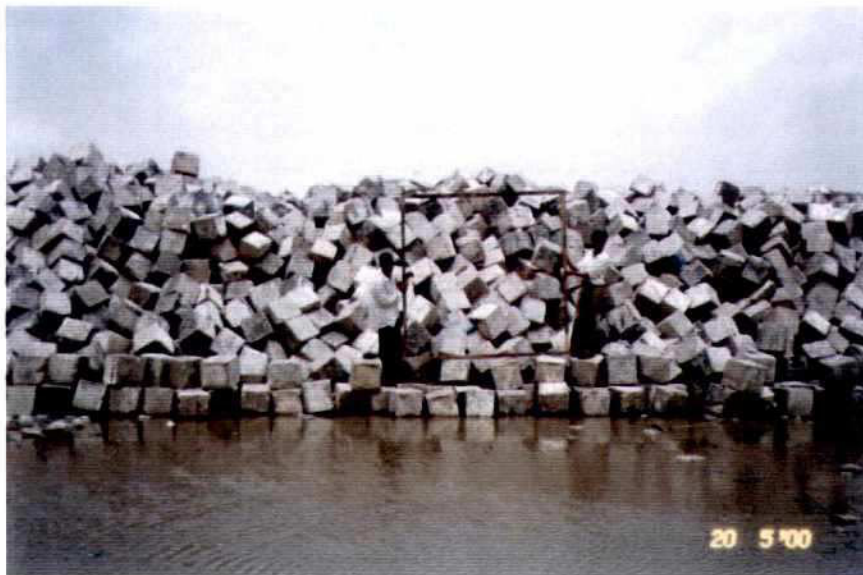
Photo 3.8-6: Falling Apron: CC-Blocks randomly dumped
