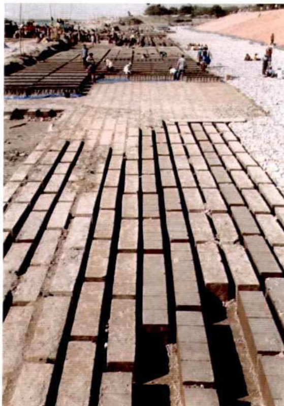
Photo 3.8-8: Launching Apron: CC-Blocks, In-situ cast
