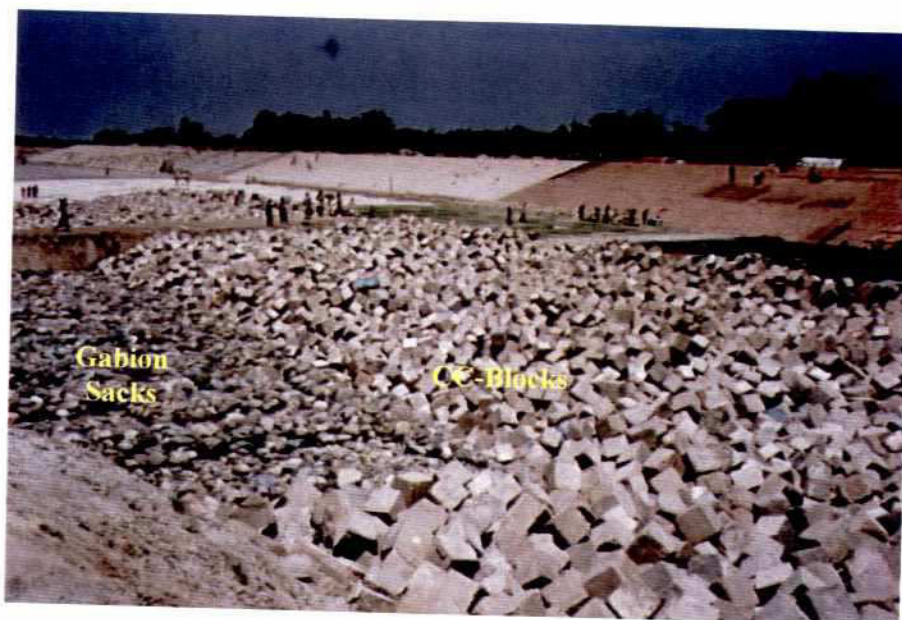
Photo 7.2-28: Section F Falling Apron: CC-Blocks, Gabion Sacks
