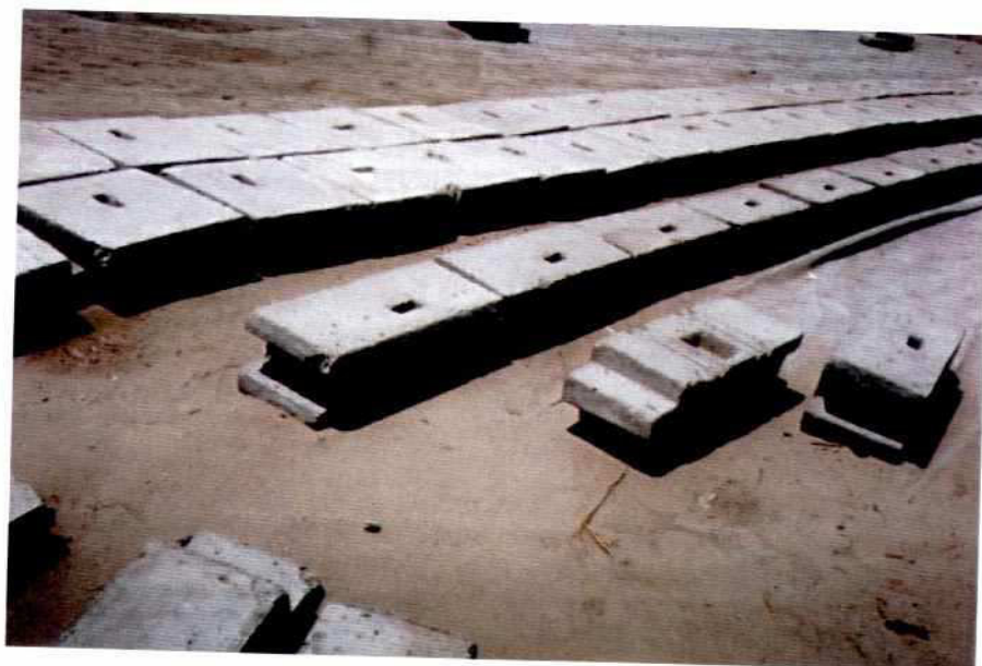
Photo 7.2-29: Section G Slope: Interlocking CC-Slabs (Tongue +Grove Type)
