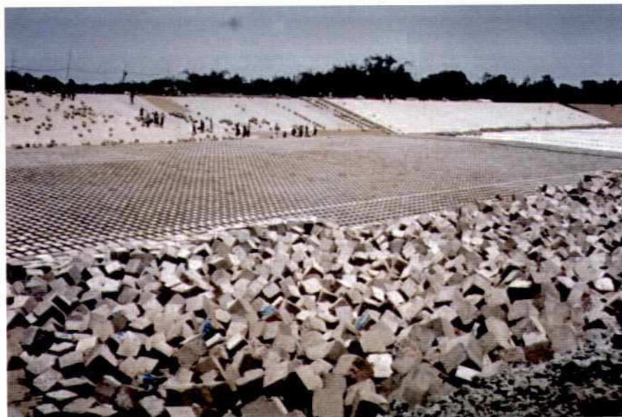
Photo 7.2-18: Section D Slope: CC-Blocks (parallel lines) Launching Apron: Articulated CC-Block Mattress Falling Apron: CC-Blocks
