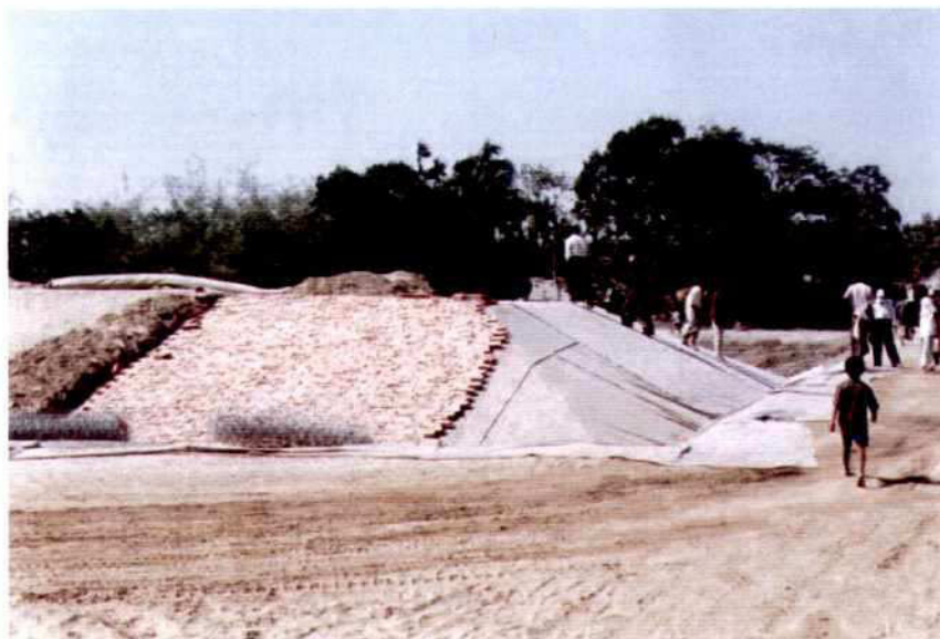
Photo 3.8-3: Upstream Termination, Brick mattressing on Geotextile Filter Mat
