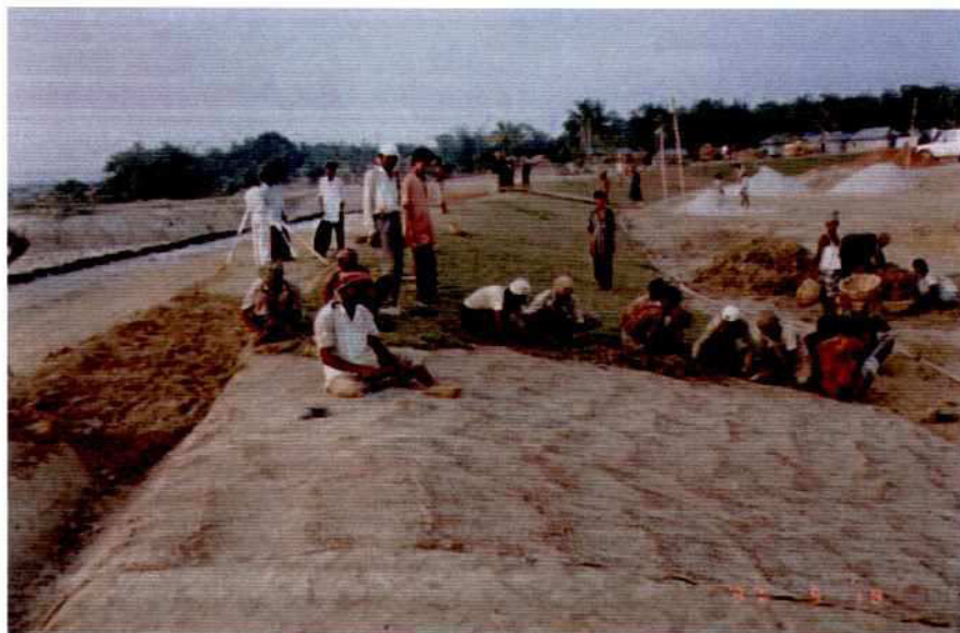
Photo 7.6-5: Embankment; Grass Sodds on Geo-Jute Soil Saver Mat
