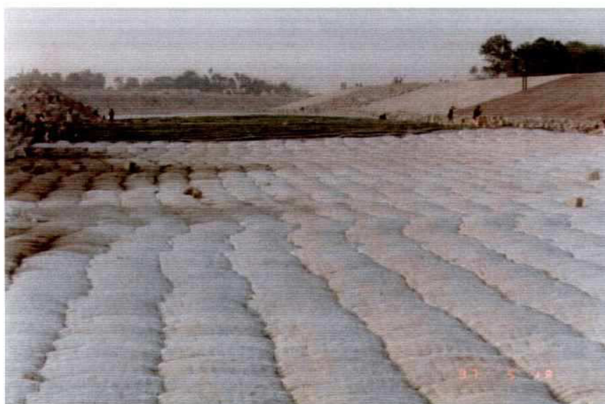
Photo 7.2-32: Section G Launching Apron: Incomat Collapsible Sandflex Mattress, Sand Filled
