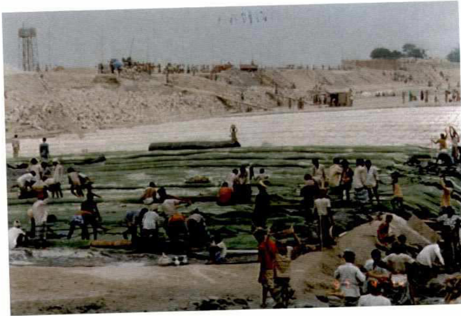
Photo 7.2-26: Section F Launching Apron: Foreshore Cellular Geo-Textile Mattress
