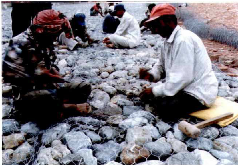
Photo 3.8-2: Closing of Wire mesh mattress
