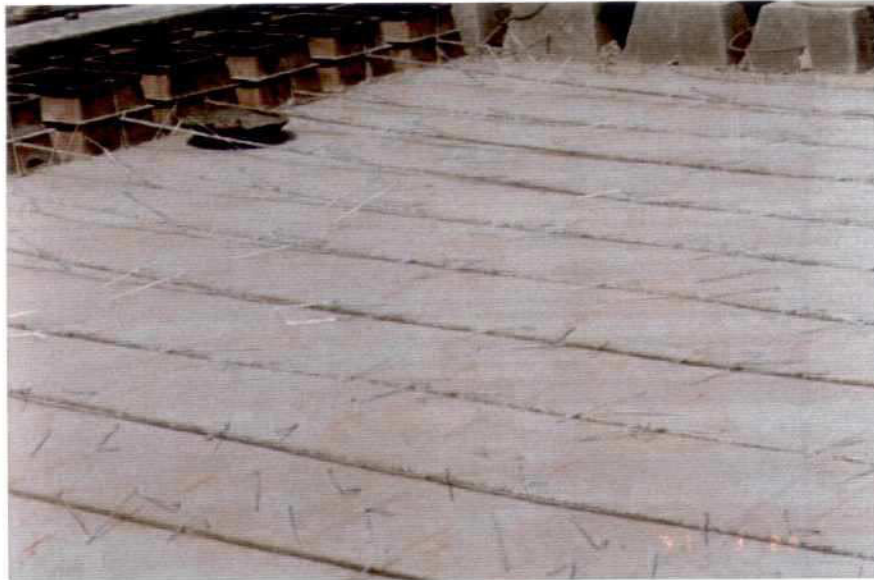
Photo 7.9-5: Articulated CC-Block Mattress Geo-Textile Filter Mat Needle Punched
