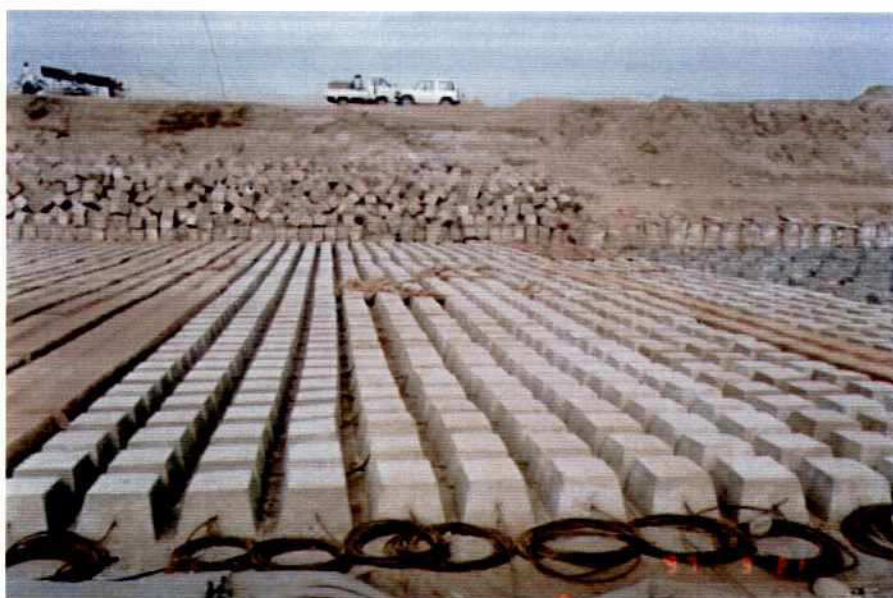
Photo 7.2-16: Section D Launching Apron: Articulated CC-Block Mattress Anchor Cables Falling Apron: CC-Blocks
