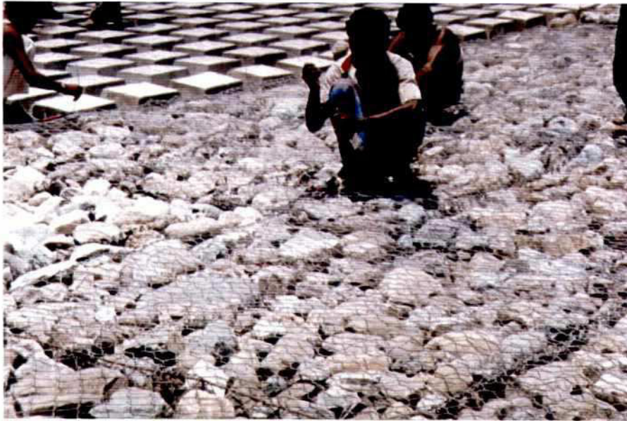
Photo 7.9-4: Closing of Wiremesh Mattress
