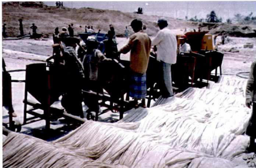
Photo 7.9-17: Filling of Incomat Collapsible Sandflex Mattress with Dry Coarse Sand By "Air Stream Blasting"
