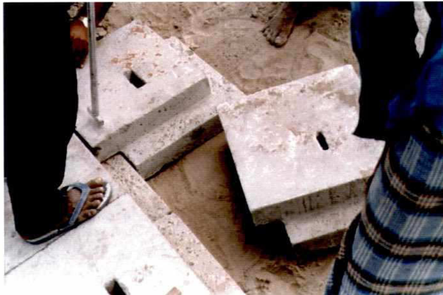
Photo 7.2-21: Section E Double Interlocking CC-Slab (Ship-Lap Type)
