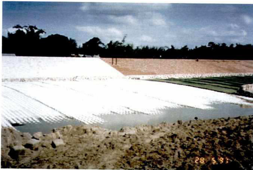
Photo 7.9-26: Overlapping (Section E, Foreshore Mattress)
