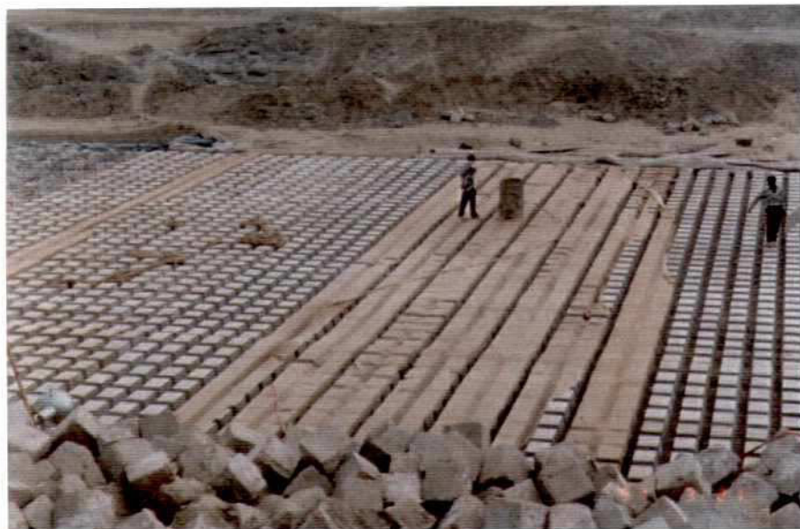
Photo 7.2-17: Section D Launching Apron: Articulated CC-Block Mattress Falling Apron: CC-Blocks
