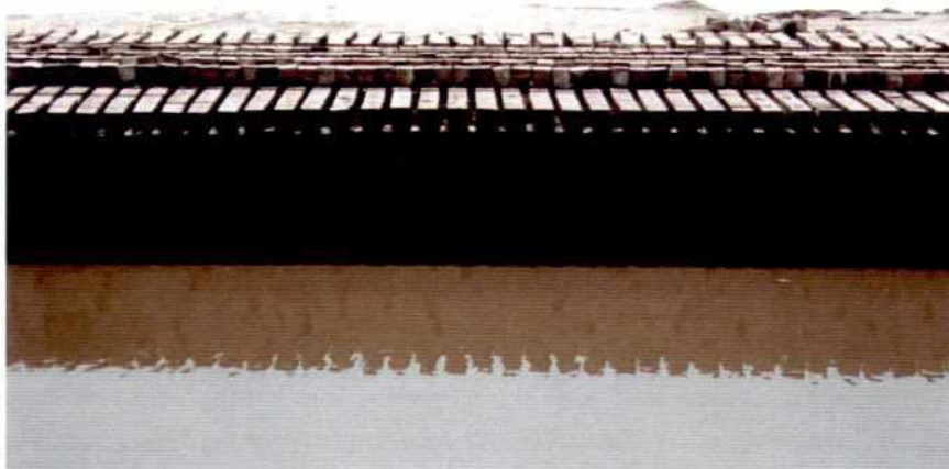
Photo 3.8-7: Launching Apron: CC-Blocks, In-situ cast
