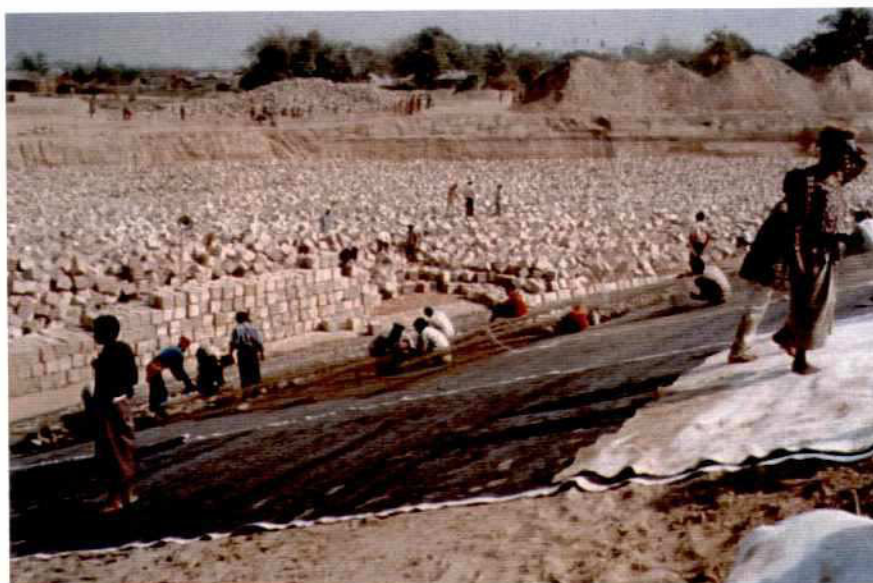
Photo 7.2-4: Section A-2 Slope: Geo-Textile Filter Mat Foot Stabilisation, CC-Blocks Launching Apron: CC-Blocks Falling Apron: Rip-Rap
