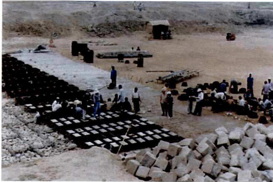
Photo 7.9-7: Articulated CC-Block Mattress
