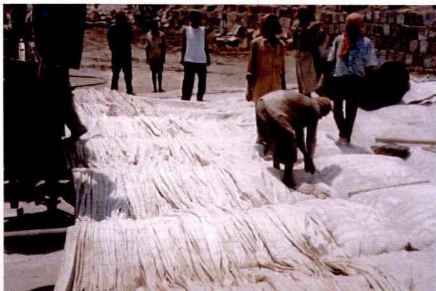
Photo 7.9-18: Filling of Incomat Collapsible Sandflex Mattress with dry Coarse Sand by “Air Stream Blasting”
