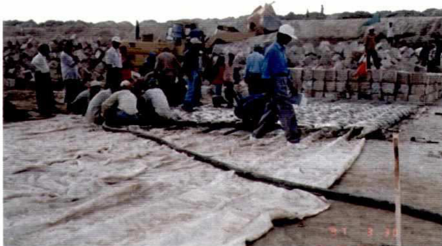
Photo 7.9-10: Foreshore Collapsible Mattress Filling with Cement Grout (Colcrete)
