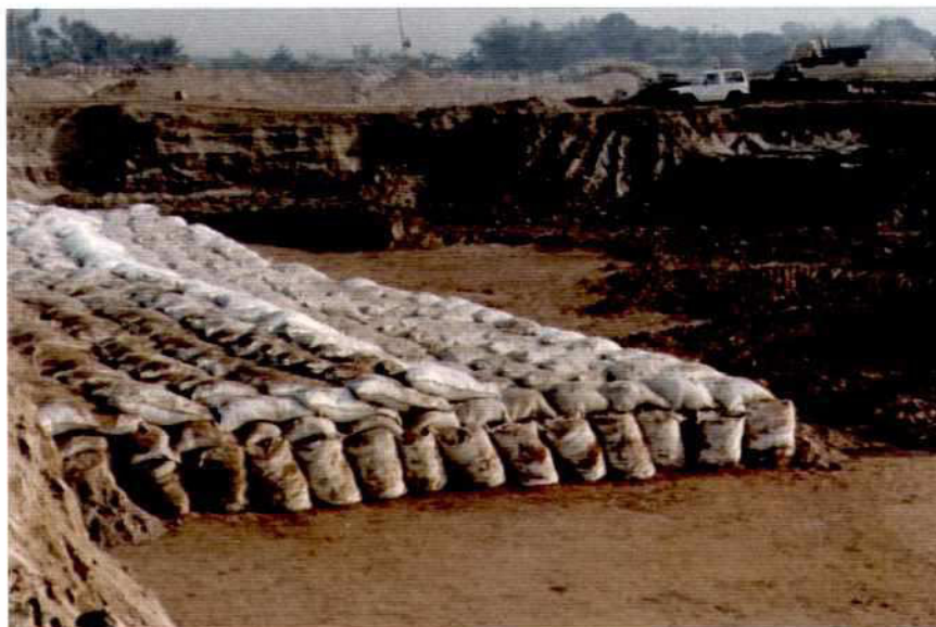
Photo 7.9-21: Geo-Textile Sand Container (Type E, 900 kg)
