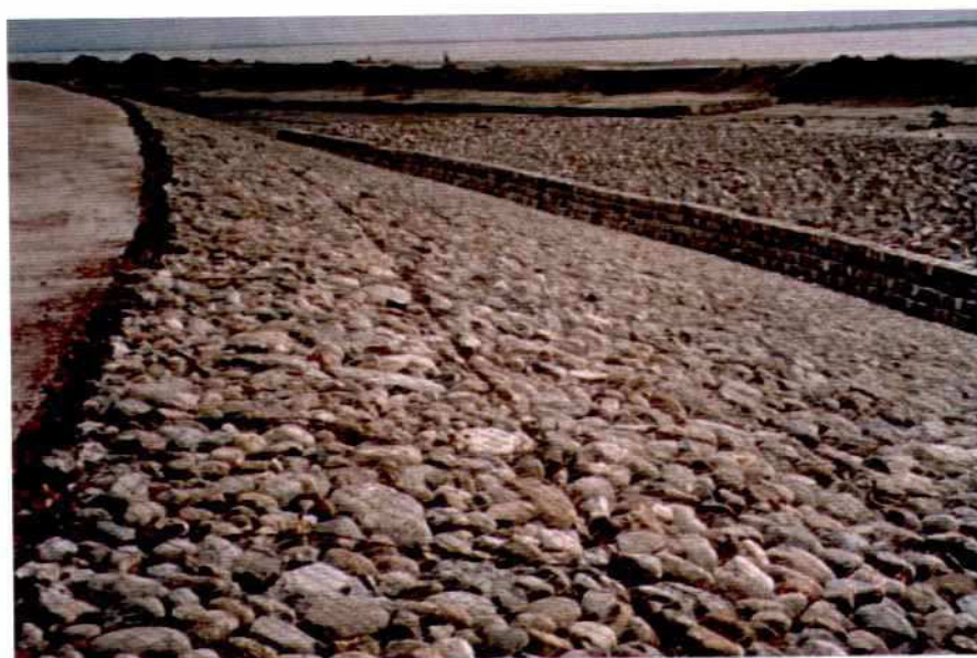
Photo 7.2-8: Section B Slope: Wiremesh Mattress (Reno), Boulder Fill Foot Stabilisation, CC-Blocks Launching Apron: CC-Blocks
