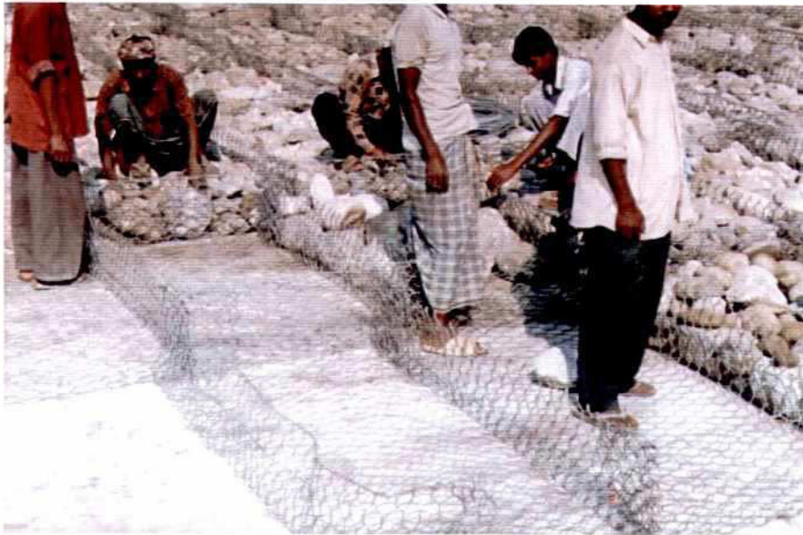
Photo 7.9-1: Wiremesh (Reno) Mattress, Boulder Filling
