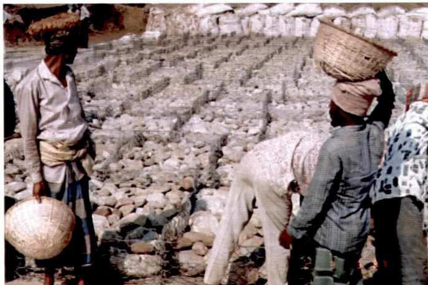
Photo 7.9-3: Wiremesh (Reno) Mattress, Boulder Filled
