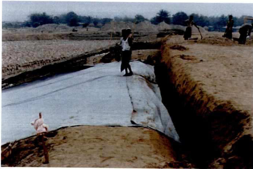
Photo 7.8-1: Laying Out of Geo-Textile Filter Mat
