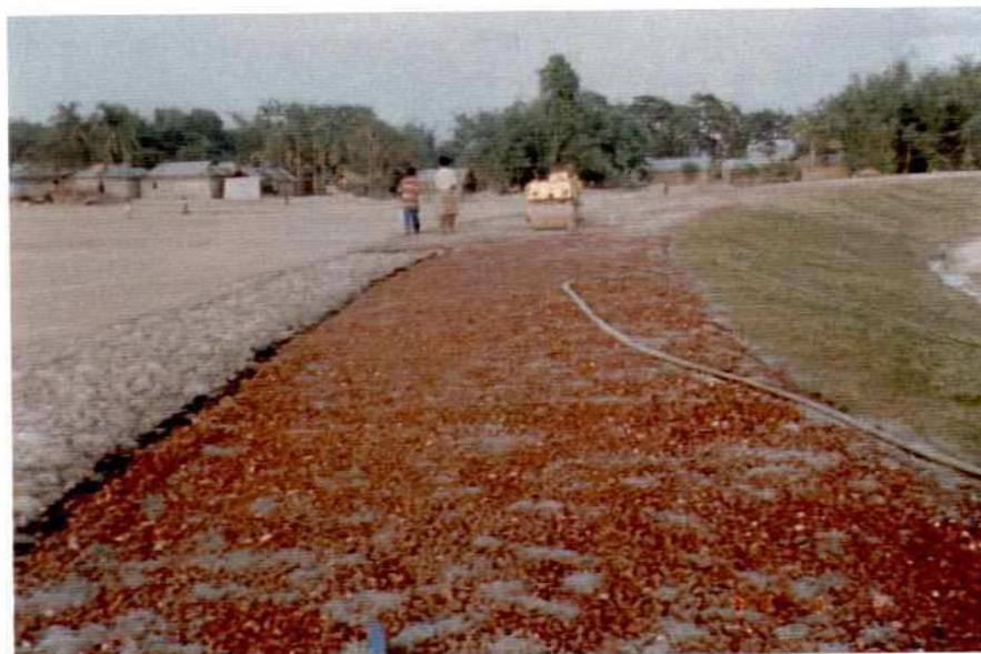
Photo 7.6-6: Embankment; Crest Finishing with compacted Khoa-Sand Mix
