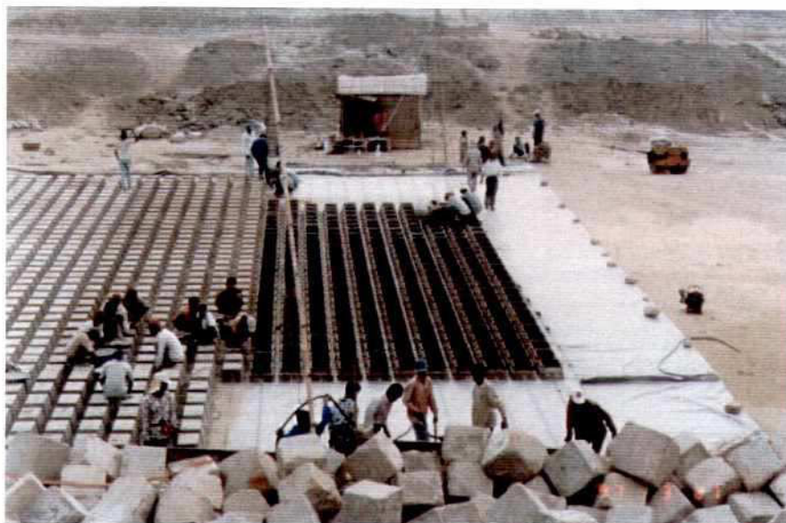
Photo 7.9-8: Articulated CC-Block Mattress
