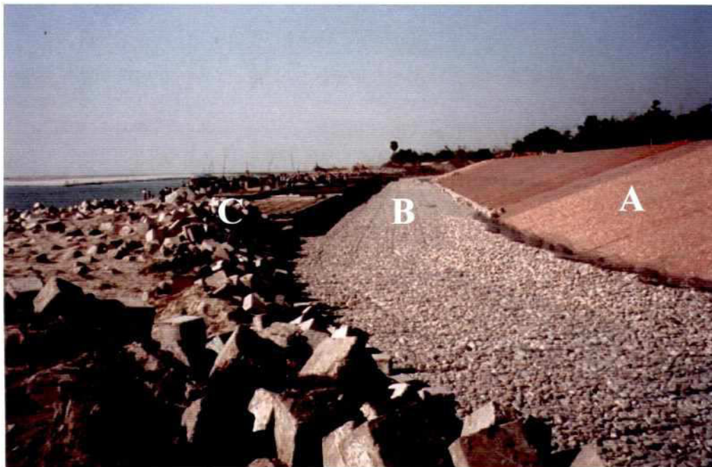
Photo 3.8-1: General view of Ghutail Revetment Test Structure with A: Slope of embankment: Brick Mattress B: Launching Apron: Wire mesh Mattress (Reno) boulder filled C: Falling Apron: CC-Blocks
