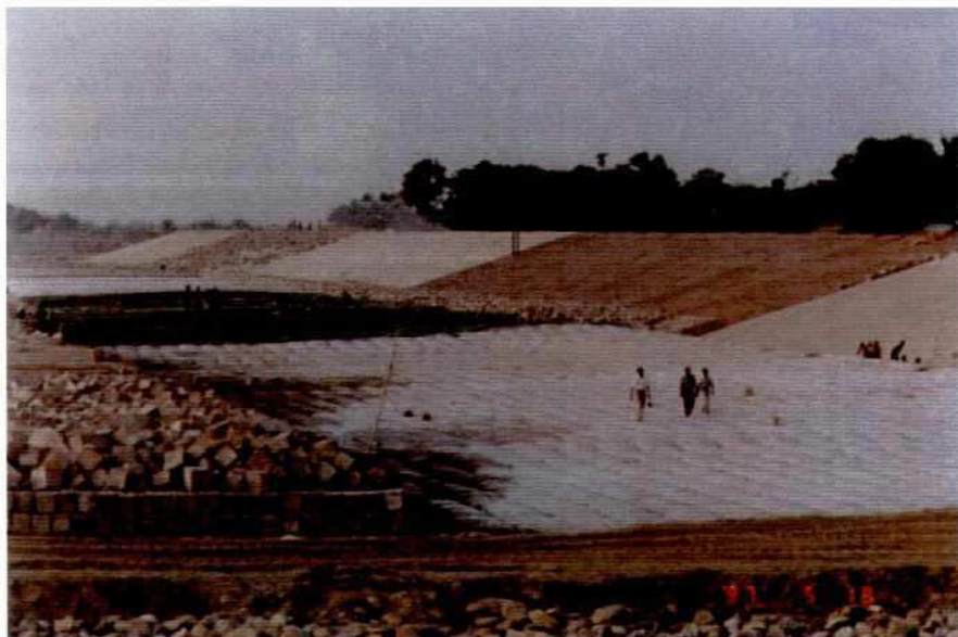
Photo 7.2-31: Section G Launching Apron: Incomat Collapsible Sandflex Mattress Falling Apron: CC-Blocks
