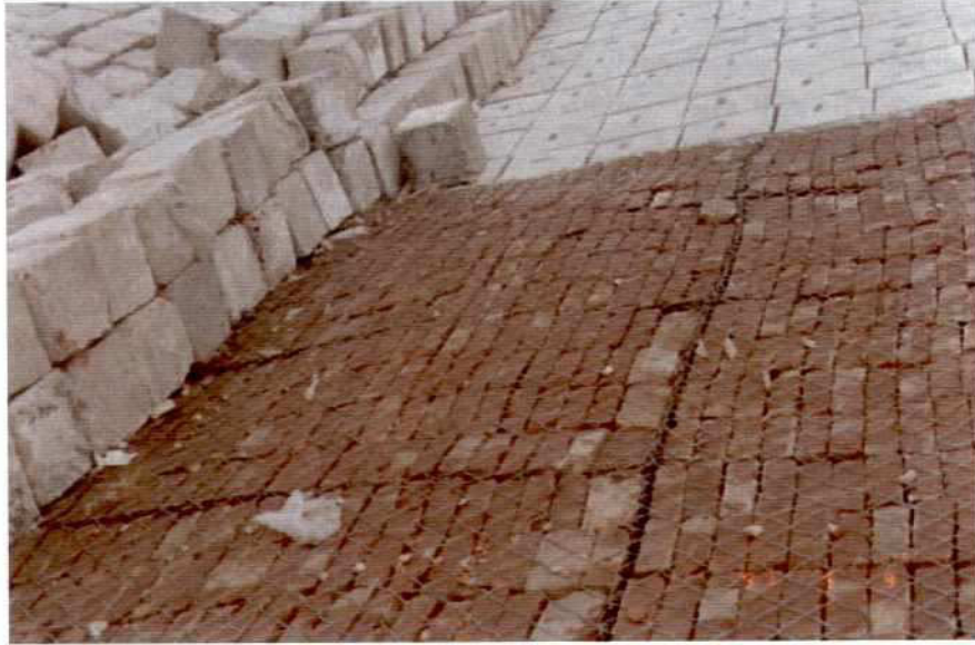
Photo 7.8-7: Wiremesh Mattress, Brick Filling
