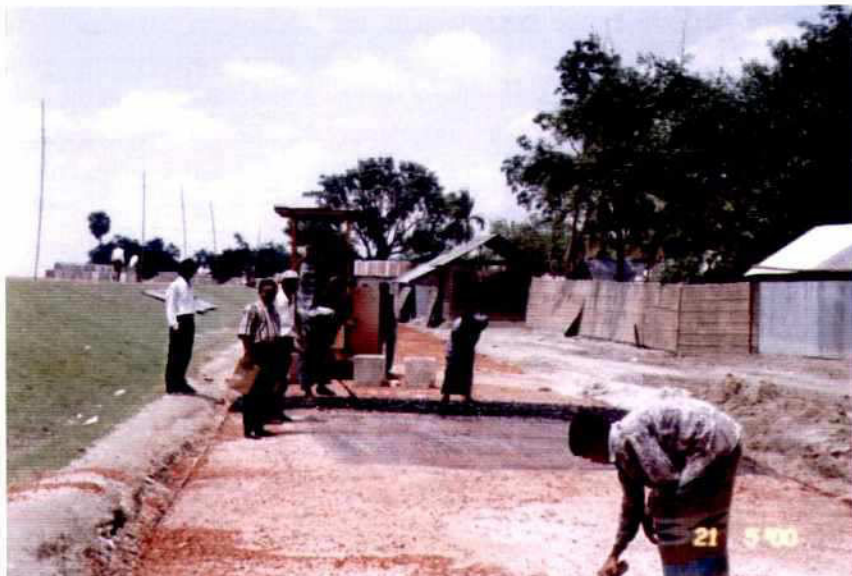
Photo 3.8-12: Road construction: Bituminising
