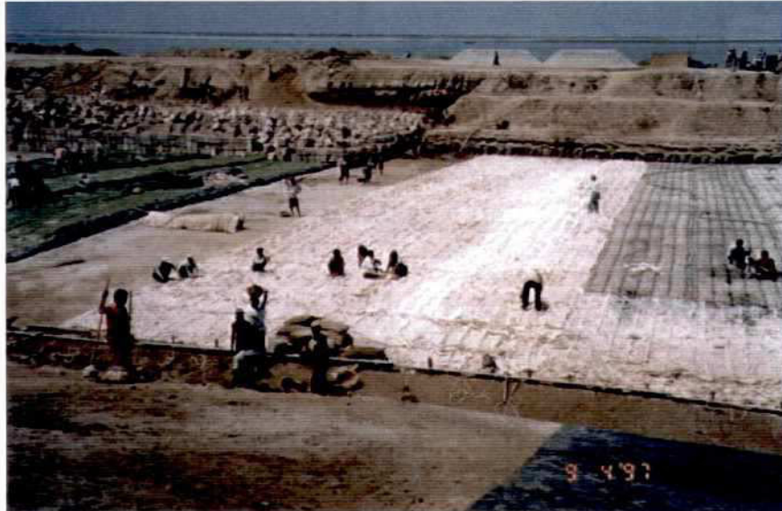
Photo 7.9-9: Foreshore Collapsible Mattress
