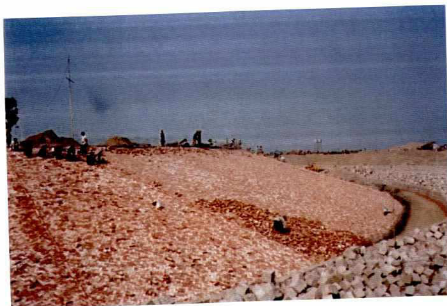
Photo 7.2-3: Section A-1 end Slope: Brick Mattress Trench for Foot Stabilisation Launching Apron: CC-Blocks
