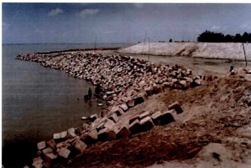
Photo 10.3-2: Section H Repair of Falling Apron
