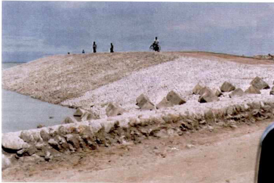
Photo 7.2-34: Section H-1, H-2 Slope: Rip-Rap with Stone Pitching (Cement Grouting)
