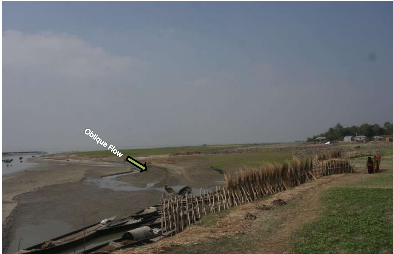
Figure 5.46 Oblique flow from main channel hit to the bandal-like structures in Jamuna River
