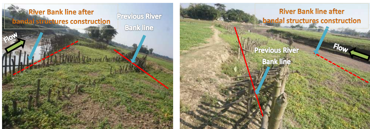
Figure 5.31 Sediment depositions on river bank induced by bandal-like structures at the Nitai River (u/s of Shankarpur Bazar, Purbadhala)
