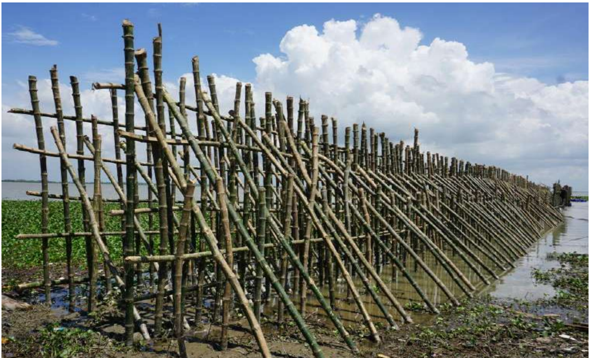
Figure 4.3 Constructed bandal structures at Enayetpur, Sirajgonj as per Design
