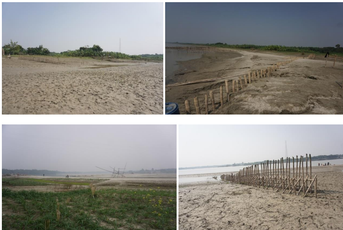
Sediment depositions on river bank induced by bandal-like structures at the left bank of Madhumati River (d/s of Kamarkhali Bridge)
