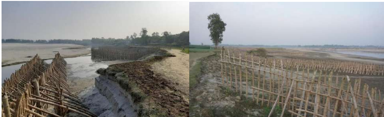
Figure 4.22 Bandal structures at Neorgacha, Chouhali
