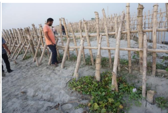
Sediment depositions on river bank induced by bandal-like structures at the right bank of Jamuna River (d/s of Enayetpur Spur)
