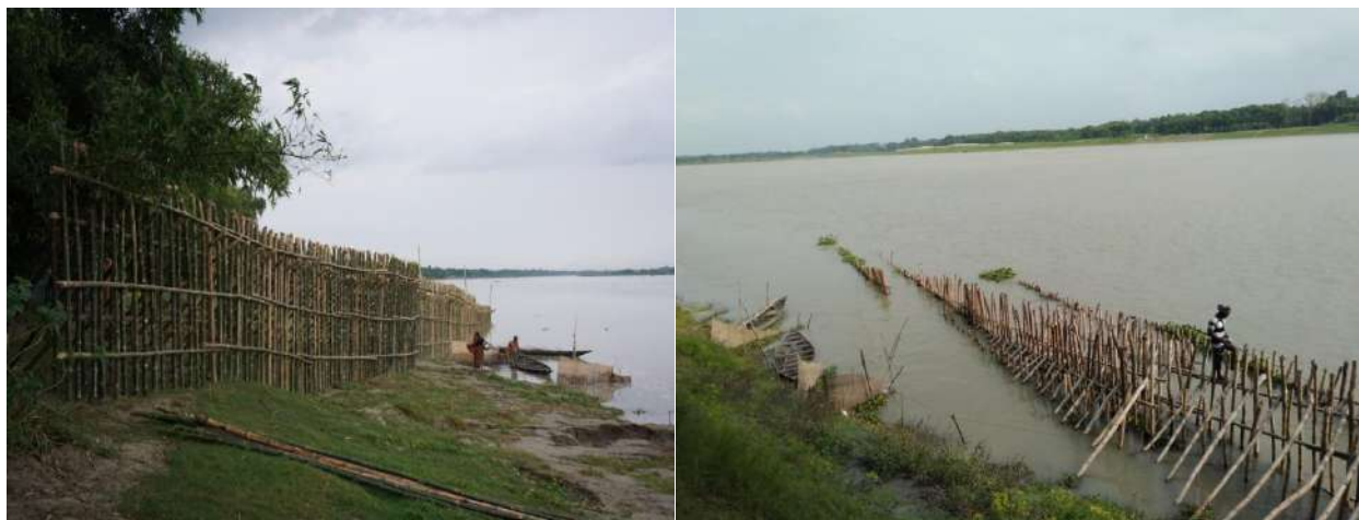
Figure 4.5 Bandal structures at u/s and d/s of Jhamshapur and Narua kheyaghat
