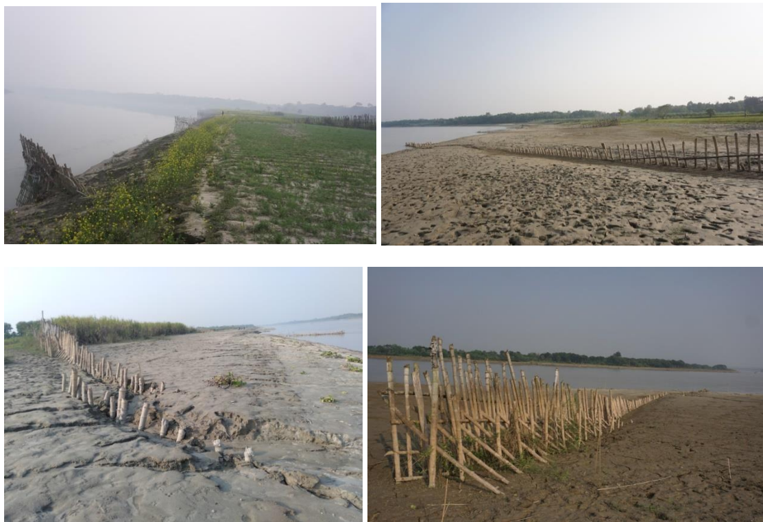
Sediment depositions on river bank induced by bandal-like structures at the right bank of Madhumati River (u/s of Kamarkhali Bridge)
