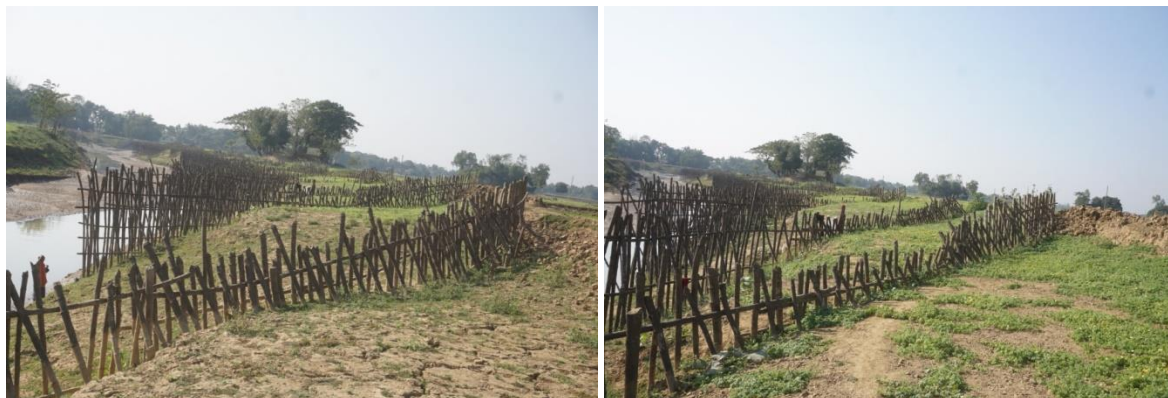
Sediment depositions on river bank induced by bandal-like structures at the Nitai River (u/s of Shankarpur Bazar, Purbadhala)
