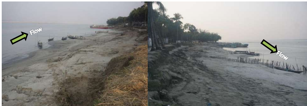
Figure 5.18 Sediment depositions on river bank induced by bandal-like structures at the right bank of Padma River (Charjoikuri)
