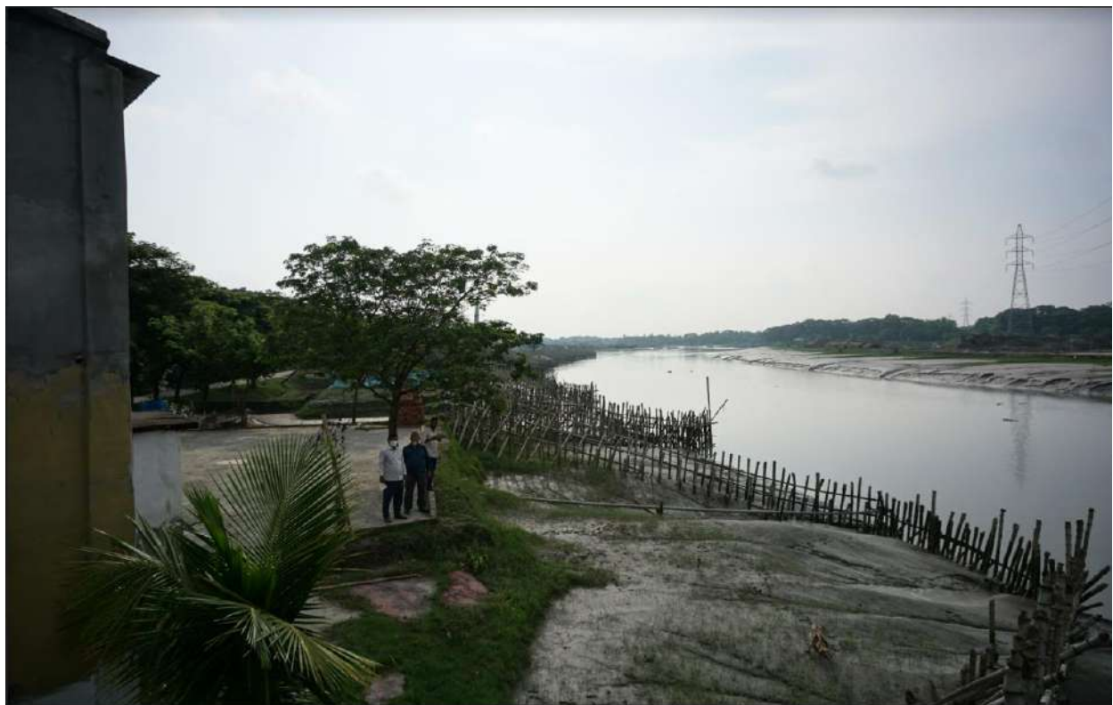
Figure 5.40 Sediment depositions on river bank induced by bandal-like structures at the Bhadra River (Kharnia Bazar, Dumuria)
