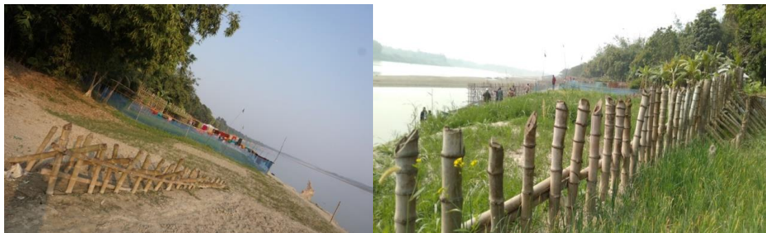
Sediment depositions on river bank induced by bandal-like structures at the left bank of Gorai River
