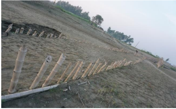
Sediment depositions on river bank induced by bandal-like structures at the left and right bank of Dhaleshwari River (Neorgacha, Chouhali)
