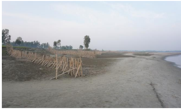
Sediment depositions on river bank induced by bandal-like structures at the left and right bank of Dhaleshwari River (Neorgacha, Chouhali)
