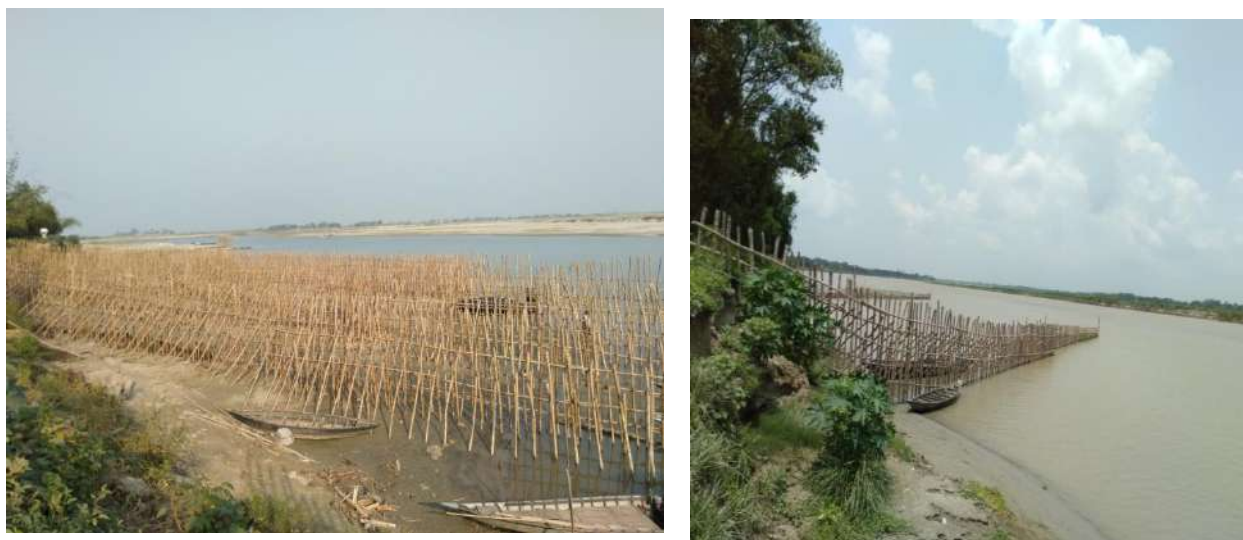
Figure 4.10 Bandal structures at u/s and d/s of Chandrapara Ghat, Sadarpur
