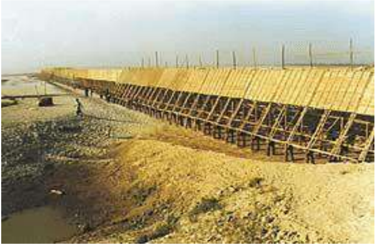
Figure 3.2 Typical bandal constructed alongside the river
