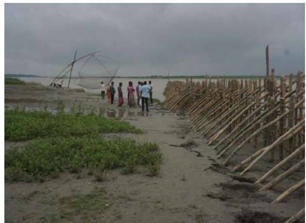
Figure 4.20 Bandal structures at Rehaipukhuria, Chouhali
