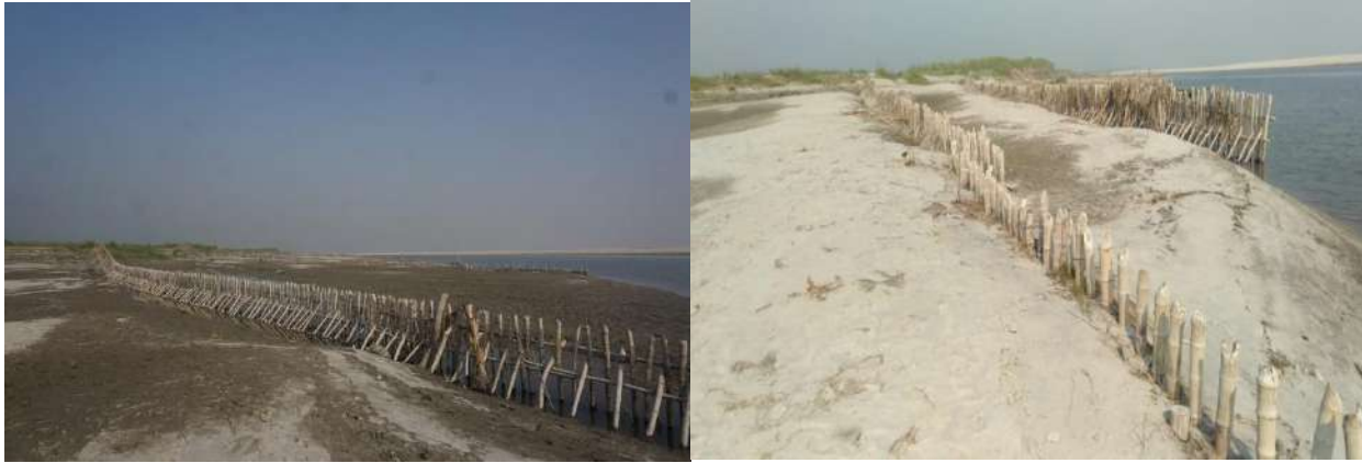
Figure 5.23 Sediment depositions on river bank induced by bandal-like structures at the right bank of Jamuna River (u/s of Cross bar-01, Sirajganj)
