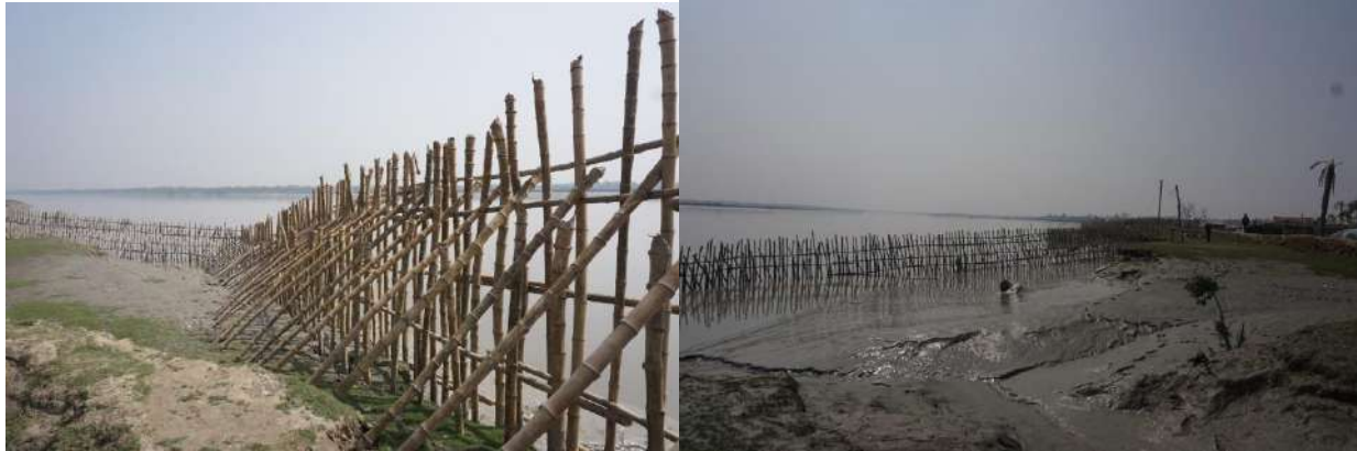
Figure 4.36 Bandal structures at Chandgoar, Dumuria, Khulna
