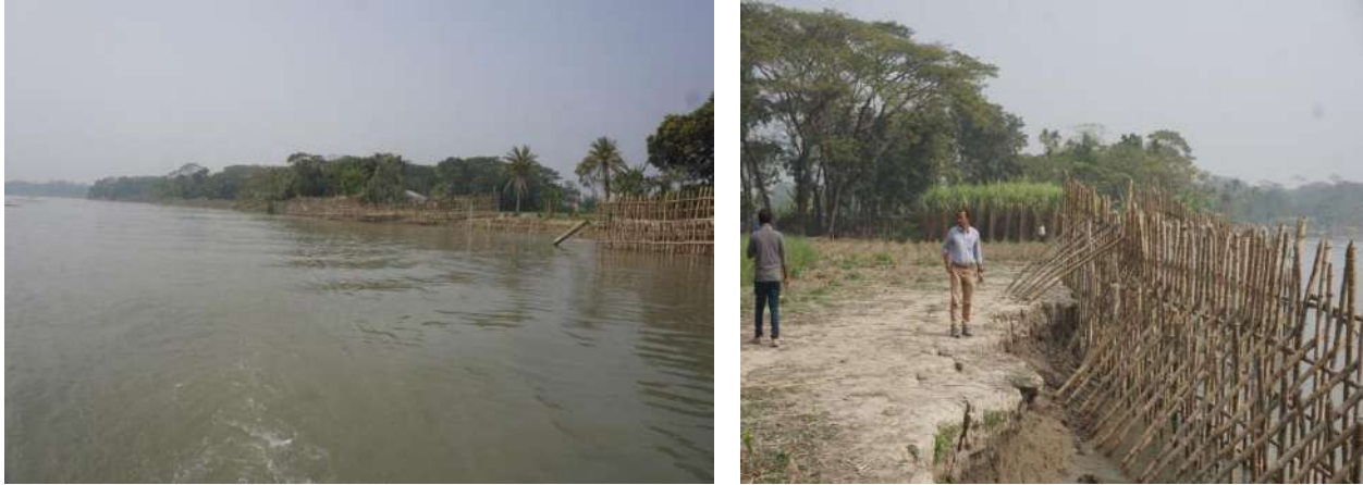
Figure 5.33 Bank erosion induced by instability of the of soil condition in Sugandha River (u/s & d/s Doarika Bridge, Babuganj)
