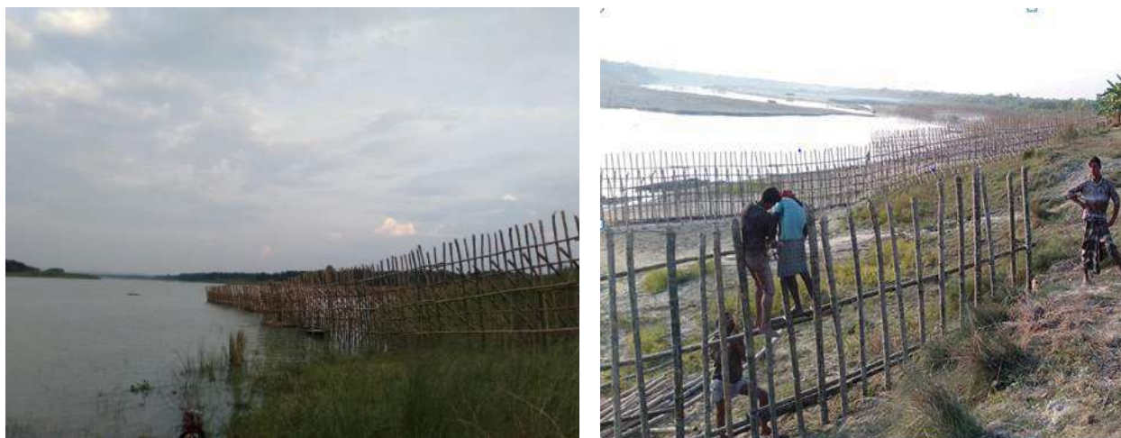
Figure 4.7 Bandal structures at u/s and d/s of Kamarkhali Bridge
