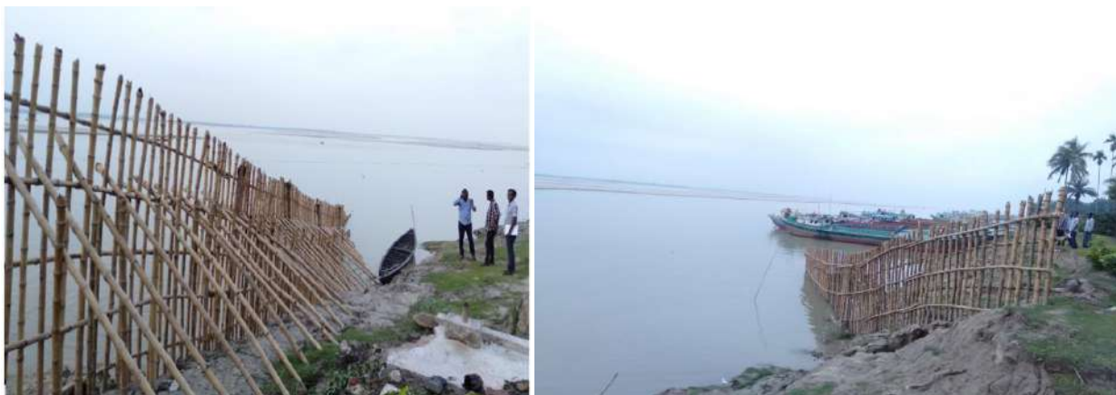
Figure 4.14 Bandal structures at Charjoikuri, Rajbari
