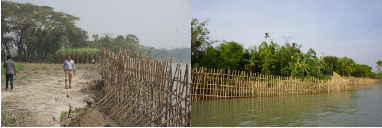
Figure 4.28 Bandal structures at u/s & d/s of Doarika Bridge, Babuganj
