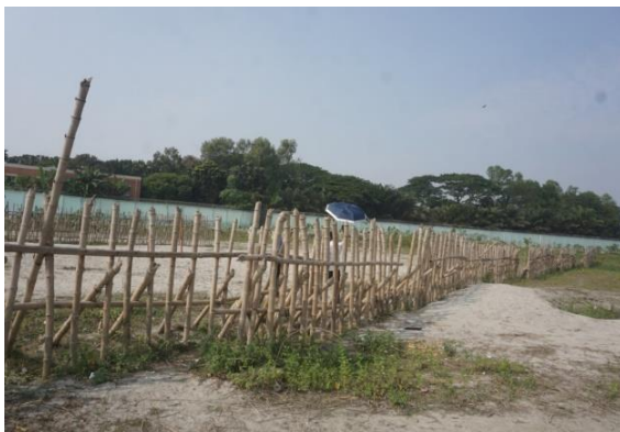
Sediment depositions on river bank induced by bandal-like structures at the right bank of Jamuna River (d/s of Enayetpur Spur)
