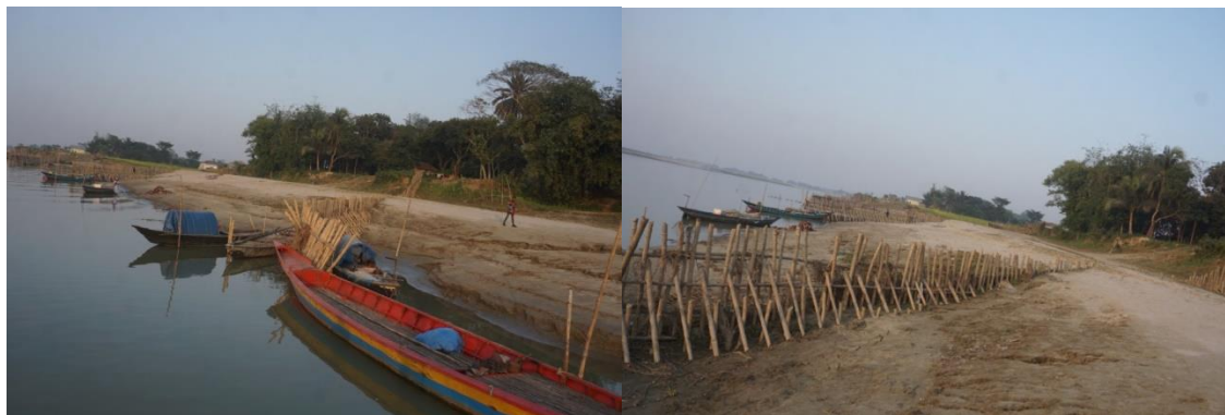
Sediment depositions on river bank induced by bandal-like structures at the right bank of Arial Khan River (d/s of Chandrapara ghat)
