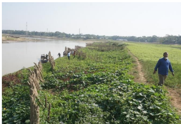
Sediment depositions on river bank induced by bandal-like structures at the right bank of Jamuna River (u/s of Cross bar-01, Sirajganj)
