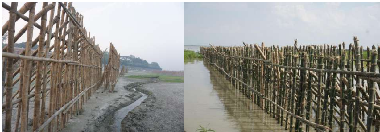
Figure 4.17 Location of the bandal structures at d/s of Enayetpur spur, Belkuchi
