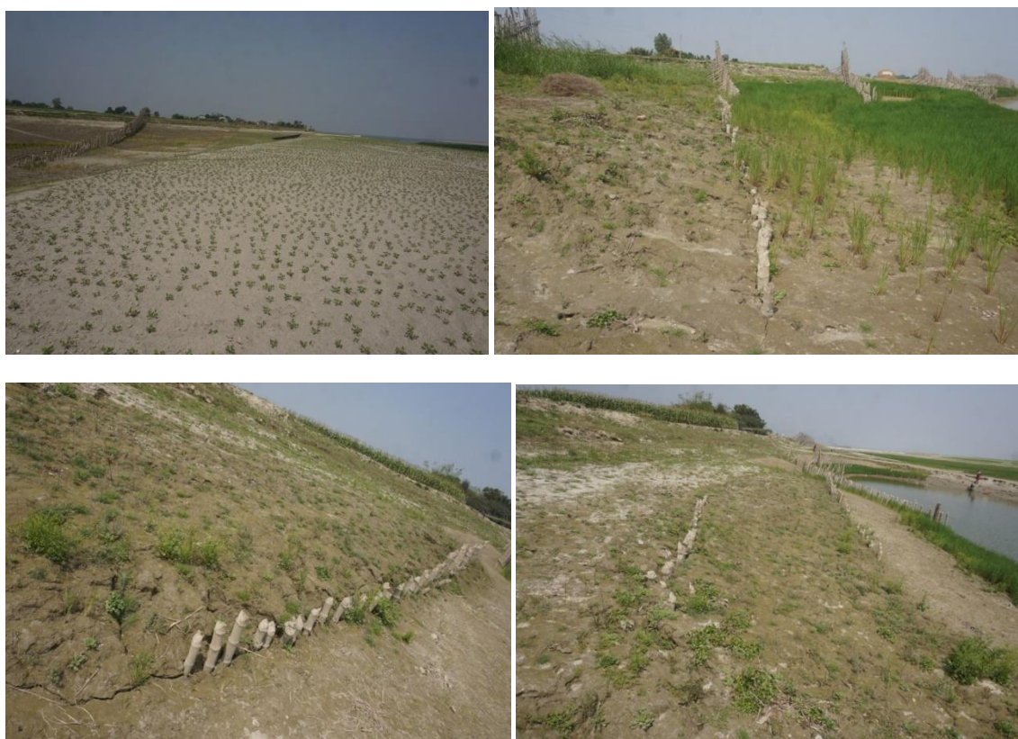
Sediment depositions on river bank induced by bandal-like structures at the right bank of Padma River (u/s of C & B ghat, Goldangirchar)
