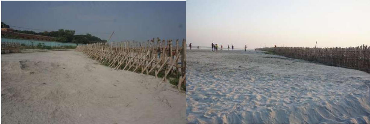
Figure 5.20 Sediment depositions on river bank induced by bandal-like structures at the right bank of Jamuna River (d/s of Enayetpur Spur)
