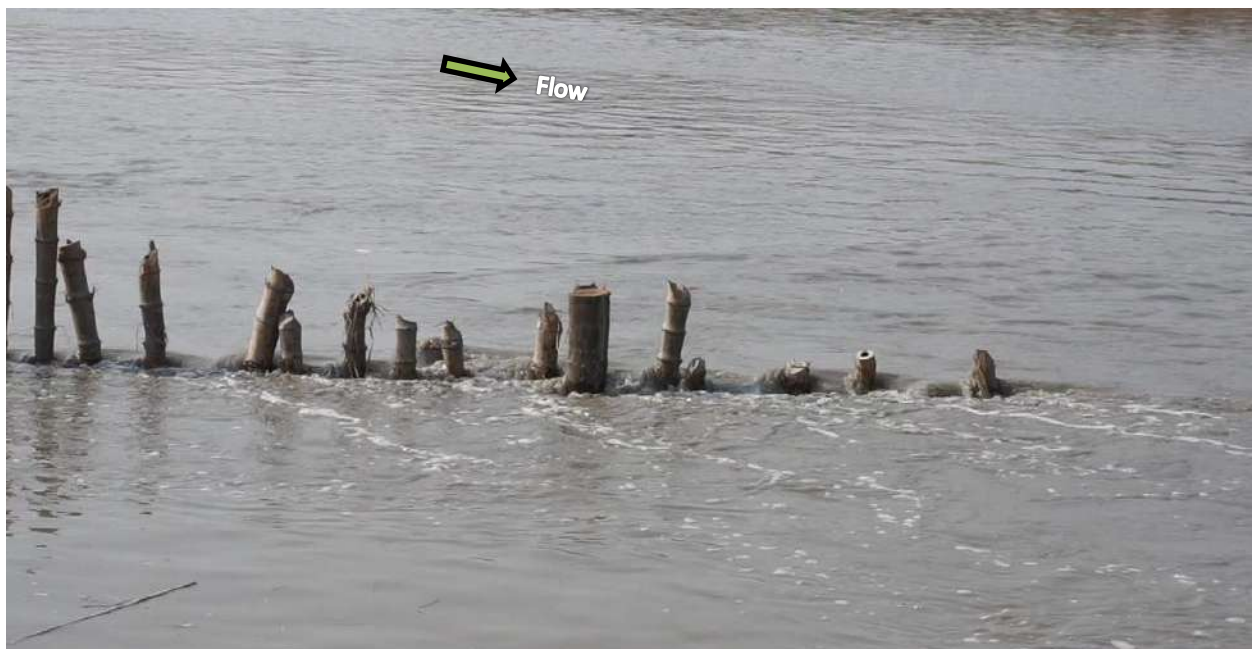
Figure 5.43 Pressure difference between the upstream and downstream side of the bandal-like structures
