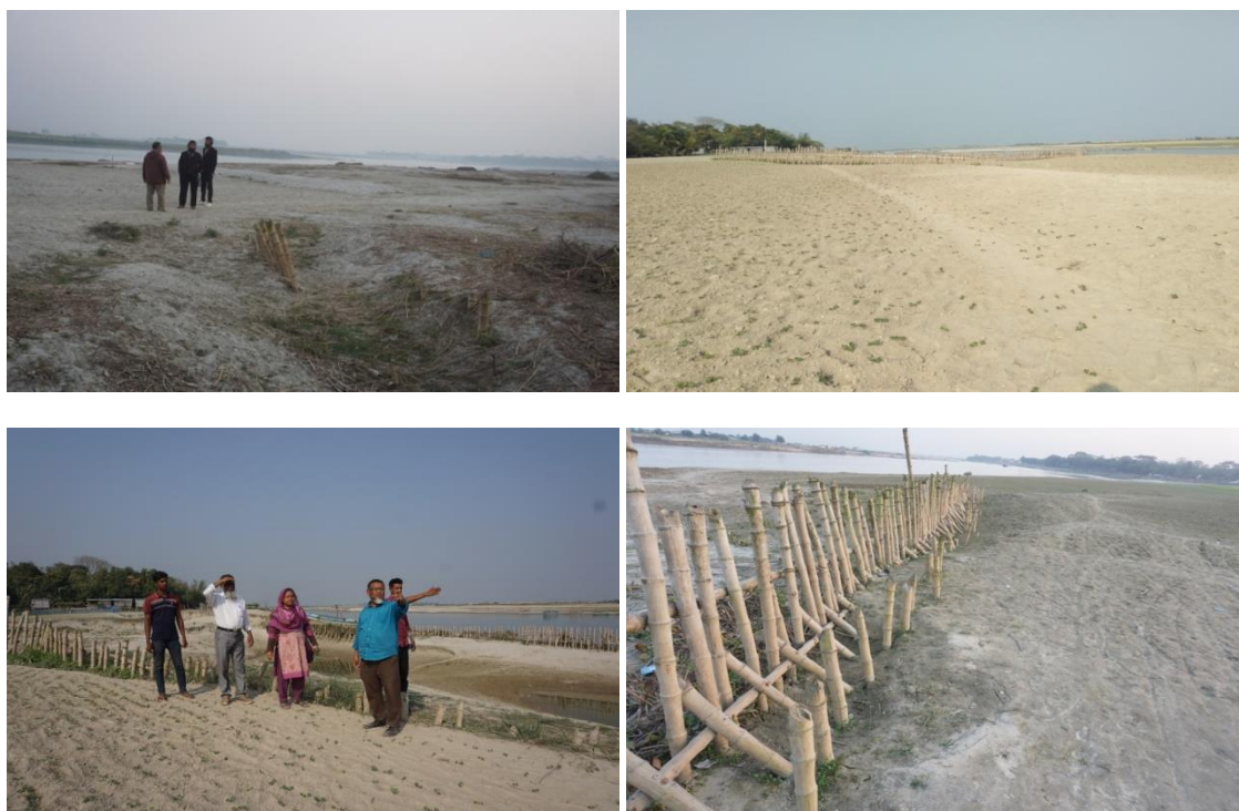
Sediment depositions on river bank induced by bandal-like structures at the right bank of Arial Khan River (u/s of Chandrapara ghat)
