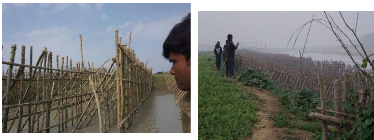
Figure 4.24 Bandal structures at Kangsa and Sumeshwari River, Purbadhala
