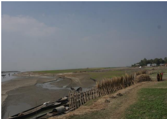
Sediment depositions on river bank induced by bandal-like structures at the left bank of Jamuna River (Rehaipukhuria, Chouhali)
