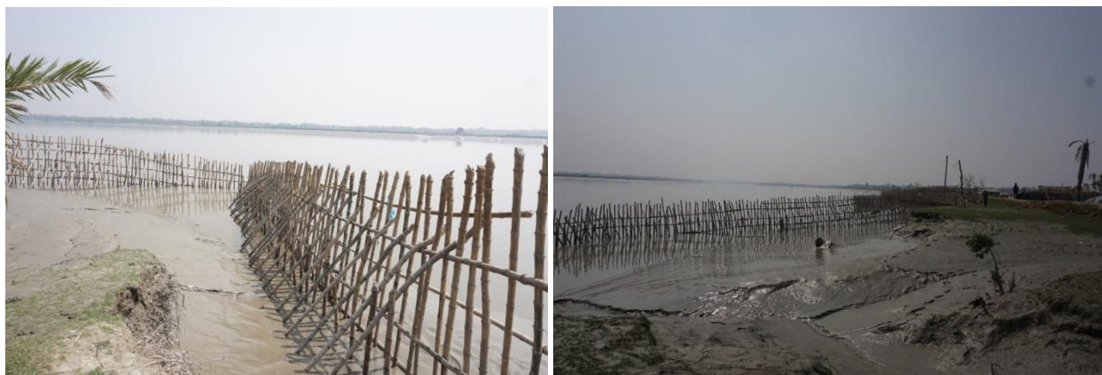
Sediment depositions on river bank induced by bandal-like structures at the Bhadra River (near Chandgoar, Dumuria)
