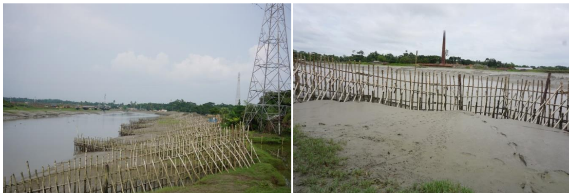
Sediment depositions on river bank induced by bandal-like structures at the Bhadra River (Kharnia Bazar, Dumuria)
