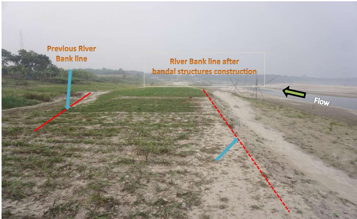
Figure 5.7 Sediment depositions on river bank induced by bandal-like structures at the left bank of Madhumati River (d/s of Kamarkhali Bridge)
