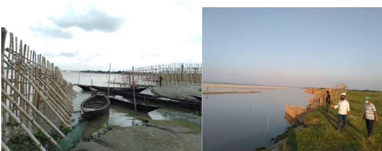
Figure 4.12 Bandal structures at Goldangirchar & Digrirchar, Faridpur
