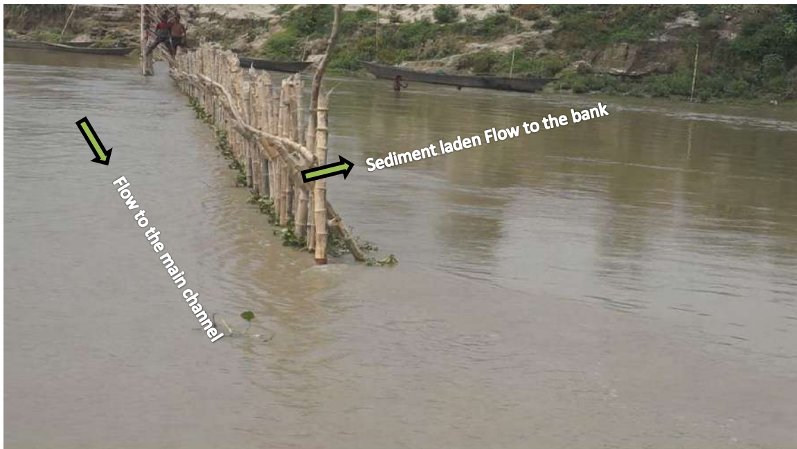
Figure 5.42 Higher flow velocity deviated to the main channel by bandal-like structures
