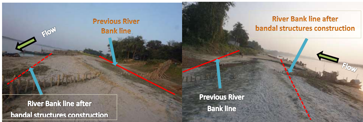
Figure 5.12 Sediment depositions on river bank induced by bandal-like structures at the right bank of Arial Khan River (d/s of Chandrapara ghat)
