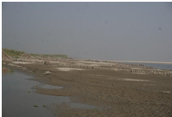
Sediment depositions on river bank induced by bandal-like structures at the right bank of Jamuna River (u/s of Cross bar-01, Sirajganj)
