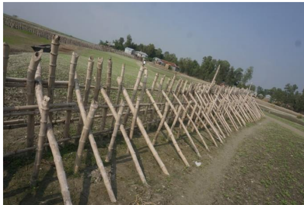
Sediment depositions on river bank induced by bandal-like structures at the left bank of Jamuna River (Rehaipukhuria, Chouhali)
