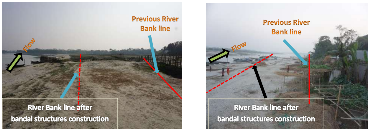
Figure 5.10 Sediment depositions on river bank induced by bandal-like structures at the right bank of Arial Khan River (u/s of Chandrapara ghat)
