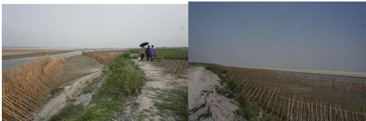
Figure 4.16 Bandal structures at u/s of Cross Bar-01, Sirajganj
