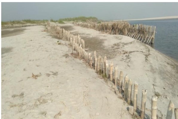
Sediment depositions on river bank induced by bandal-like structures at the right bank of Jamuna River (u/s of Cross bar-01, Sirajganj)
