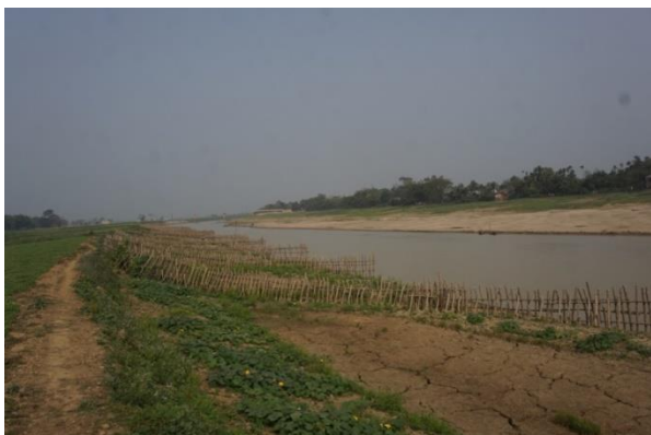
Sediment depositions on river bank induced by bandal-like structures at the right bank of Jamuna River (u/s of Cross bar-01, Sirajganj)
