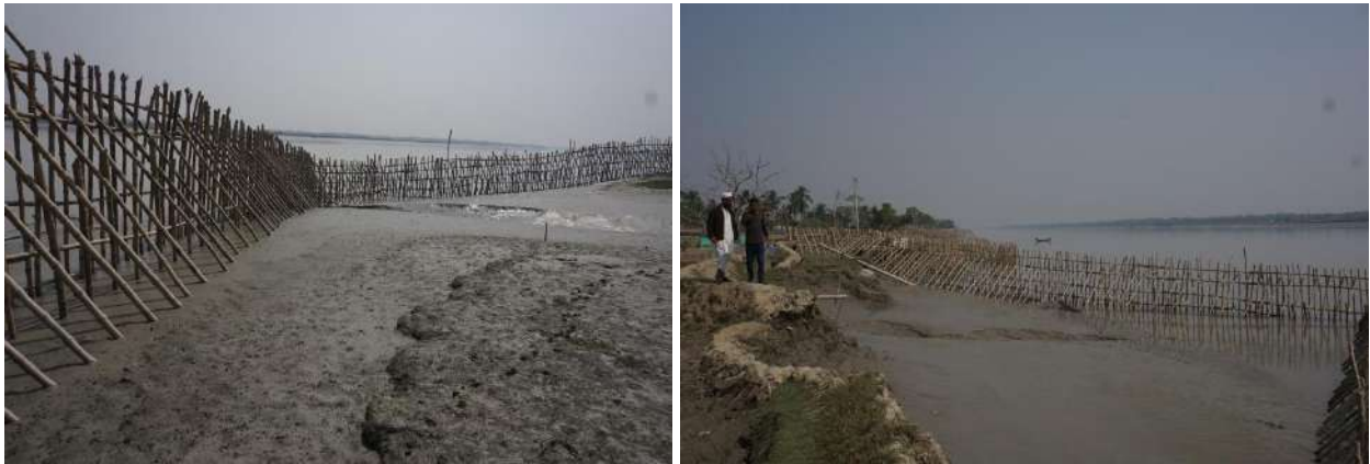
Figure 5.37 Sediment depositions on river bank induced by bandal-like structures at the Bhadra River (near Chandgoar, Dumuria)
