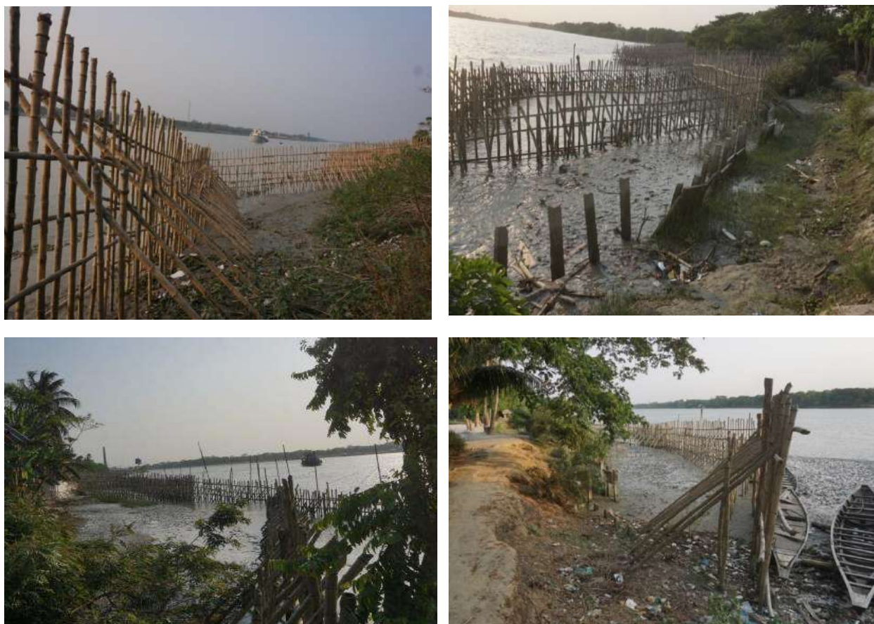
Figure 5.35 Sediment depositions on river bank induced by bandal-like structures at the Rupsha-Atai Rivers
