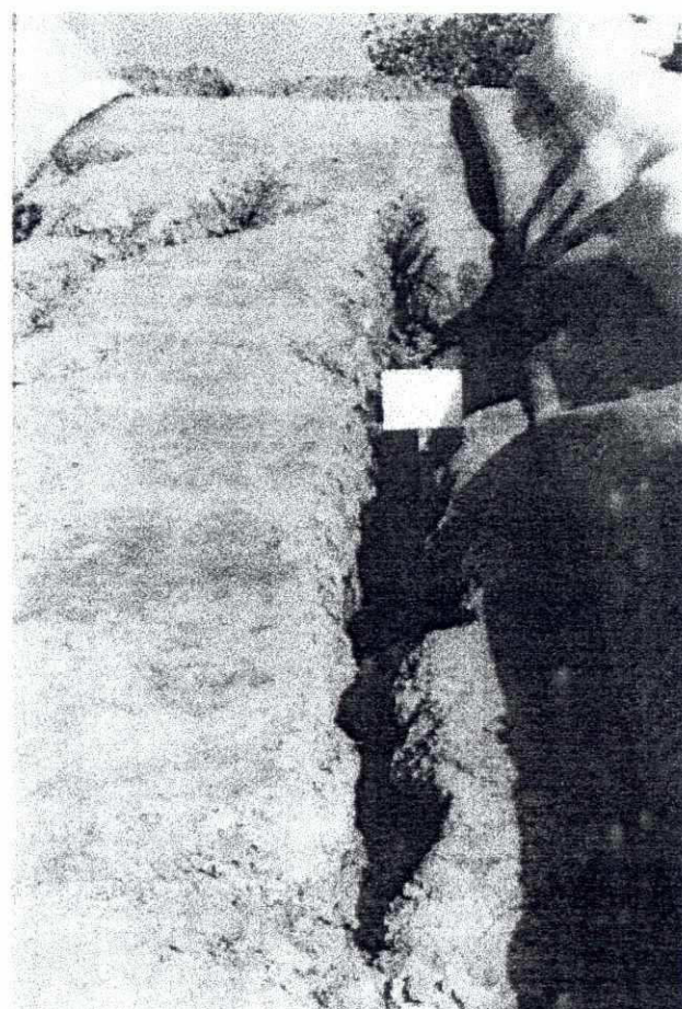
Both pictures: Sight on rain-cuts Section E-2 (19.02.1998)
