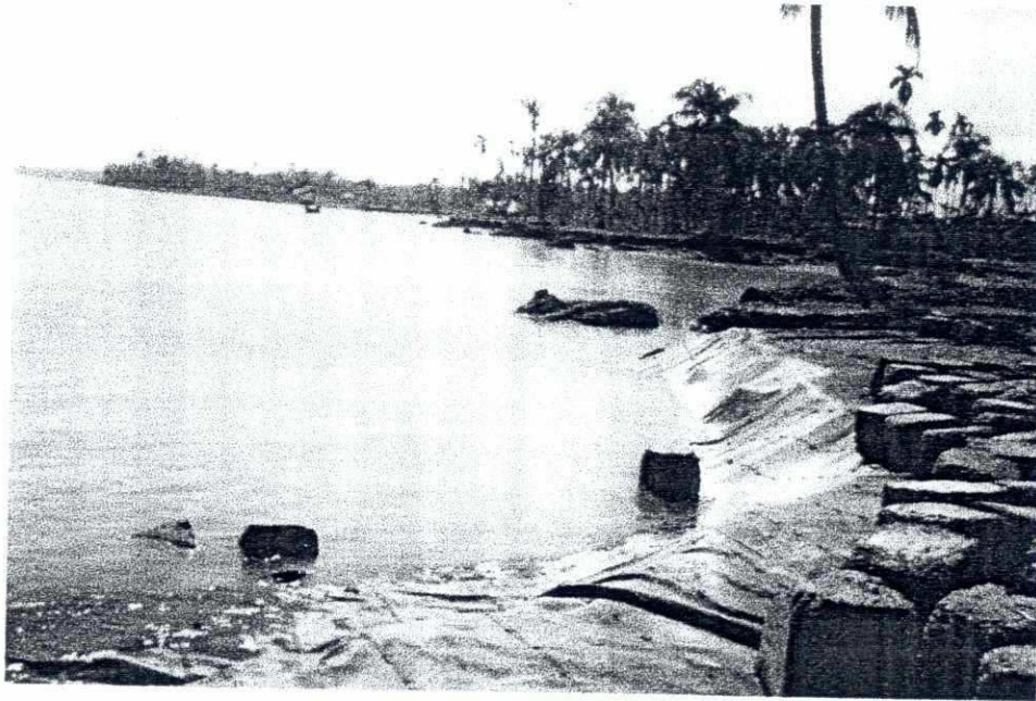
Picture 13 During the flood erosion attacked the downstream side of KC-3.
