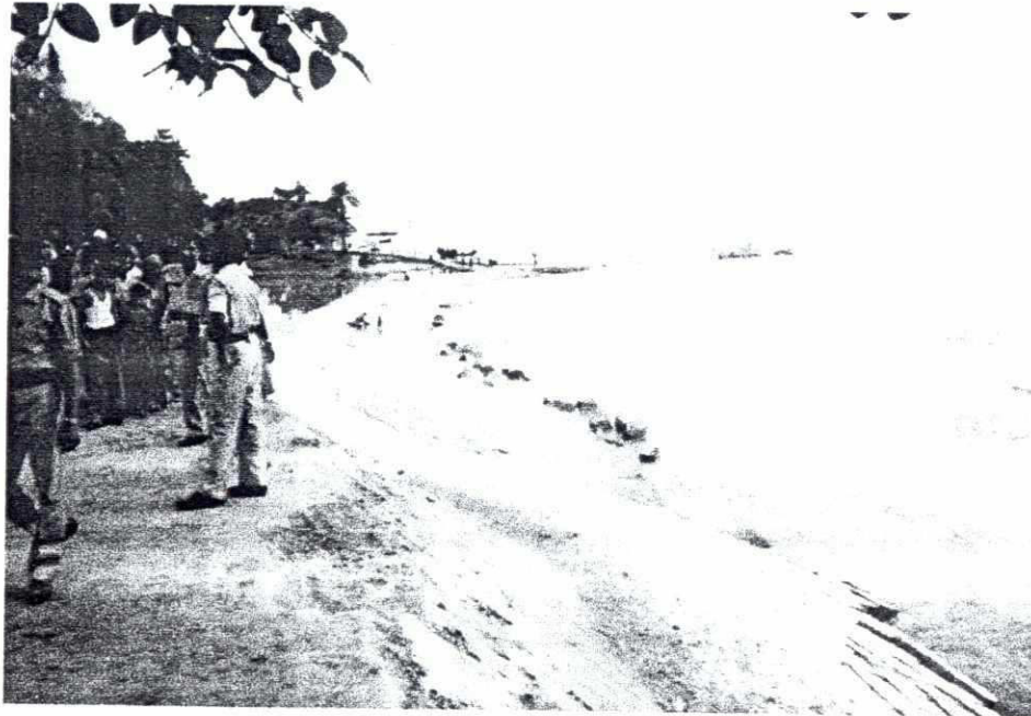
Picture 4 Block pitching performed by the Chadpur BWDB near the downstream spur
