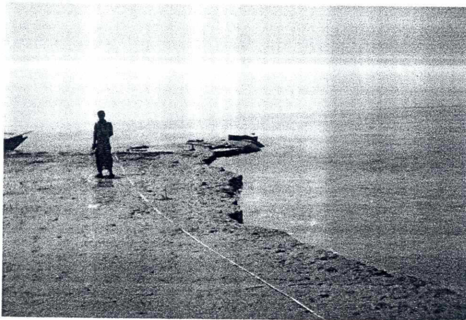
Picture 9 During the flood the downstream spur has disappeared at Haimchar.
