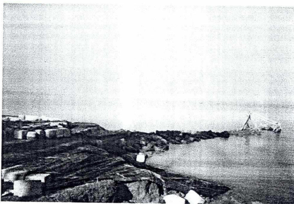
Picture 12 After being hit by a river vessel the downstream spur has tilted.
