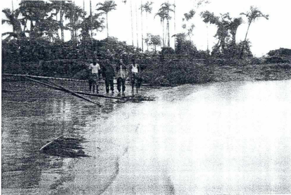
Picture 15 Siltation pattern at the upstream side of the middle spur (KC-2)
