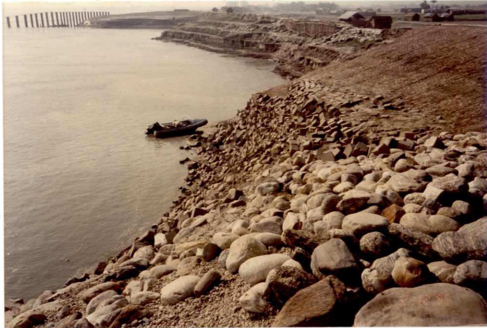
Photo 21: Groyne G-2 on 02.12.1995; view from groyne toward (d/s) main damage to embankment (water level at 15.79 m PWD)
