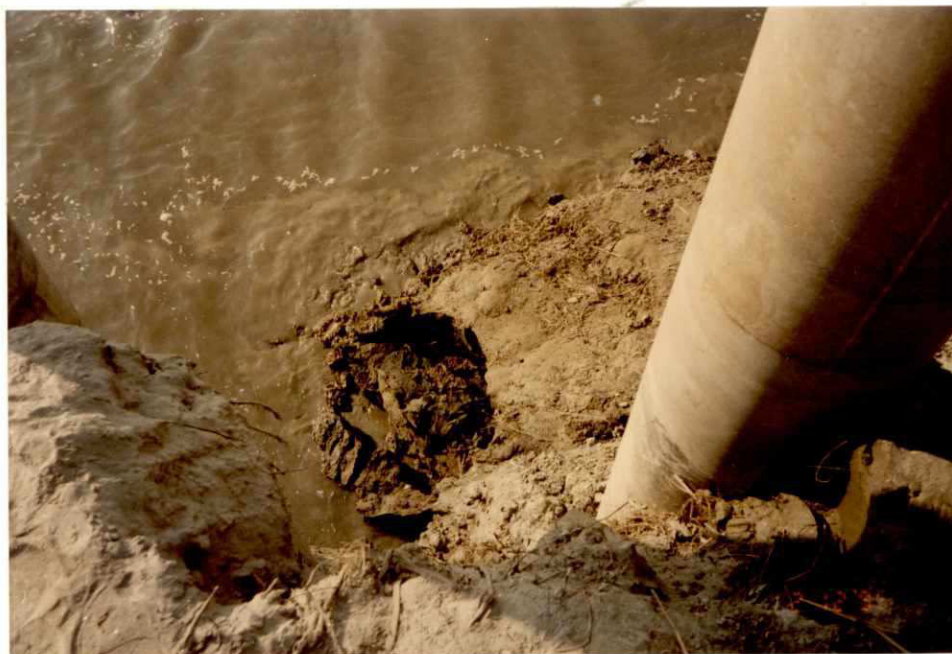
Photo 5: Groyne G-A on 02.12.1995; erosion process around spun cc-piles (water level at 15.79 m PWD)
