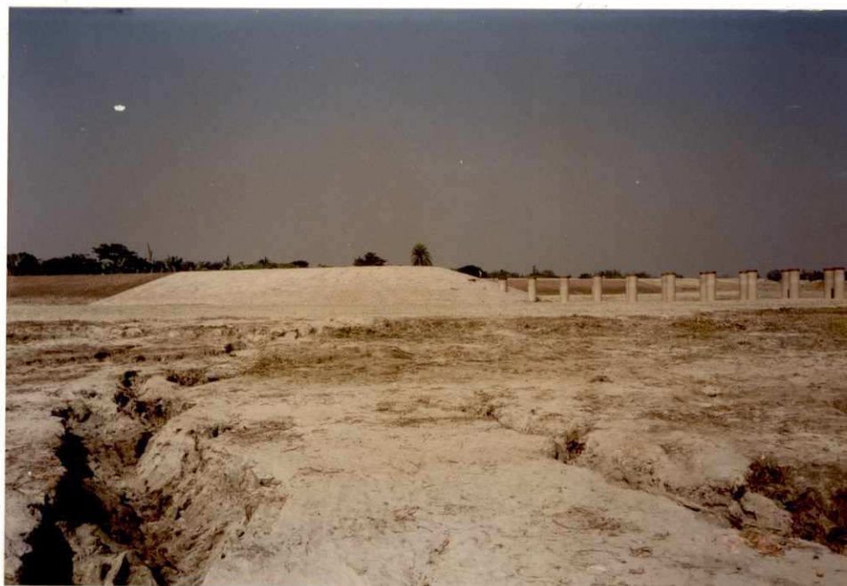
Photo 32: Groyne G-B/1 on 03.12.1995; Impermeable groyne without any damage
