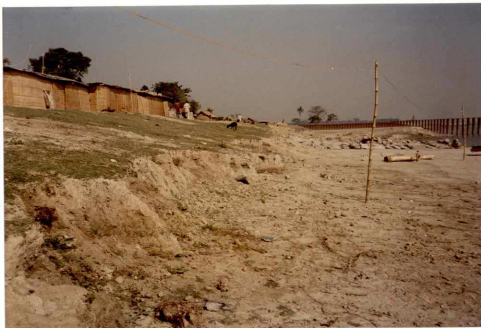
Photo 25: Groyne G-1 on 03.12.1995; main embankment eroded by waves (Durba grass planted too late to develop proper rooting) (water level at 15.75 m PWD)
