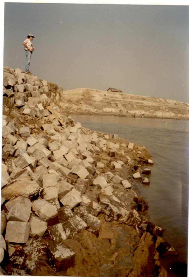
Photo 17: Groyne G-3 on 02.12.1995; (u/s side) scattered cc-blocks of falling apron (protection to impermeable groyne head) (water level at 15.79 m PWD)
