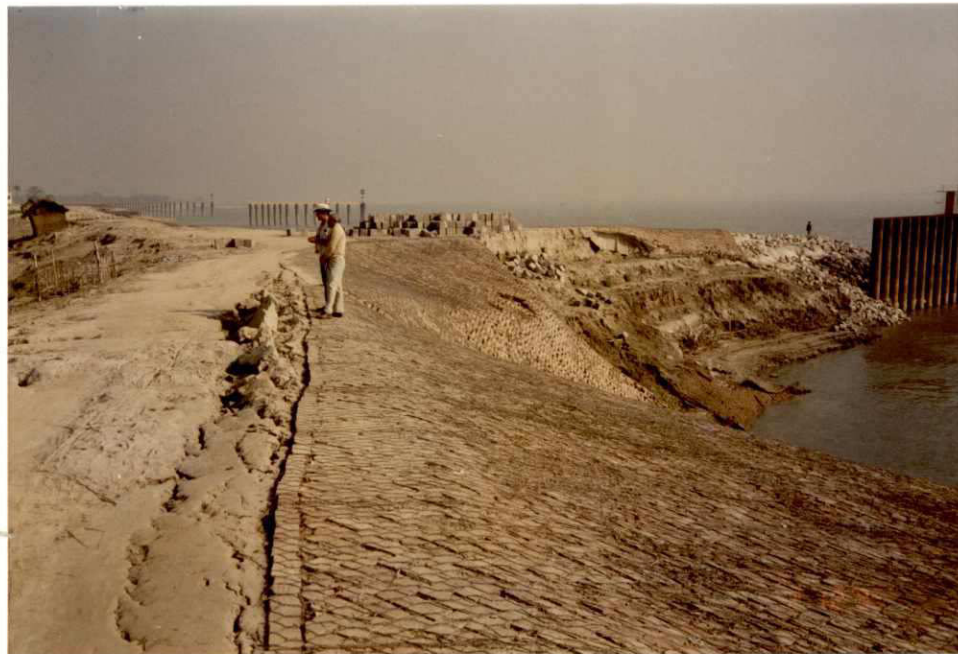
Photo 11: Groyne G-3 on 02.12.95; Anchorage of brick mattress effected by major slide but yet functional (water level at 15.79 m PWD)
