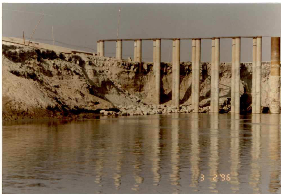
Photo 6: Groyne G-A on 03.02.1996; eroding bank reached d/s edge of cofferdam. Falling apron around cofferdam head completely unfunctional (water level at 14.48 m PWD)
