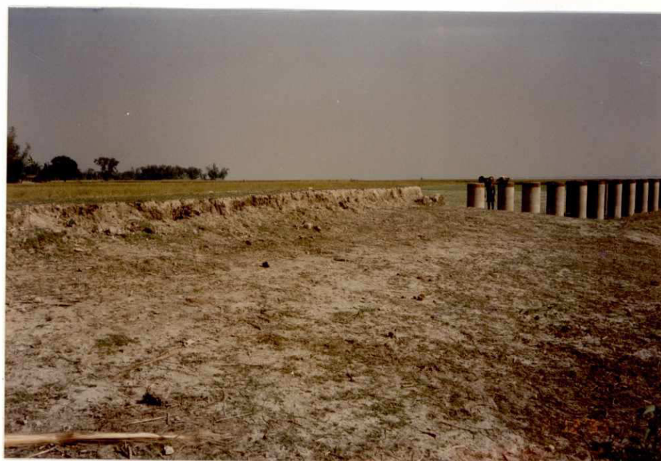
Photo 33: Groyne G-B/2 on 03.12.1995; Impermeable groyne; earthdam and Durba grass cover; downstream side eroded (Durba grass sods planted too late)
