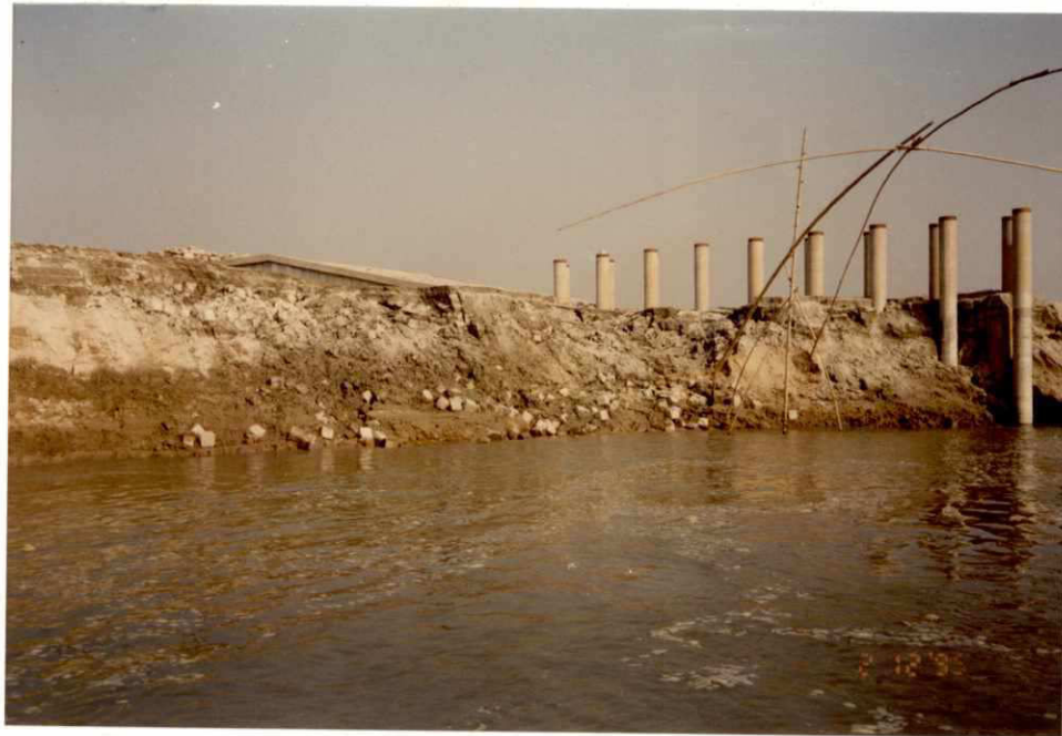
Photo 3: Groyne G-A on 02.12.1995; bank erosion reached d/s edge of cofferdam (water level at 15.79 m PWD)
