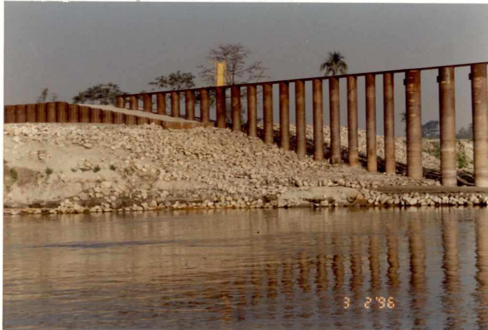
Photo 27: Groyne G-1 on 03.02.1996; view from d/s side; slope protection functional (water level at 14.48 m PWD)
