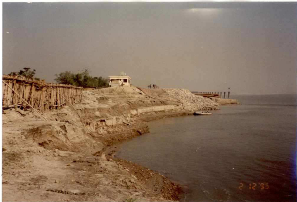
Photo 20: Groyne G-2 on 02.12.1995; Temporary cofferdam approx. 80 m downstream from G-2 as closure for breached main embankment (water level at 15.79 m PWD)
