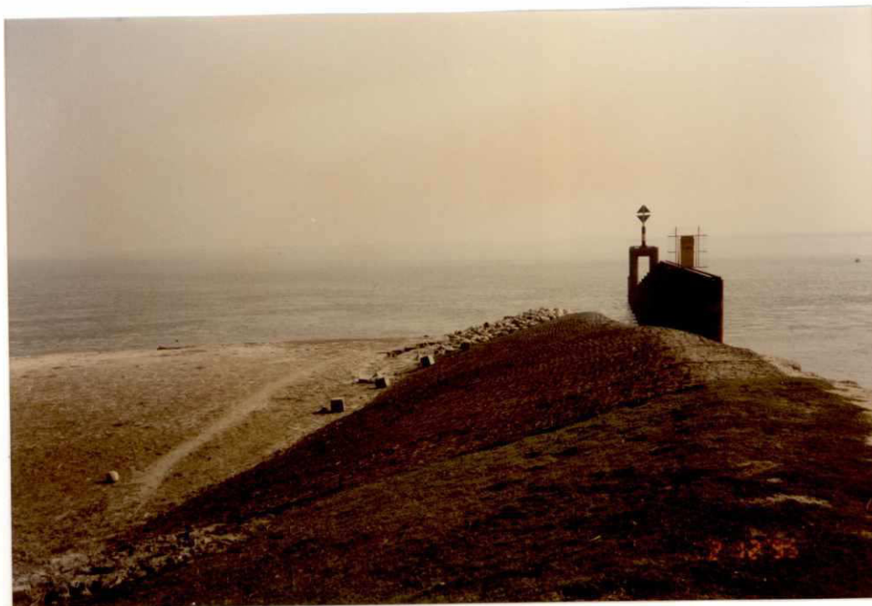
Photo 14: Groyne G-3 on 02.12.1995; View along impermeable part of G-3; upstream portion yet fully in tact (water level at 15.79 m PWD)
