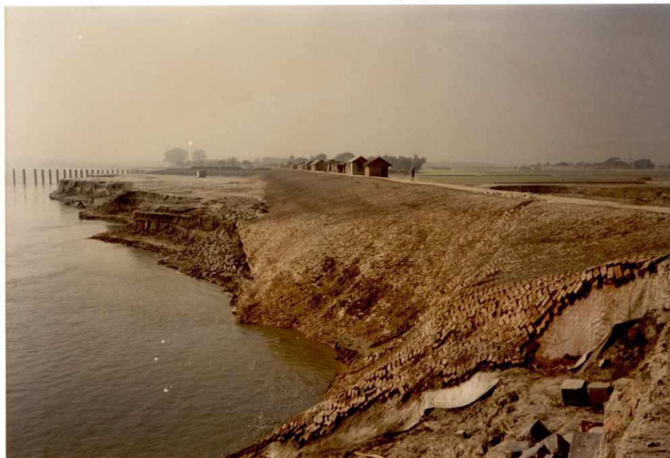
Photo 13: Groyne G-3 on 02.12.1995; Damaged main embankment d/s from G-3 (water level at 15.79 m PWD)
