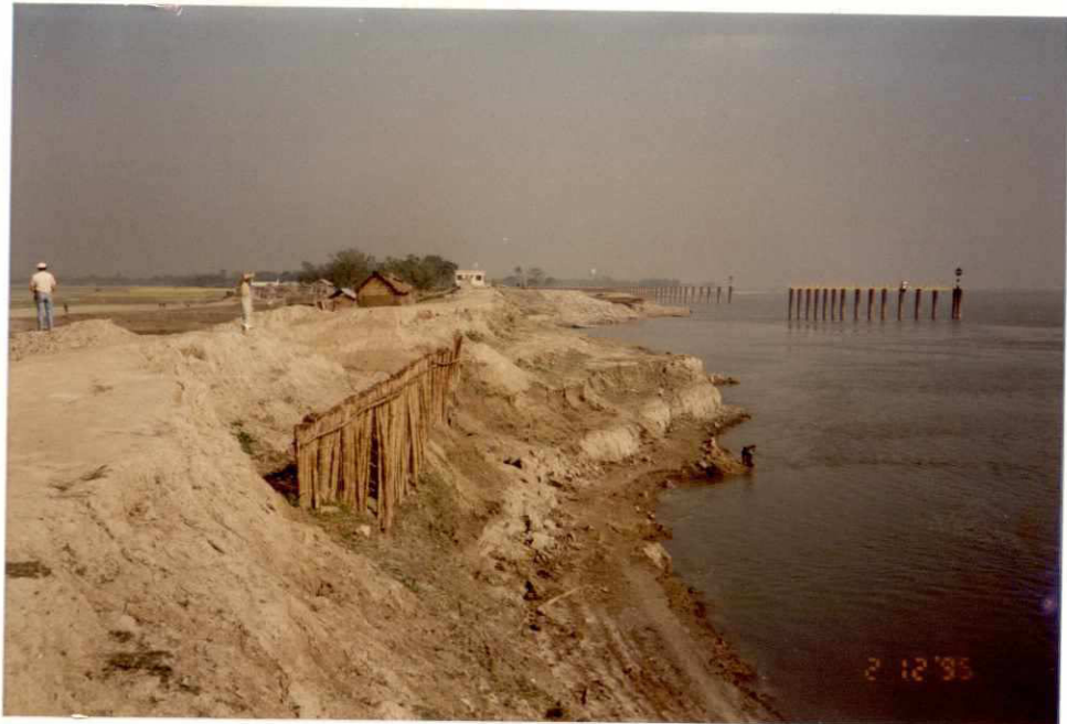
Photo 19: Groyne G-2 on 02.12.1995; Damaged main embankment (water level at 15.79 m PWD)
