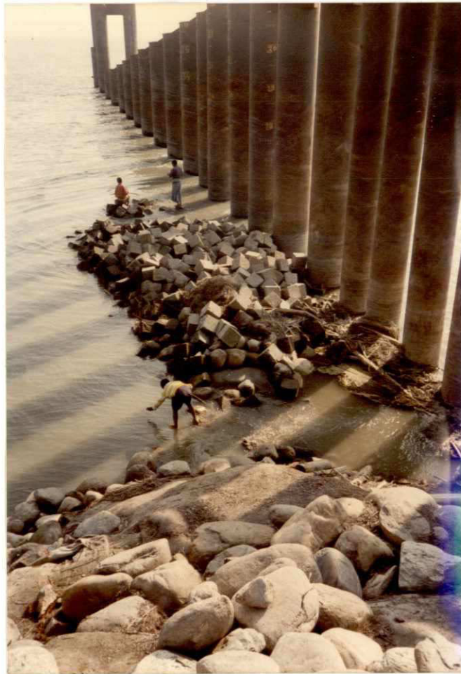
Photo 15: Groyne G-3 on 02.12.1995; falling apron of u/s impermeable groyne head; stone dumping along piles likely to be excessive dumping during construction (water level at 15.79 m PWD)
