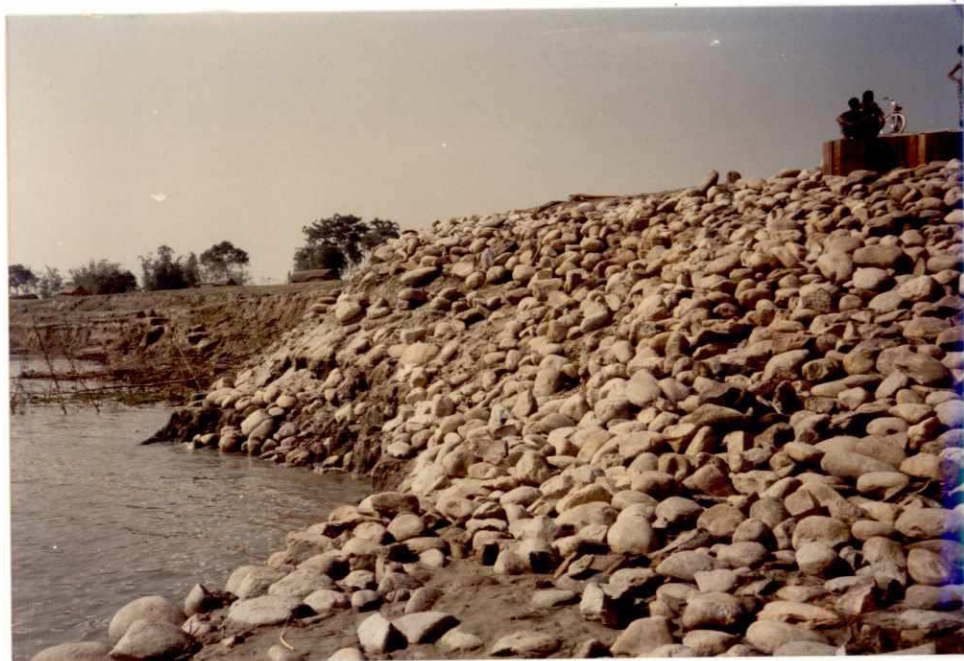
Photo 28: Groyne G-1 on 03.12.1995; slope deformation, rip-rap on granular filter layer (water level at 15.75 m PWD)
