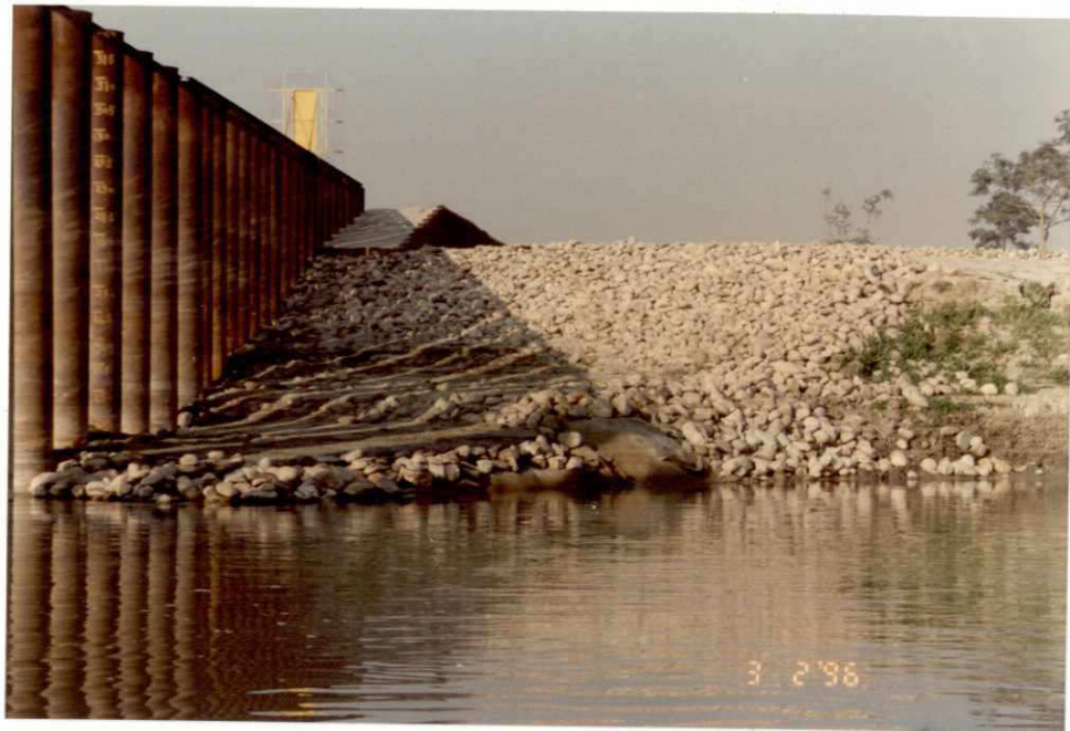
Photo 29: Groyne G-1 on 03.02.1996; View from u/s side; slope protection in tact; Geo-jute-sand mat partly exposed within bed protection around the piles (water level at 14.48 m PWD)
