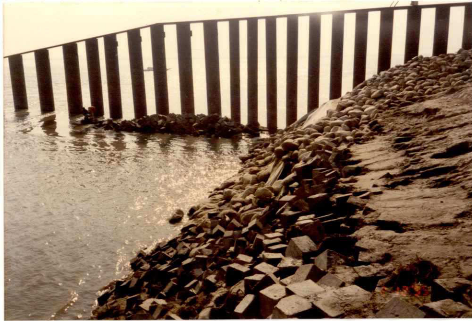
Photo 15: Groyne G-3 on 02.12.1995; falling apron of u/s impermeable groyne head; stone dumping along piles likely to be excessive dumping during construction (water level at 15.79 m PWD)
