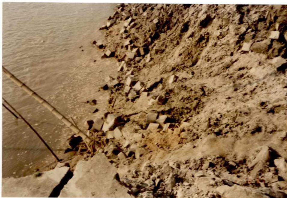
Photo 4: Groyne G-A on 02.12.1995; Falling apron near d/s edge of cofferdam (water level at 15.79 m PWD)
