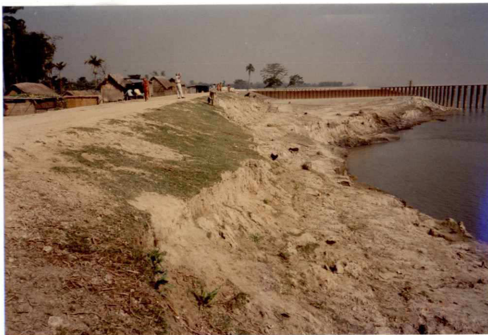
Photo 26: Groyne G-1 on 03.12.1995; main embankment eroded by waves and return current (water level at 15.75 m PWD)
