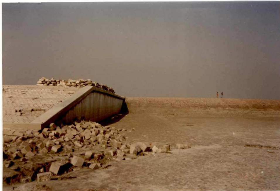
Photo 8: Groyne G-A on 02.12.1995; view along u/s side of cofferdam, no damages (water level at 15.79 m PWD)
