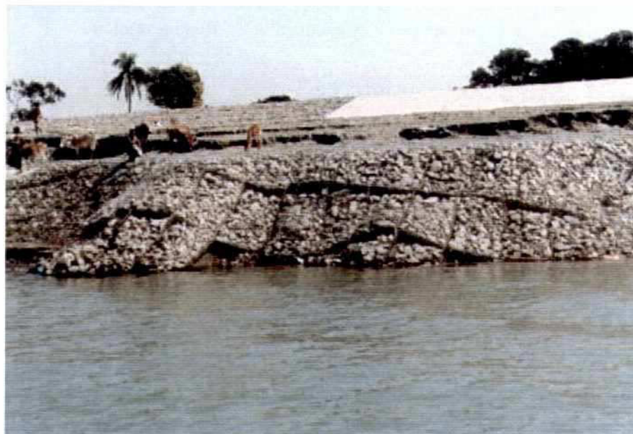
Photo 5.2-1: Section C: Launching apron on February 18, 1998; Water level at 13.00 m+PWD
