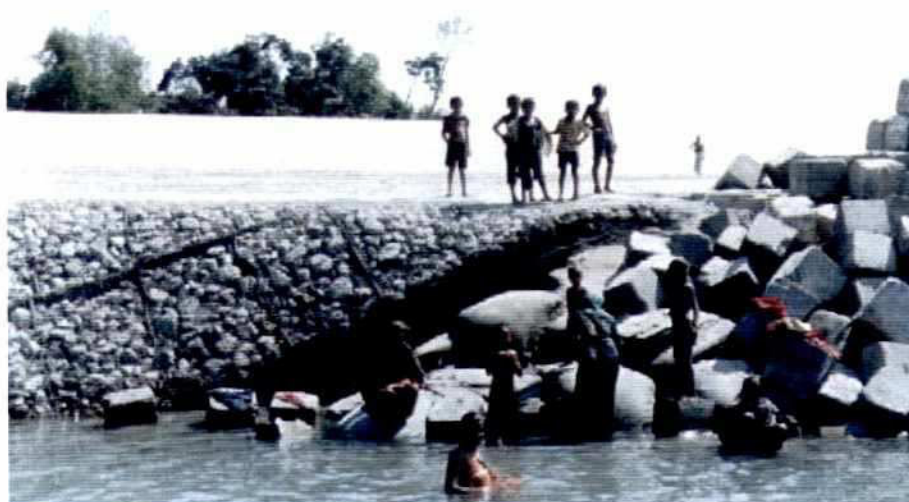
Photo 5.2-2: Transition Section C/D on February 18, 1998; Section C: Launching apron; Section D: Falling apron; Water level at 13.00 m+PWD
