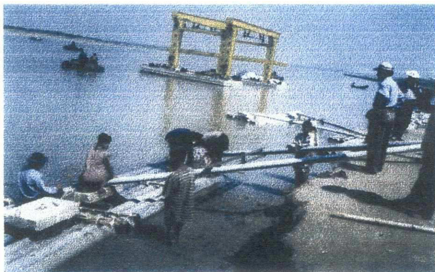
Picture 4 Transport of foundation slabs and A-frames to the THP
