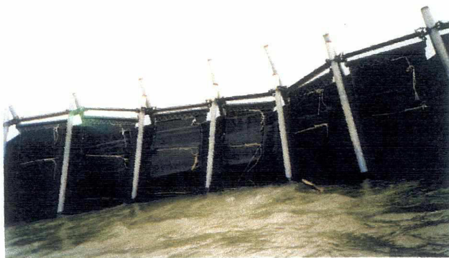
Tilted A-frames after spring tide
