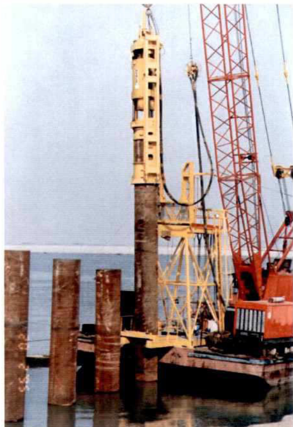
Photo 7.11-11: Piling of Steel Piles dia 1016 mm and 1220 mm by Hydraulic Hammer Menck MHF 10-15
