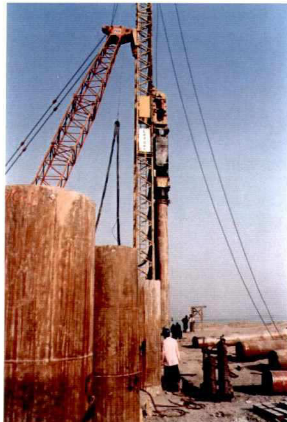
Photo 7.11-4: On-shore Piling of Steel Pile dia 711 mm; Piling rig Kobe 22
