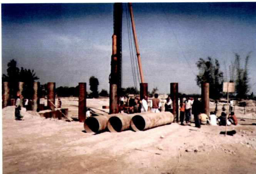
Photo 7.11-1: On-shore Piling of Steel Pile dia 711 mm; Piling rig Kobe 22
