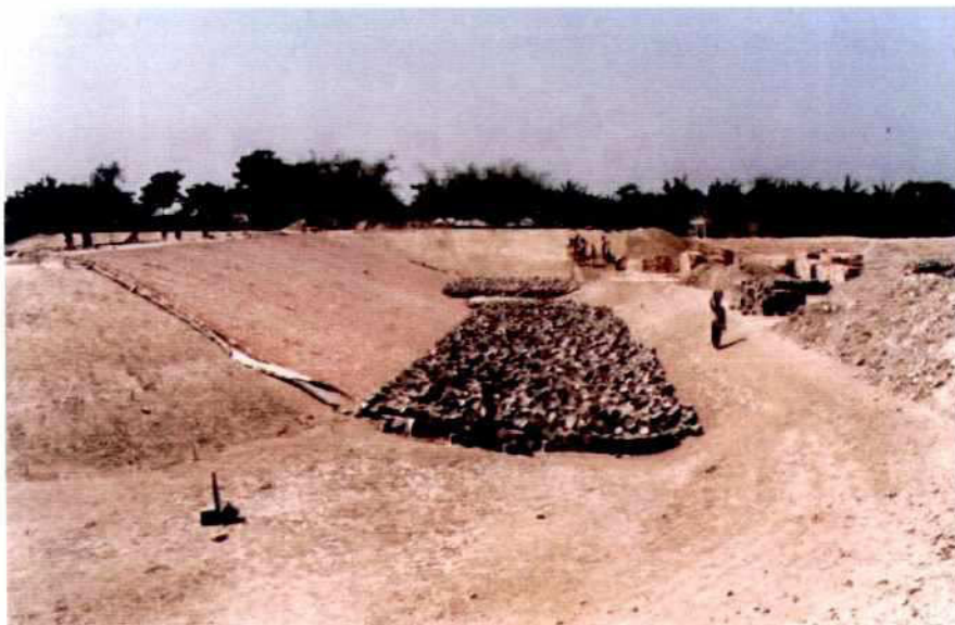
Photo 7.7-6: Brick-Mattress on Geotextile Filter Mat at Groyne G-B1
