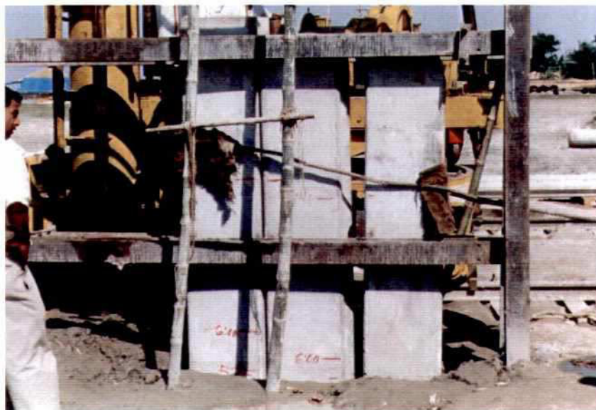
Photo 7.13-6: Concrete Sheet Pile Guide Frame
