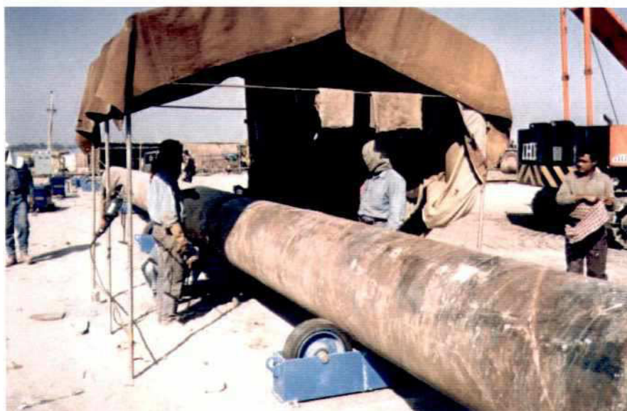
Photo 7.10-2: Pile Welding Roller Bed
