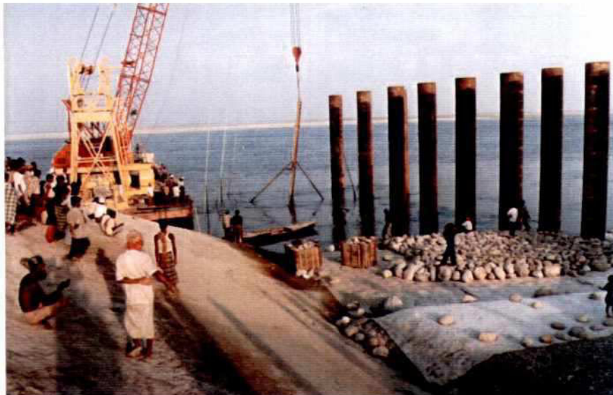
Photo 7.9-4: Groyne G-1, Bed Protection, manually laid Boulders on Geotextile Filter Mat
