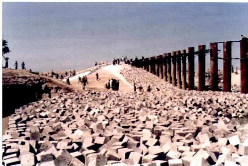
Photo 7.9-6: Groyne G-2, Bed Protection, dumped CC-Blocks (without filter layer)
