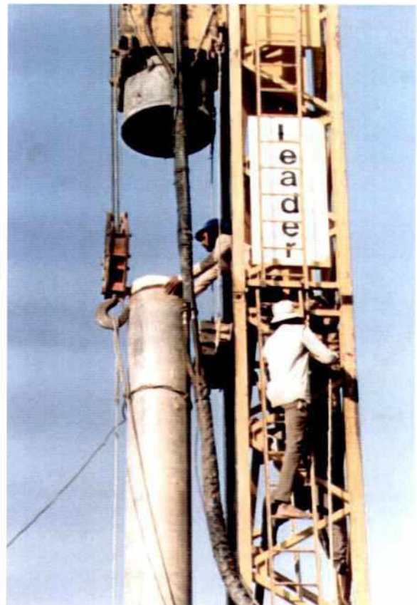
Photo 7.12-4: Piling pre-cast Concrete Spun Piles, Piling Rig, Hydraulic BSP Hammer; Detail: Fixing of Special Pile Head Cushion
