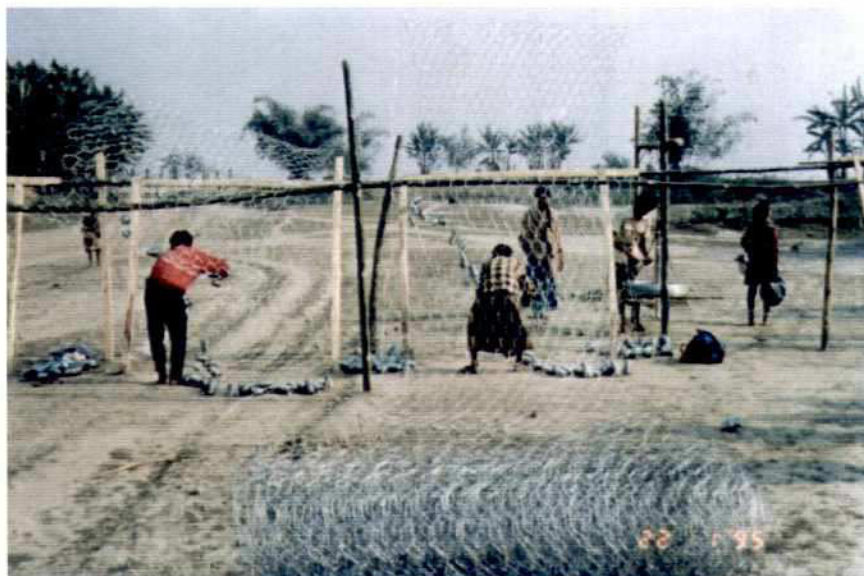
Photo 4.1-6: Production of Wiremesh at site
