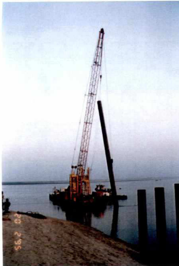
Photo 7.11-7: Pile lifting
