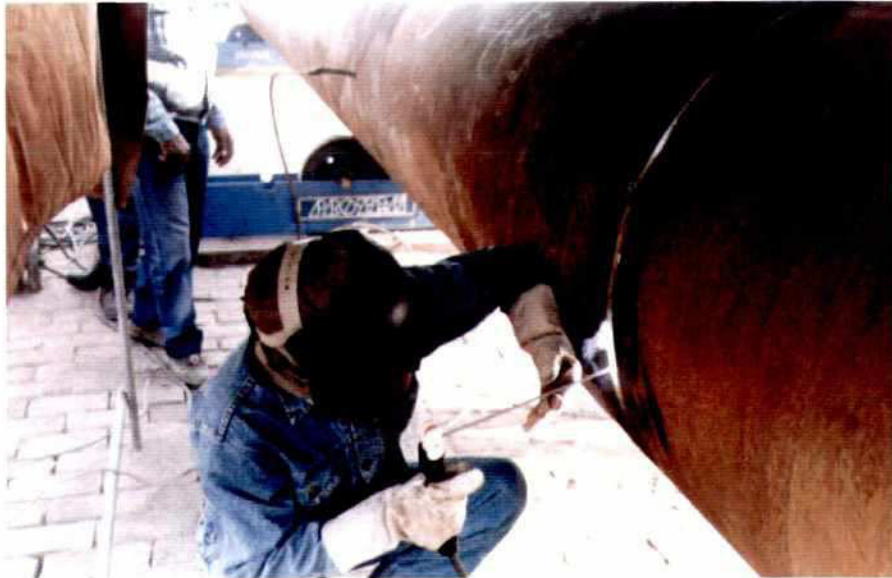
Photo 7.10-3: Vertical upwards Welding on Roller Bed
