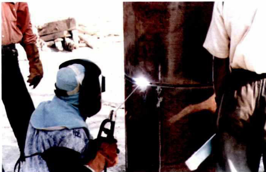
Photo 7.10-4: Horizontal Welding "In-Situ Pile Joints"
