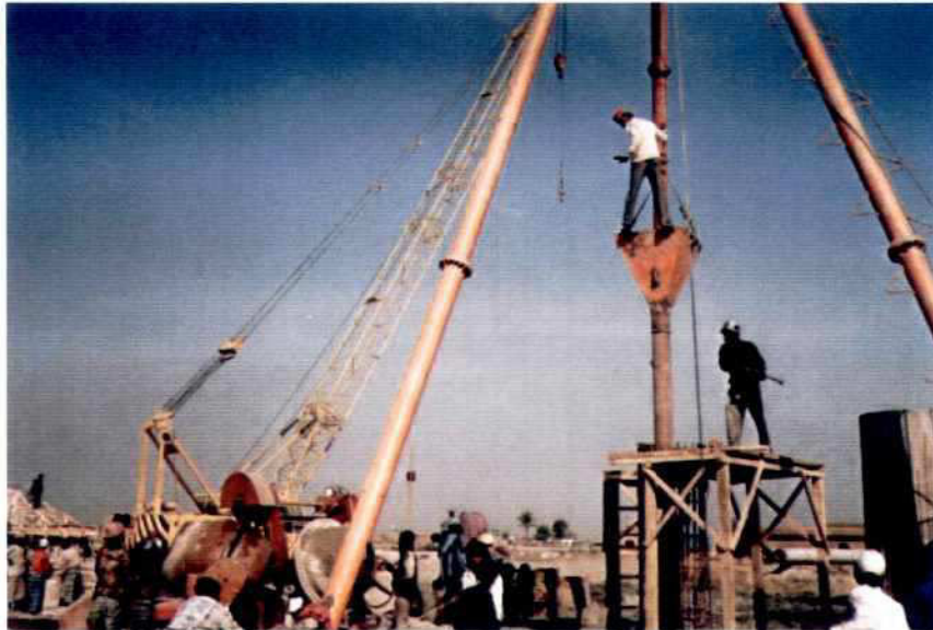
Photo 7.14-3: Concreting of In-Situ Bored Piles, under Water Method
