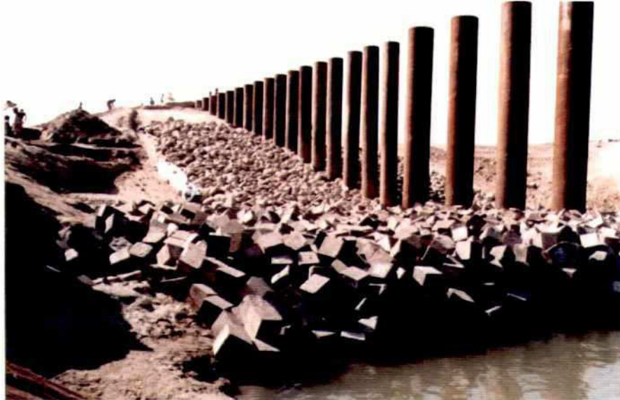
Photo 7.9-5: Groyne G-2, Bed Protection, dumped CC-Blocks (without filter layer)
