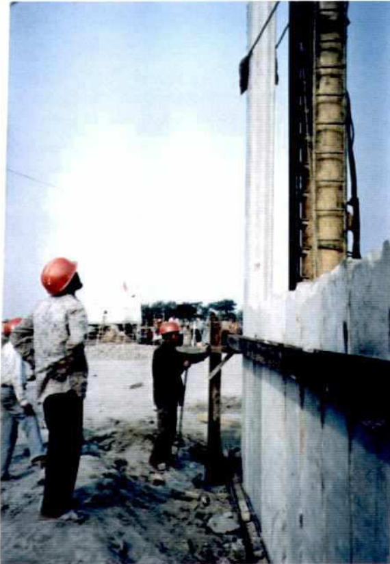
Photo 7.13-5: Concrete Sheet Pile Guide Frame
