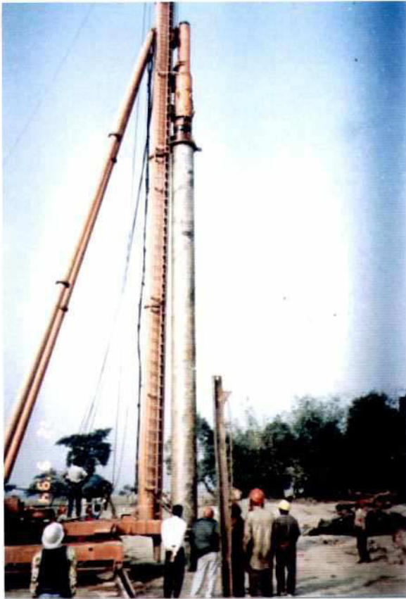
Photo 7.12-1: Piling pre-cast Concrete Spun Piles, Piling Rig, Diesel Pile Hammer Kobe 22
