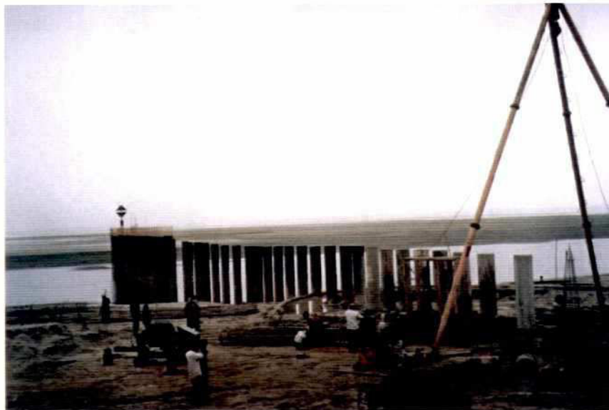
Photo 10.6-1: Adaptation Works at Groyne G-2; Construction of In-Situ Bored Piles
