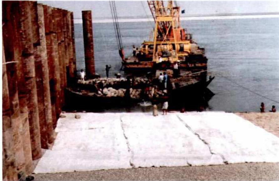
Photo 7.9-3: Groyne G-1, Bed Protection, dumping of Boulders on Geotextile Filter Mat
