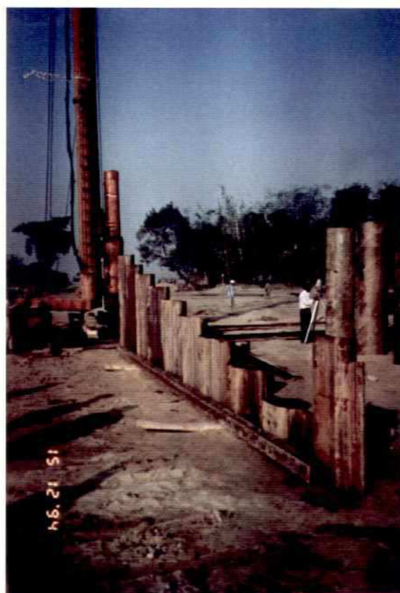
Photo 7.13-2: Steel sheet pile installation at Groyne G-1; Piling with Kobe Diesel Hammer
