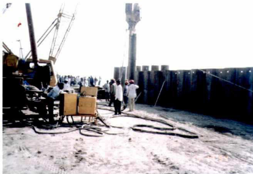
Photo 7.13-1: Steel sheet pile installation at Groyne G-1; Piling with Electric Vibrator
