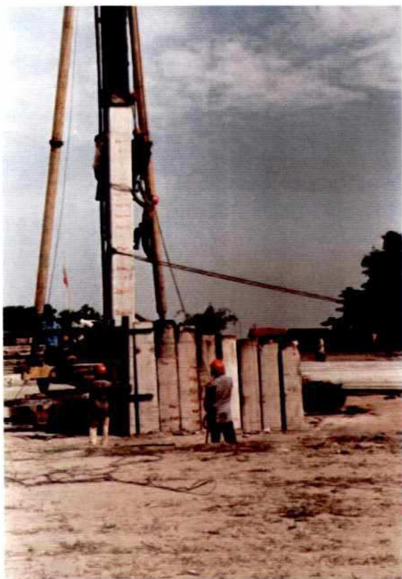
Photo 7.13-3: Concrete Sheet Pile installation; Piling with Diesel Hammer Kobe 22
