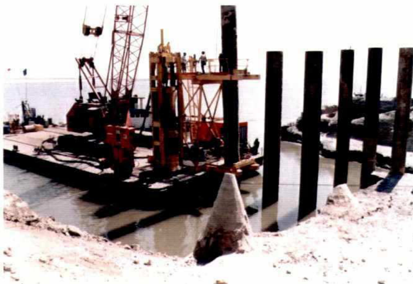
Photo 7.11-9: Pile positioning and fixing into the Pile Guiding Frame
