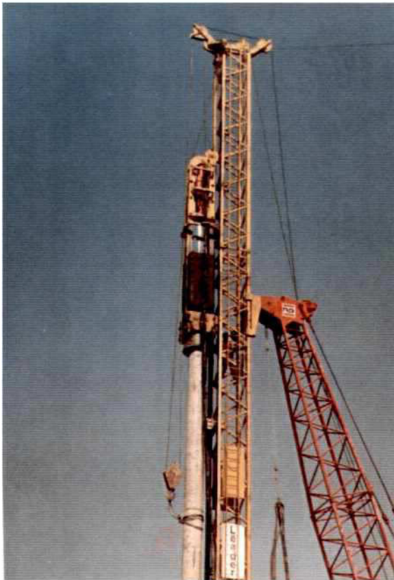
Photo 7.12-3: Piling pre-cast Concrete Spun Piles, Piling Rig, Hydraulic BSP Hammer
