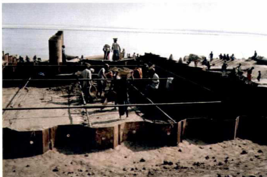
Photo 7.5-6: Backfill of the Cofferdam of Groyne G-1
