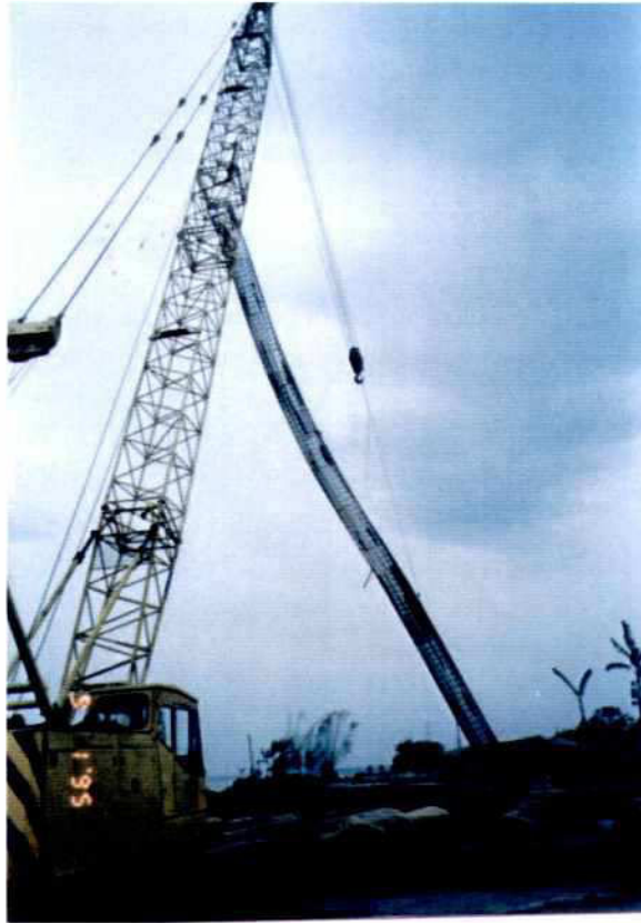
Photo 7.14-2: Lifting of Reinforcement Cage of In-Situ Bored Piles
