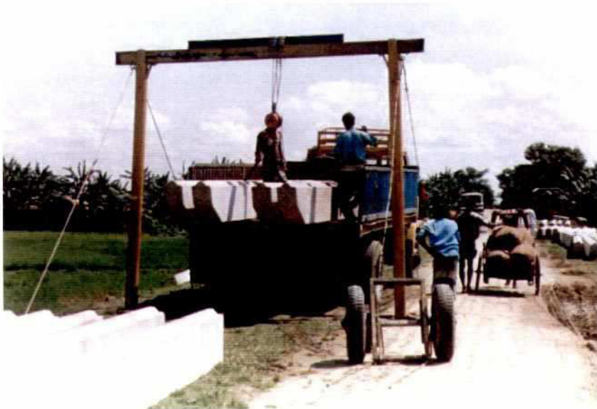
Photo 4.1-1: Pre-cast Reinforced Sheet Piles
