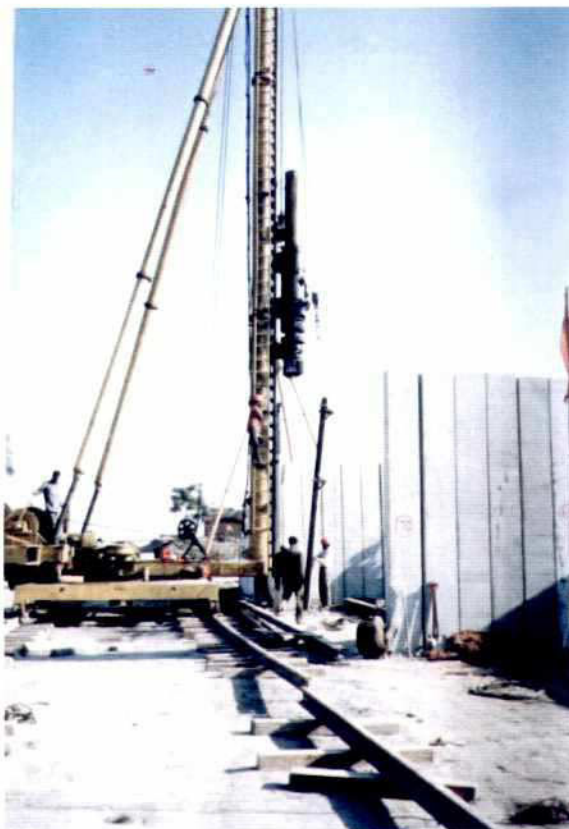
Photo 7.13-4: Concrete Sheet Pile installation; Piling with Diesel Hammer Kobe 22
