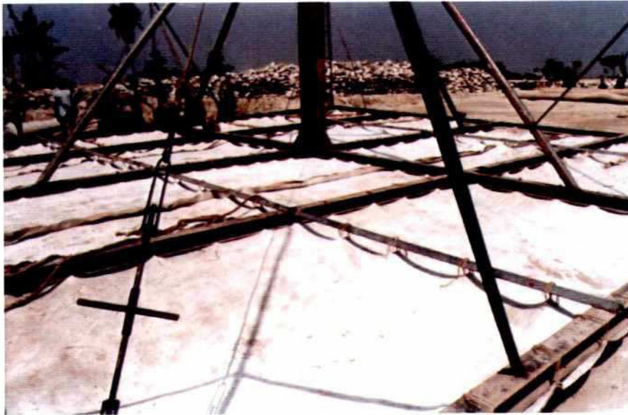
Photo 7.8-1: Geotextile Mat fixed to a Steel Frame
