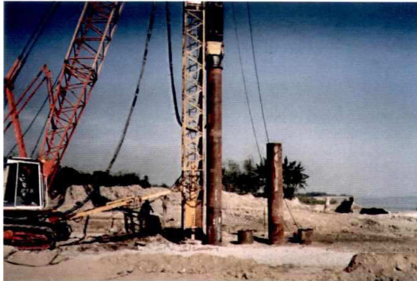
Photo 7.11-3: On-shore Piling of Steel Pile dia 711 mm; Piling rig Kobe 22
