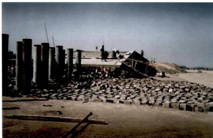
Photo 7.9-9: Groyne G-A, Bed Protection, CC-Blocks
