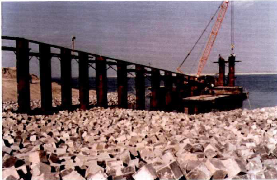
Photo 7.9-7: Groyne G-3, Scour Protection, CC-Blocks
