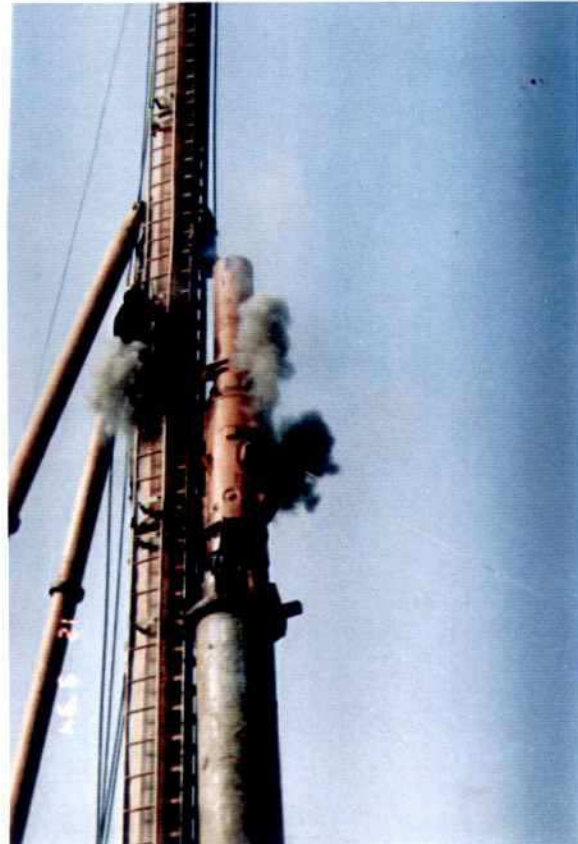
Photo 7.12-2: Piling pre-cast Concrete Spun Piles, Piling Rig, Diesel Pile Hammer Kobe 22
