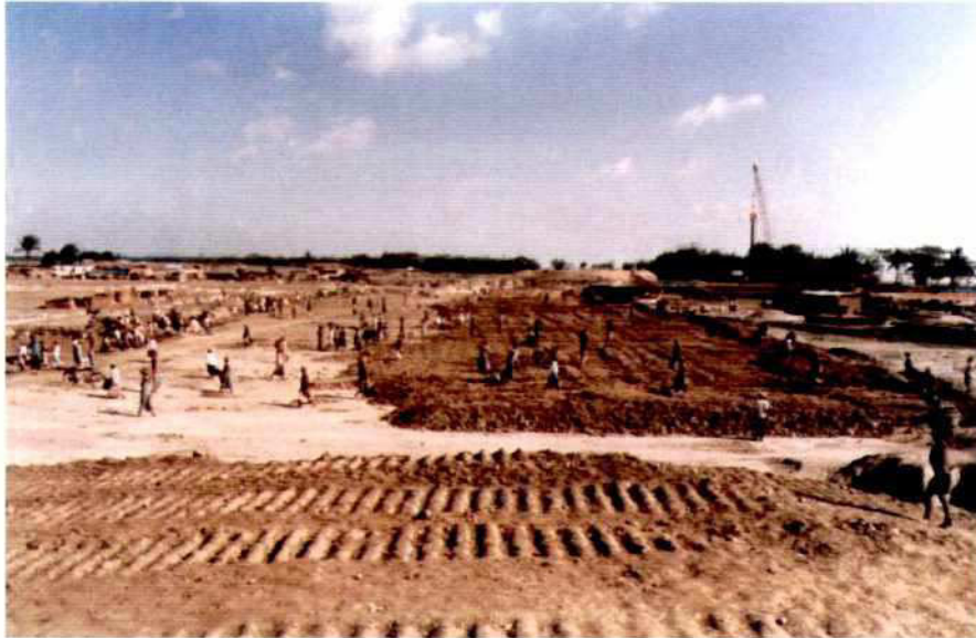
Photo 7.5-1: Earth filling for Main Embankment
