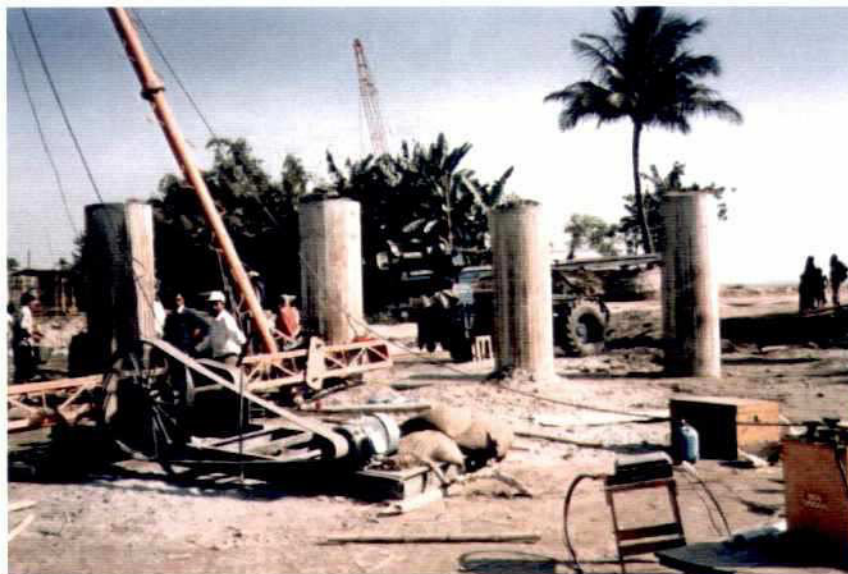
Photo 7.14-4: Ready In-Situ Bored Piles with the permanent Steel Casing
