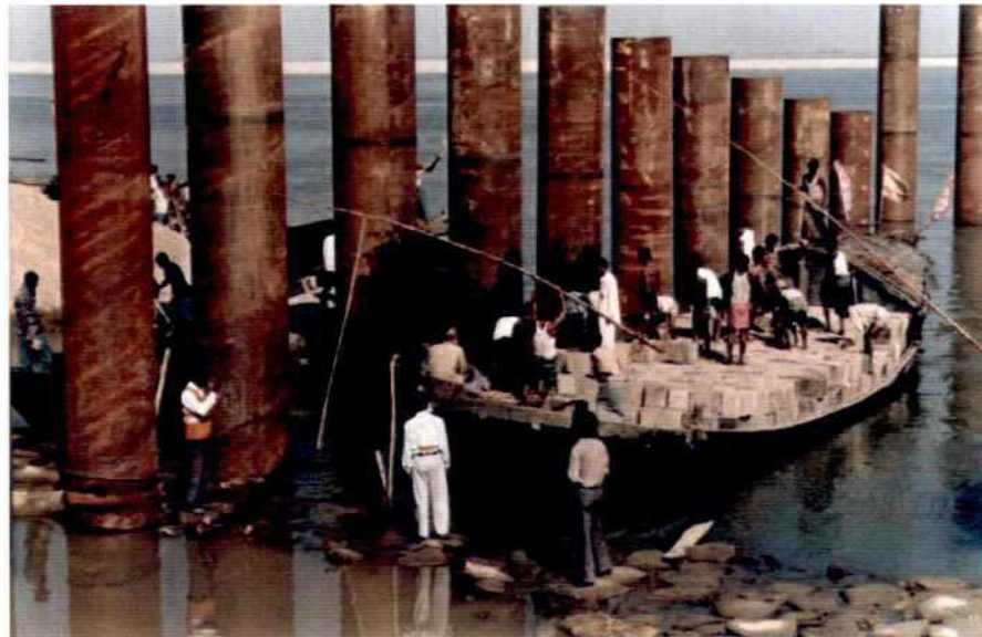
Photo 7.9-2: Dumping of CC-Blocks as Bed Protection from a Country Boat
