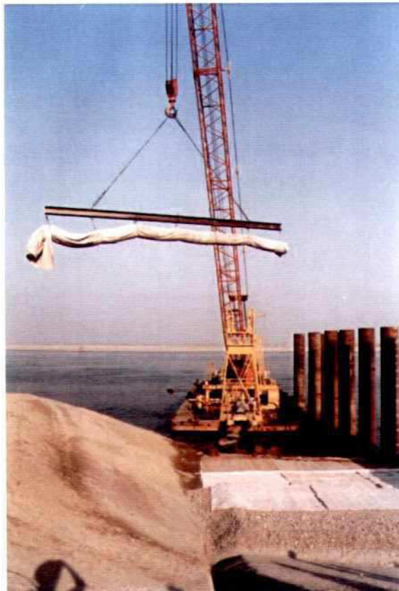
Photo 7.8-2: Geotextile Mat Fixed to a Steel Beam
