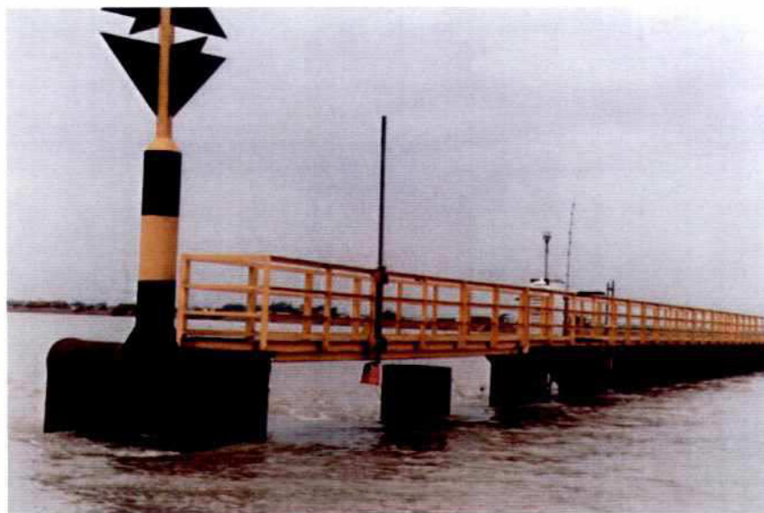
Photo 7.15-2: Steel Gangway of Groyne G-2 with installed Monitoring Equipment
