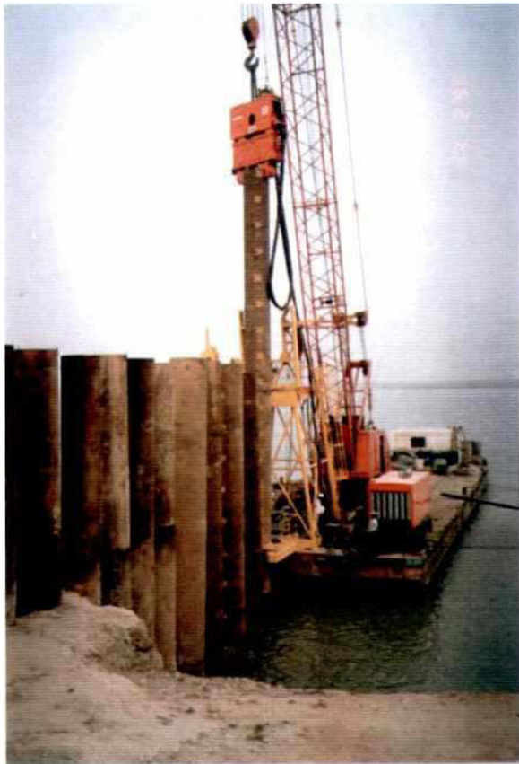
Photo 7.11-10: Piling of Steel Piles dia 1016 mm and 1220 mm by Vibrator PTC 50 H4
