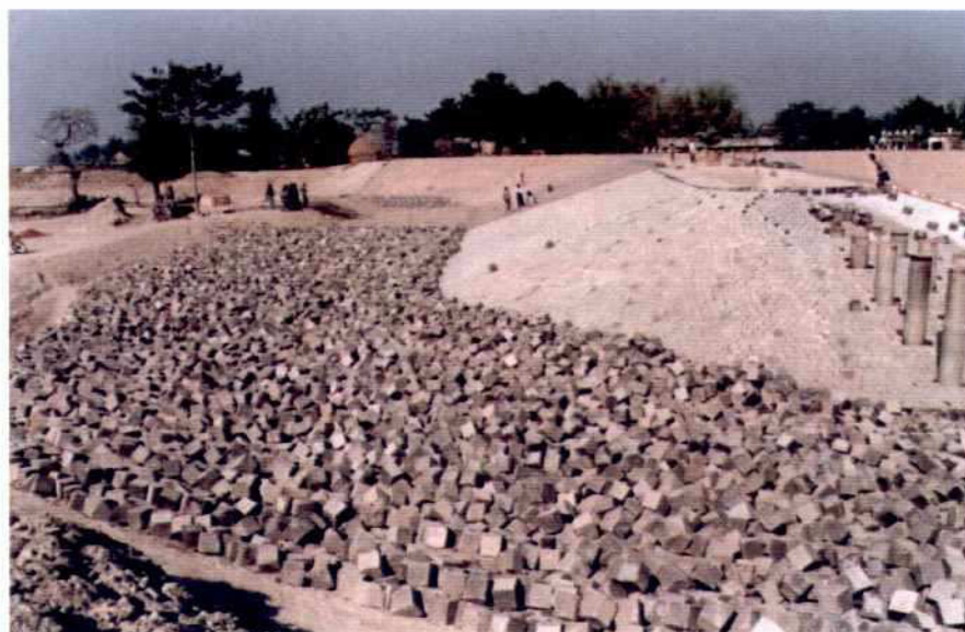
Photo 7.9-10: Groyne G-B/a, Bed Protection, CC-Blocks
