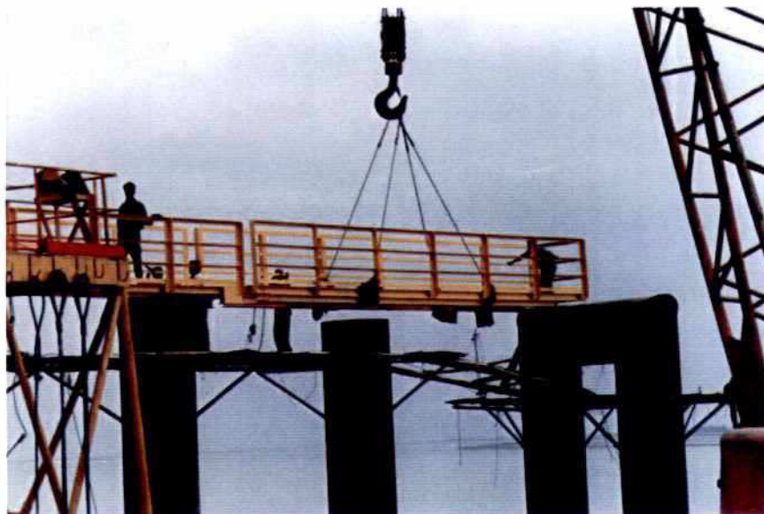
Photo 7.15-1: Installation of Steel Gangway at Groyne G-2
