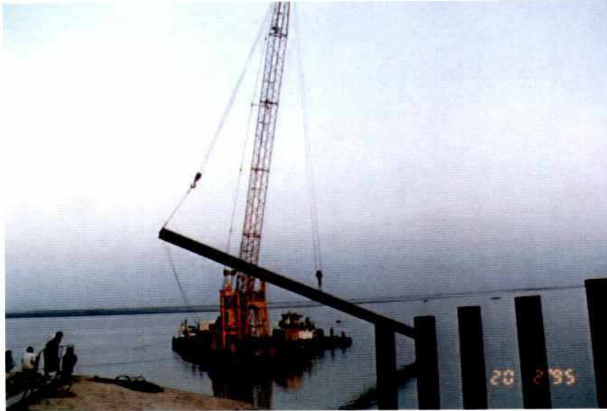
Photo 7.11-6: Pile lifting
