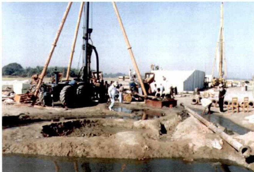
Photo 7.14-1: Drilling of In-Situ Bored Piles, Reverse rotary Method
