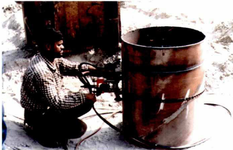
Photo 7.10-5: Pile Gas cutting
