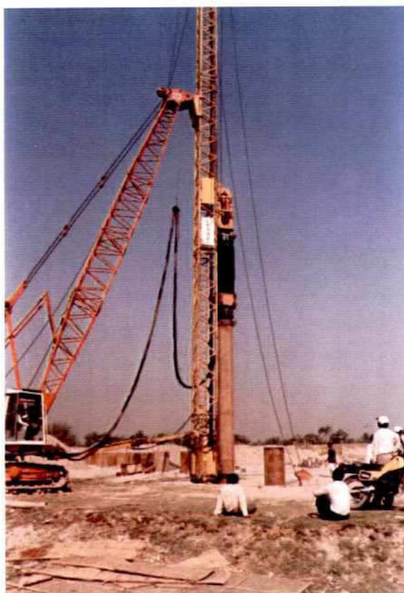
Photo 7.11-2: On-shore Piling of Steel Pile dia 711 mm; Piling rig Kobe 22 Hydraulic BSP Hammer, Leader and R-B 600 SC (Lincoln) Crawler Crane
