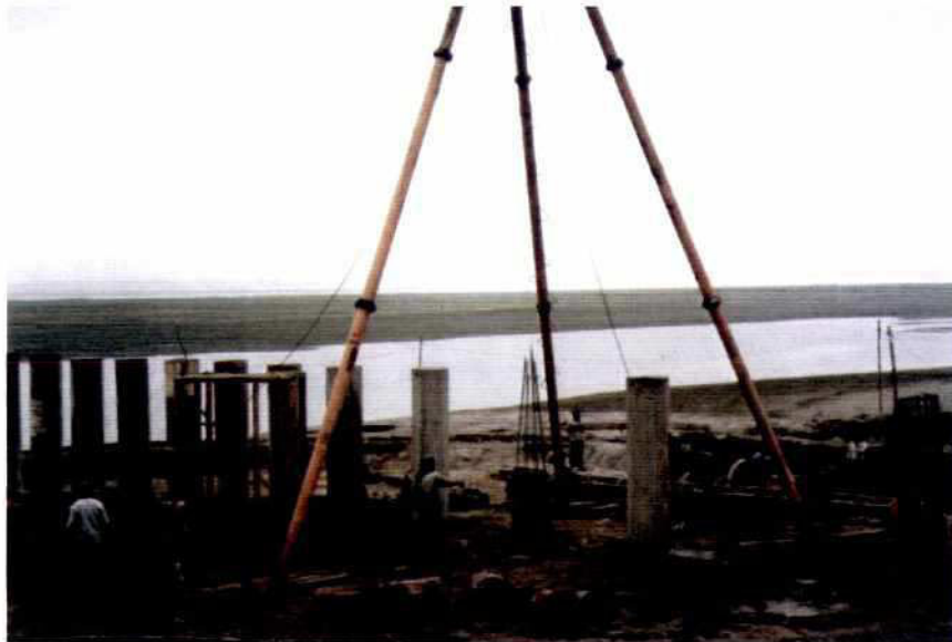
Photo 10.6-2: Adaptation Works at Groyne G-2; Construction of In-Situ Bored Piles
