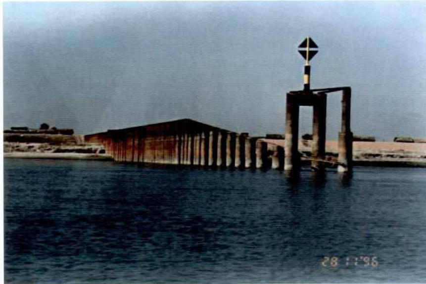
Photo 10.6-3: Adaptation Works at Groyne G-2; Construction of In-Situ Bored Piles
