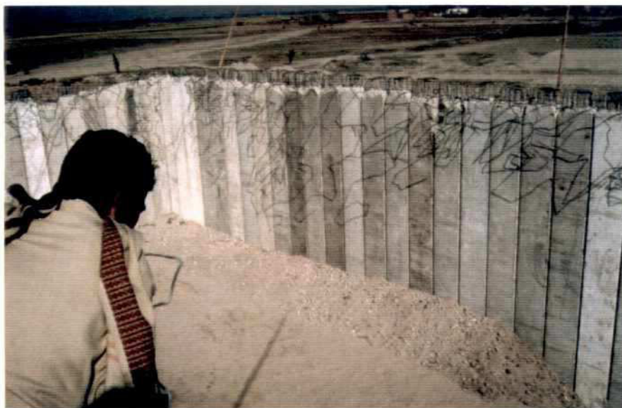
Photo 7.5-5: Backfill of the Cofferdam of Groyne G-A
