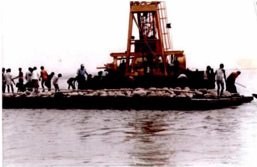
Photo 7.9-1: Dumping of Boulders as Bed Protection from a Flat Barge
