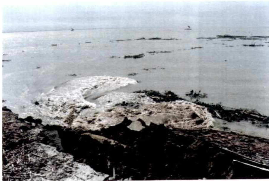
Photo 6.8-3: Erosion process during slide at groyne G-3, August 1995
