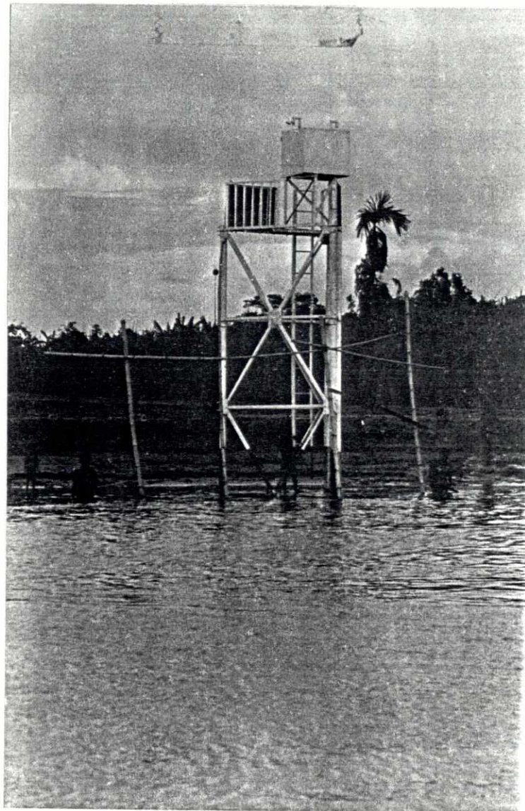
Figure 4.2 : AWLR installation at Bahadurabad, left channel.
