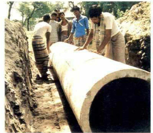
Landless labourers receive training to cast concrete pipes
