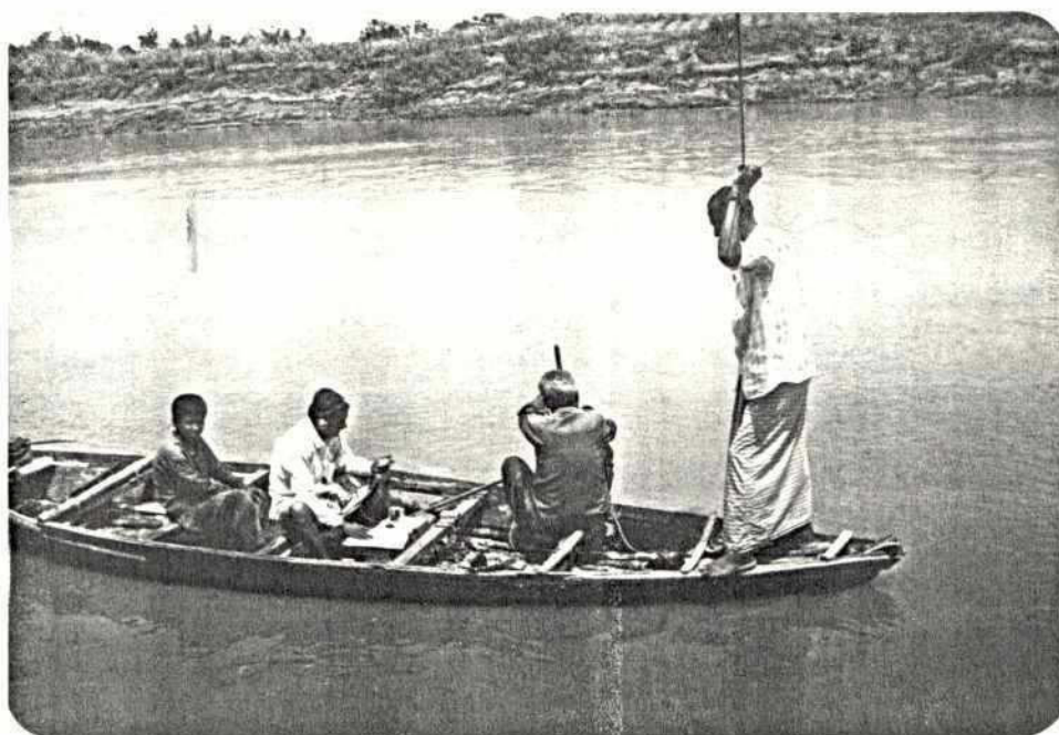
Discharge measurement and dip sample on Khowai River
