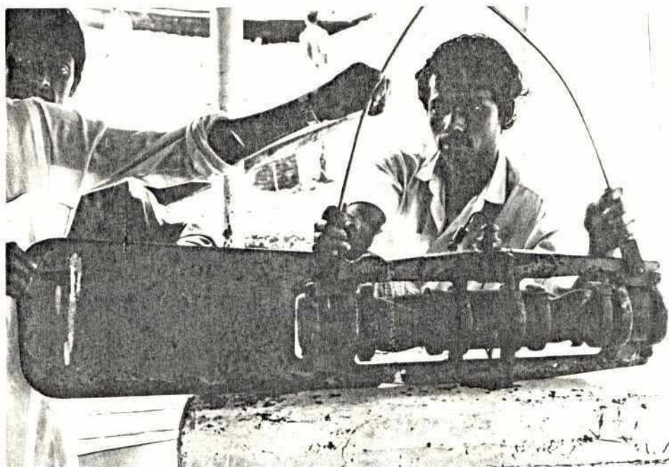
Binkley Sampler used on Meghna River
