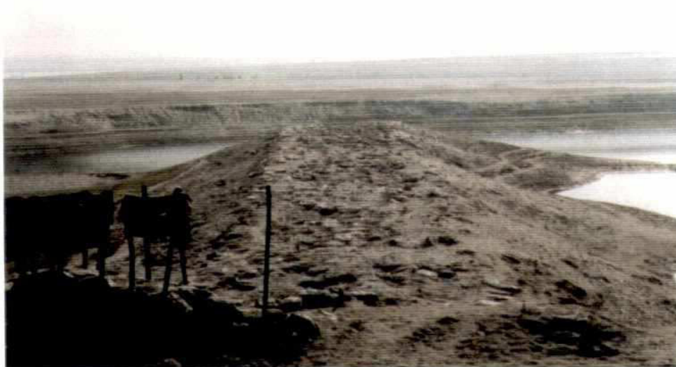
Photo 4.2-10: Earth dam after the flood in January 1998
