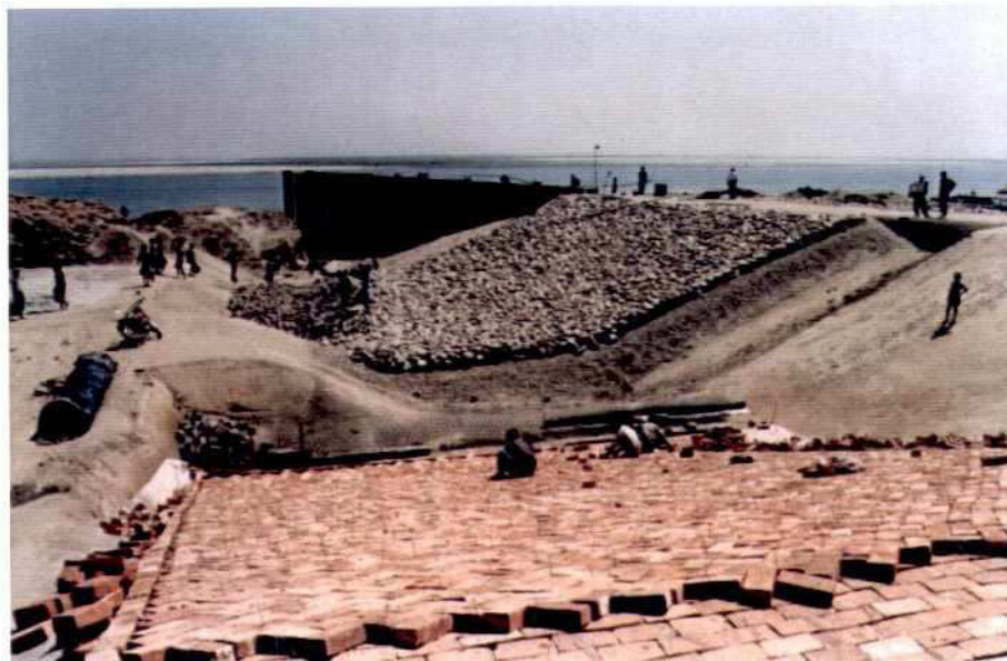
Photo 3.5-4: Installation of rip-rap and brick mattress at groyne G-2
