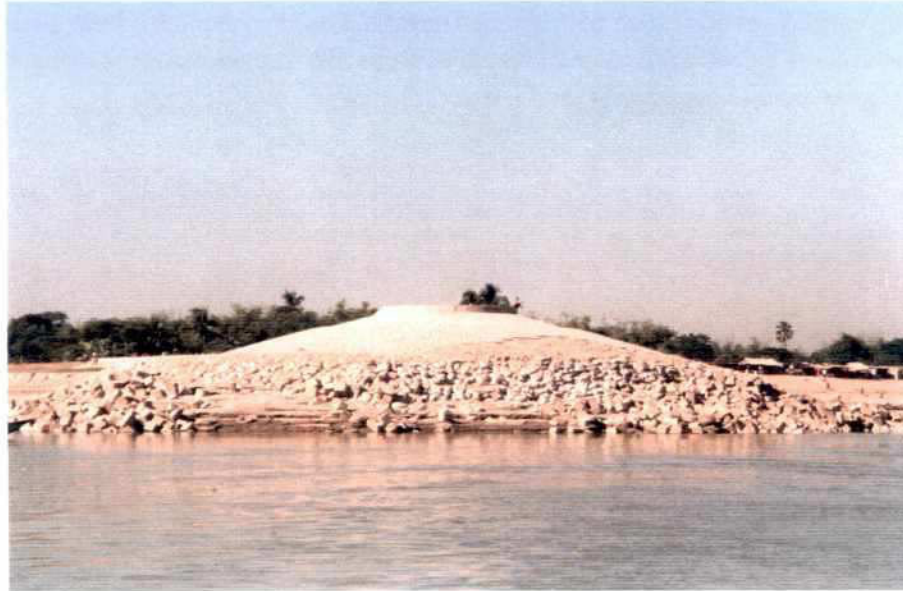
Photo 8.2-4: Head of Kalitola Groyne with dumped concrete blocks and sand bags (situation in December 1999)
