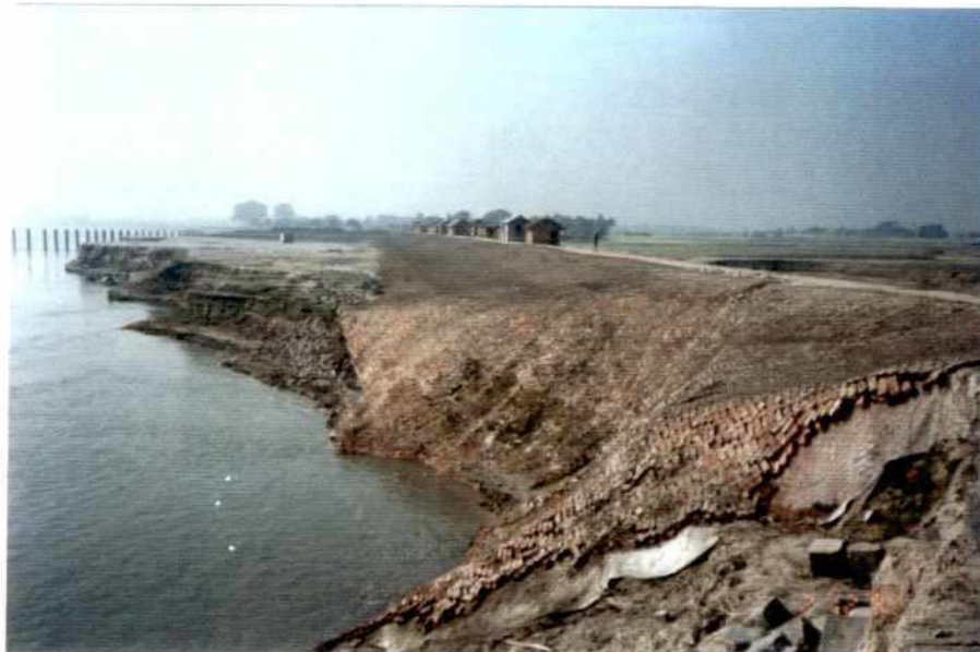
Photo 3.7-4: Main embankment downstream from groyne G-3 after monsoon flood
