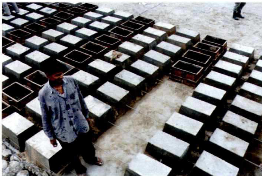
Photo 4.4-4: Casting of articulating CC-blocks, interconnected by steel cables
