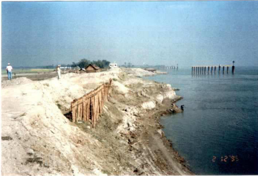
Photo 3.7-1: Remnants of groyne G-2 (view from downstream) and erosion of main embankment d/s of groyne G-2
