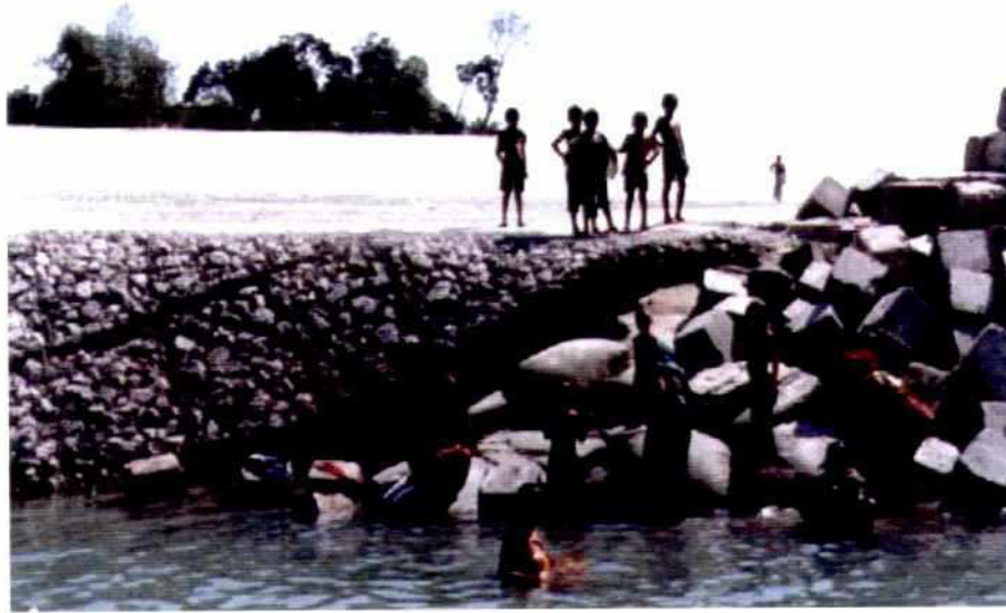
Photo 4.5-1: Partially launched Reno ® -mattresses at section C after monsoon period 1997
