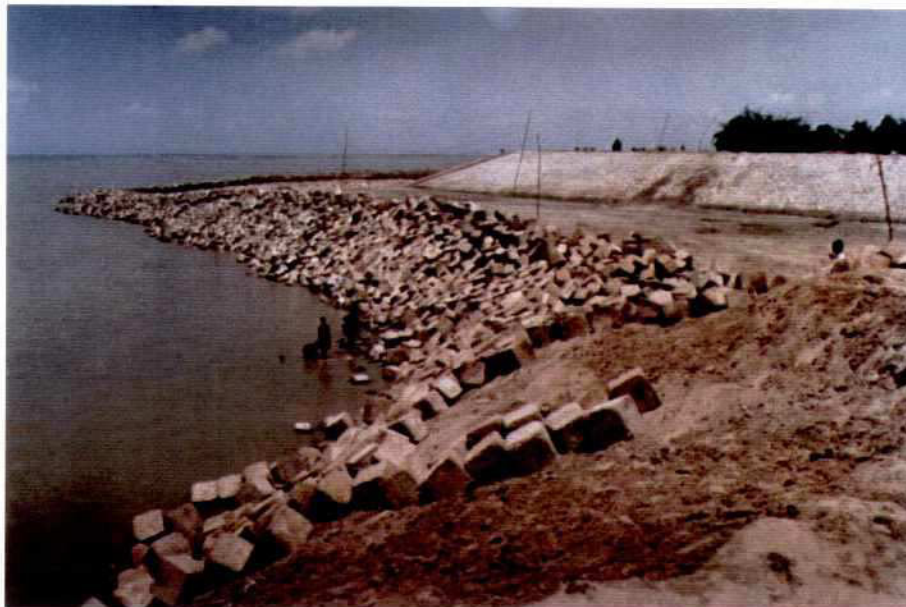
Photo 4.5-2: Exposed sub-layers after severe erosion during monsoon 1997 in front of Section H
