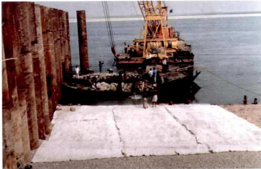
Photo 3.5-3: Groyne G-1, installation of bed protection, dumping of boulders on geo-jute sandwich filter mat
