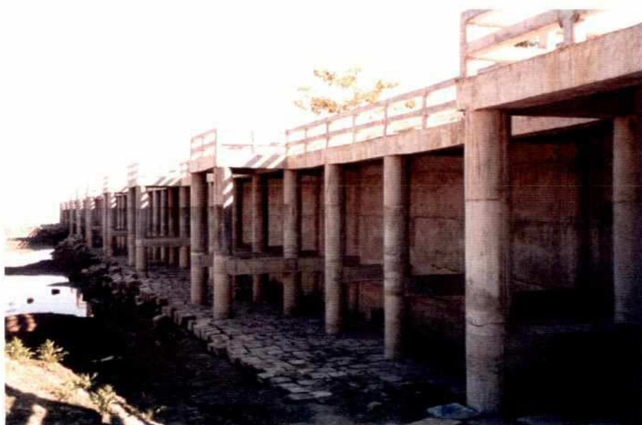
Photo 8.2-6: BWDB-groyne at Singrabari. The protection around the concrete structure has partially displaced (situation in December 1999)
