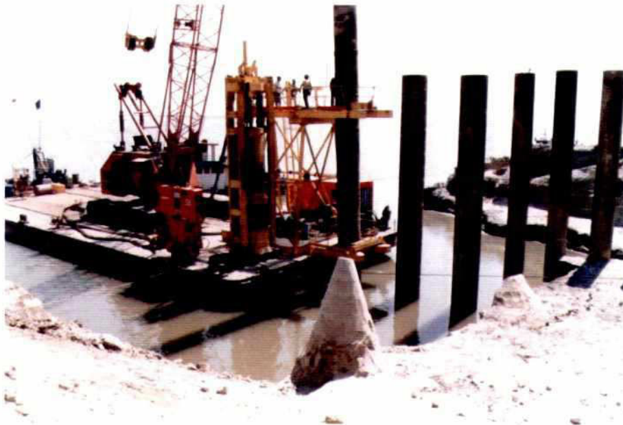
Photo 3.5-5: Off-shore installation of steel pile
