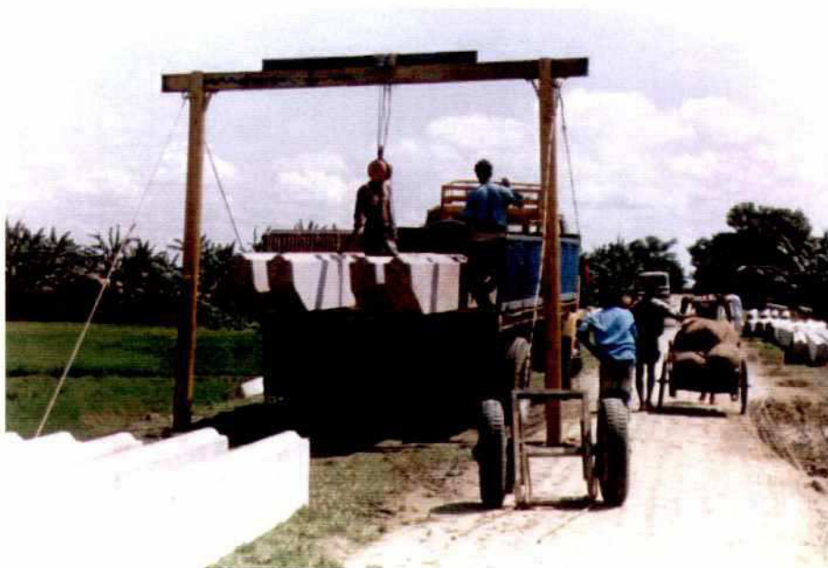
Photo 3.4-3: Pre-cast reinforced sheet piles
