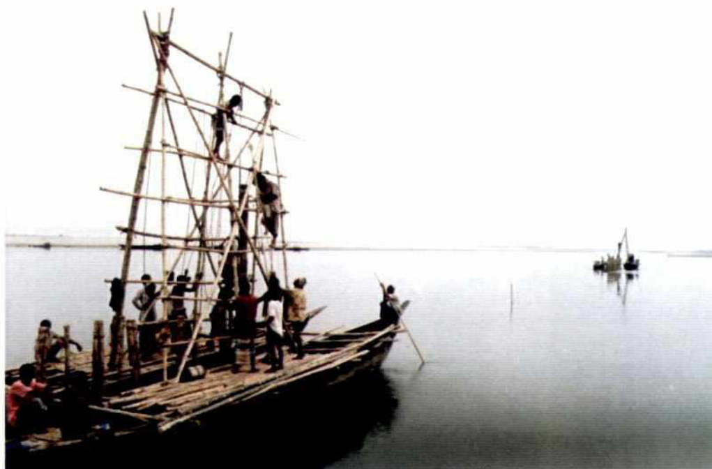
Photo 4.3-1: Pile driving for installation of low water bandals
