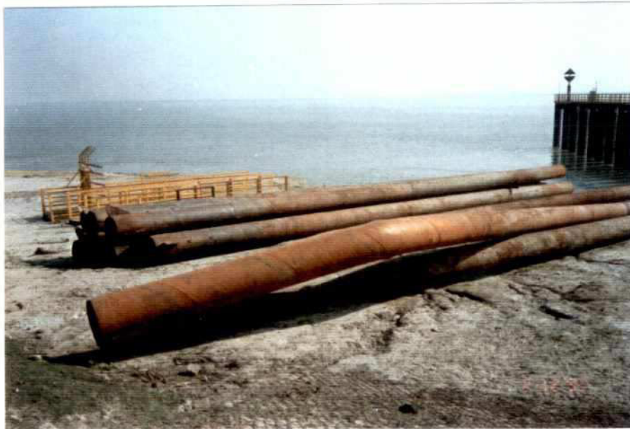
Photo 3.7-2: Recovered tubular steel piles of groyne G-2
