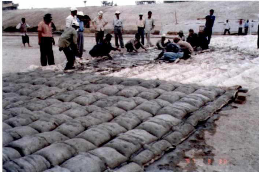
Photo 4.4-5: Filling of the Foreshore ® collapsible mattress with cement grout
