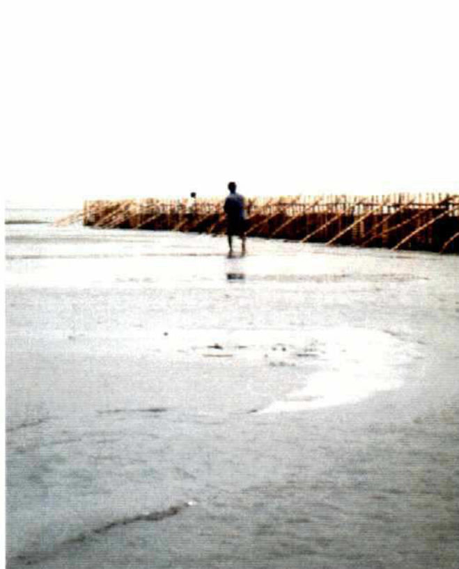
Photo 4.3-4: Sedimentation behind the low water bandals
