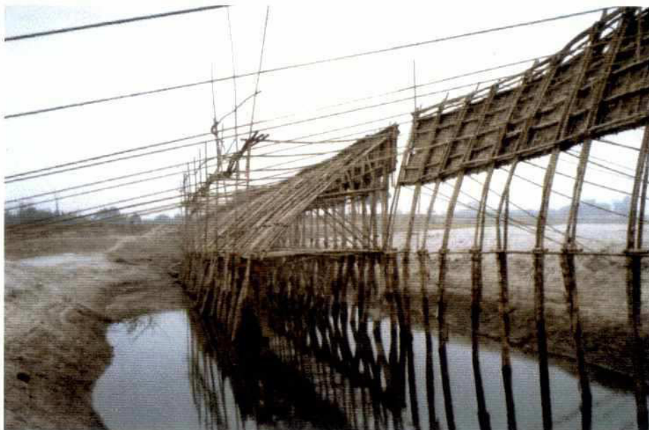
Photo 4.2-8: Scour below the bandal structure Type B and C in January 1998
