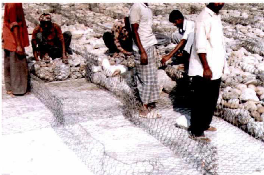
Photo 4.4-3: Reno ® -mattress placed on geo-textile (stone filled cages to be closed by wire mesh)
