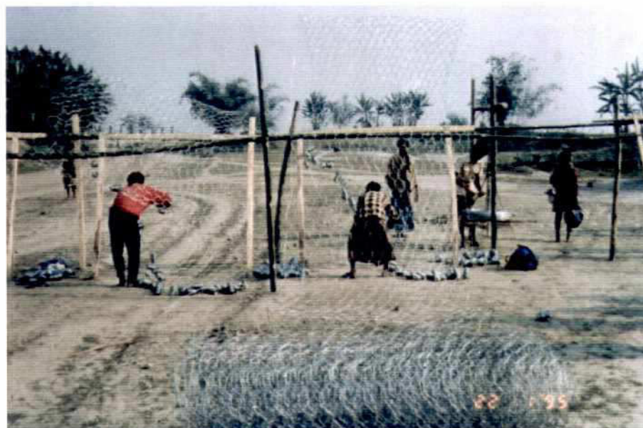
Photo 3.4-1: Production of wiremesh at site
