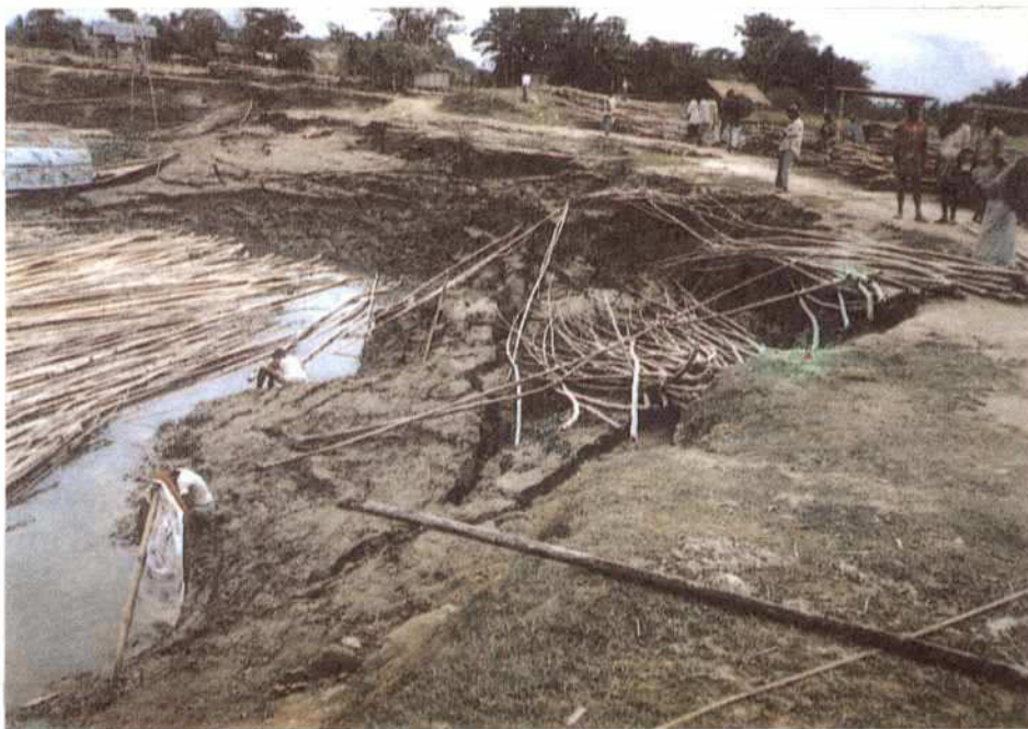
PHOTO 6 : Slump failures in left bank near Markuli.
