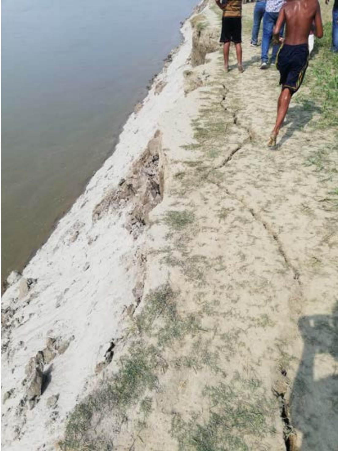
Figure A-8 Crack near the bank
