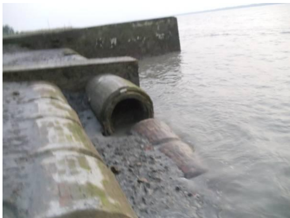
Figure 4.4: Damaged Sluice
