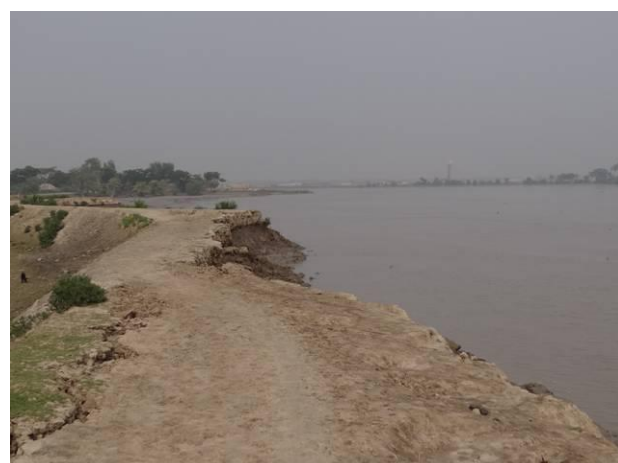
Figure 16: Embankment erosion the Dhaki River
