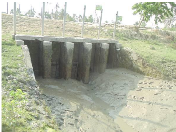
Figure 4.2: 5 vent Drainage Regulator
