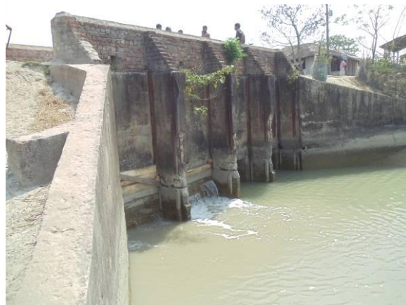
Figure 4.5: Sluice 4 vent regulator
