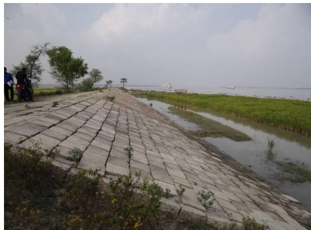
Figure 8: Slope protection at Chunkuri Village
