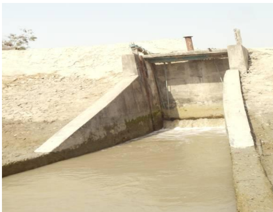
Figure 4.4: Sluice 1 vent regulator
