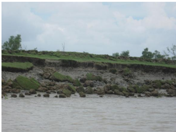
Figure 6.10: Erosion at right bank of the Passur River (Chunkuri village)
