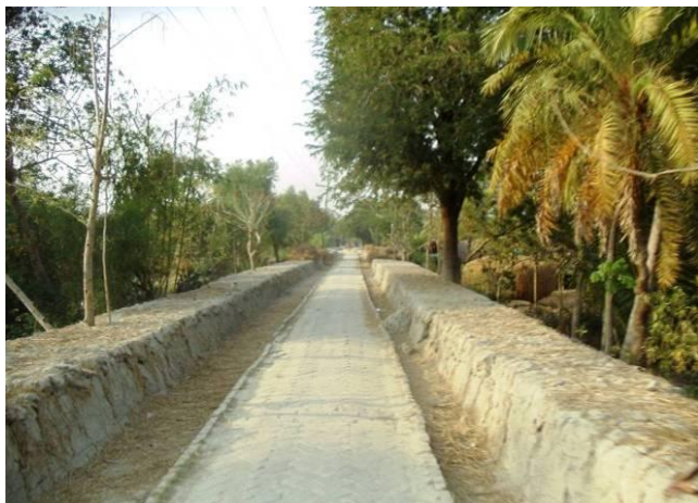
Figure 19: Internal Herringbone road in the Polder
