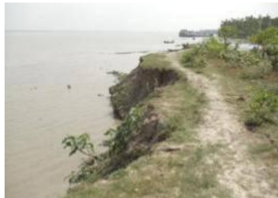
Figure 0.5: Erosion-affected Embankment at Tafalbaria
