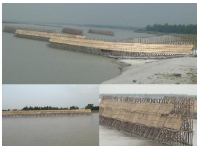
Figure 3.19: Sketch of Permanent-Type Top Blocked Permeable Groyne
