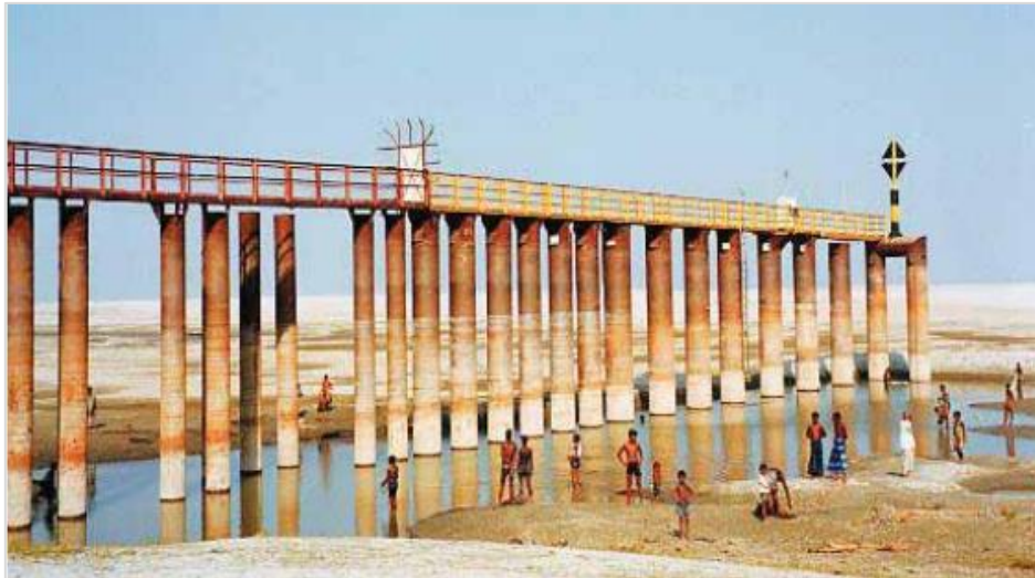
Figure 4.6: Permeable Groyne at Kamarjani of Jamuna River
